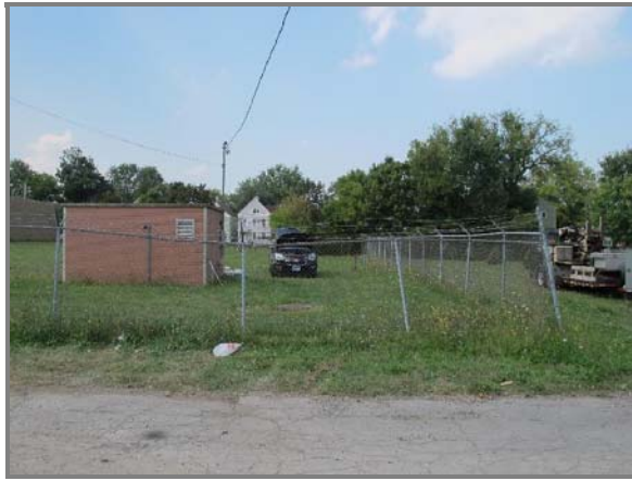
Bent-over fence poles and a separated top pipe.
