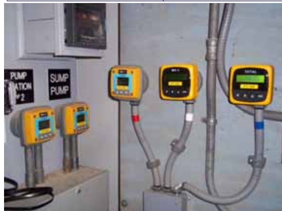
Photo 5: Flow Transmitters
