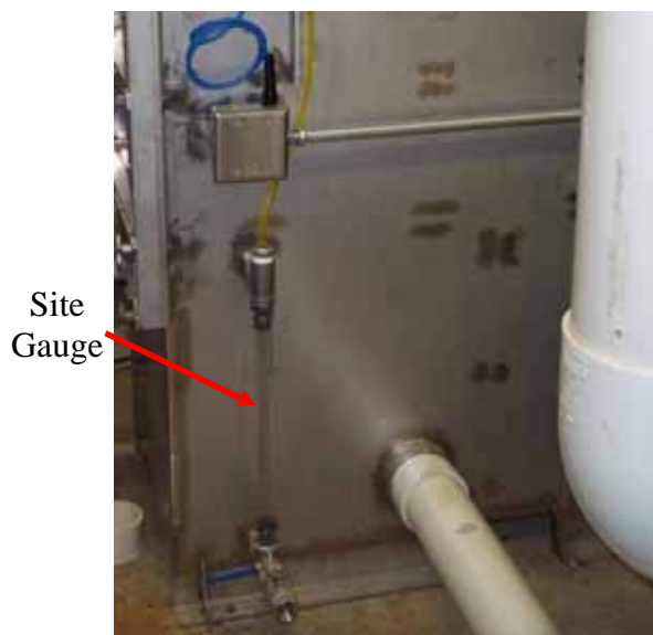
Photo 2: Air Stripper Site Gauge
