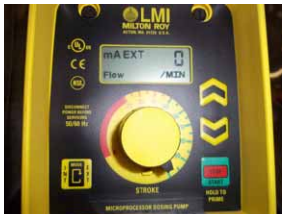
Photo 1: Chemical Metering Pump Controls
