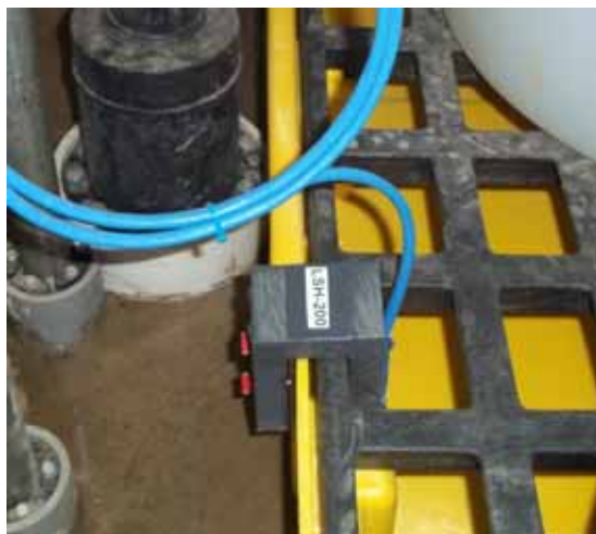
Photo 7: Wet Pallet Sensor
