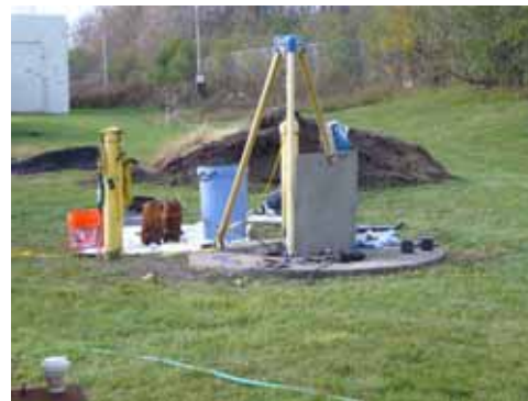
Photo 2: Tripod Set Up For Confined Space Entry
