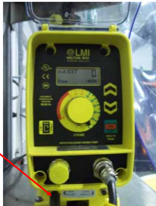
Photo 6: Chemical Metering Pump
