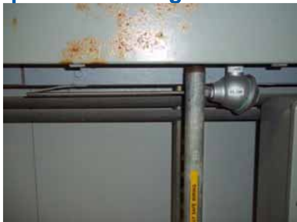
Photo 9: Building Temperature Transmitter
