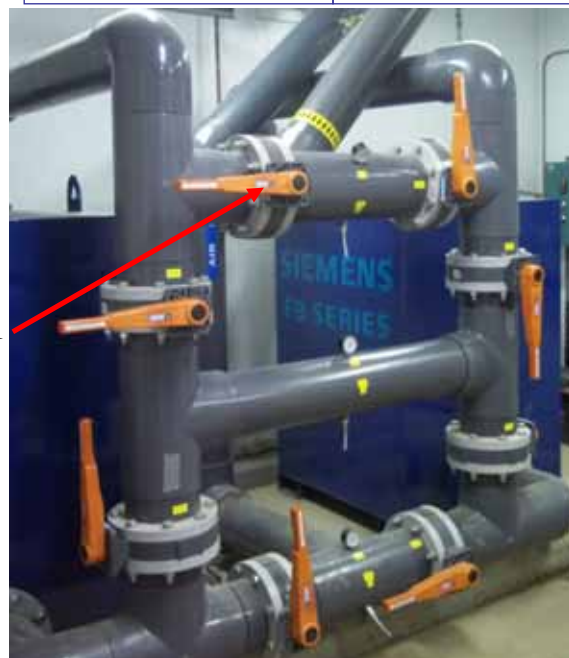
Photo 4: VPGAC Manifold
