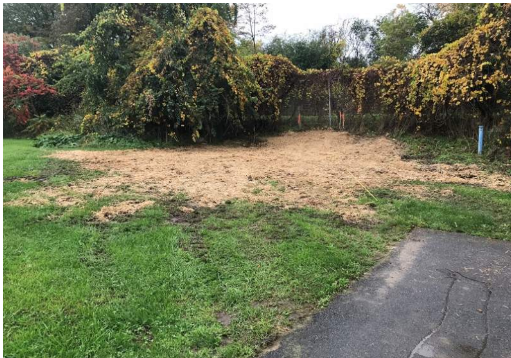
Date: 10/11/2018 Site Name: Former Lockheed Martin Corporation French Road Facility Photographer's Initials: AG Description: Photograph #21 from the southern portion of Excavation Area LMCU-SS-20 facing north showing seed and straw spread at this location.
