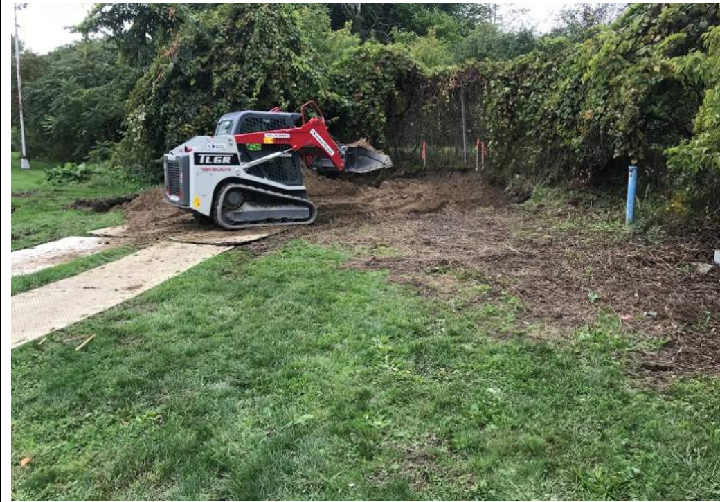
Date: 09/28/2018 Site Name: Former Lockheed Martin Corporation French Road Facility Photographer's Initials: AG Description: Photograph #12 from the eastern portion of Excavation Area LMCU-SS-21 facing west showing placement of backfill in this area.
