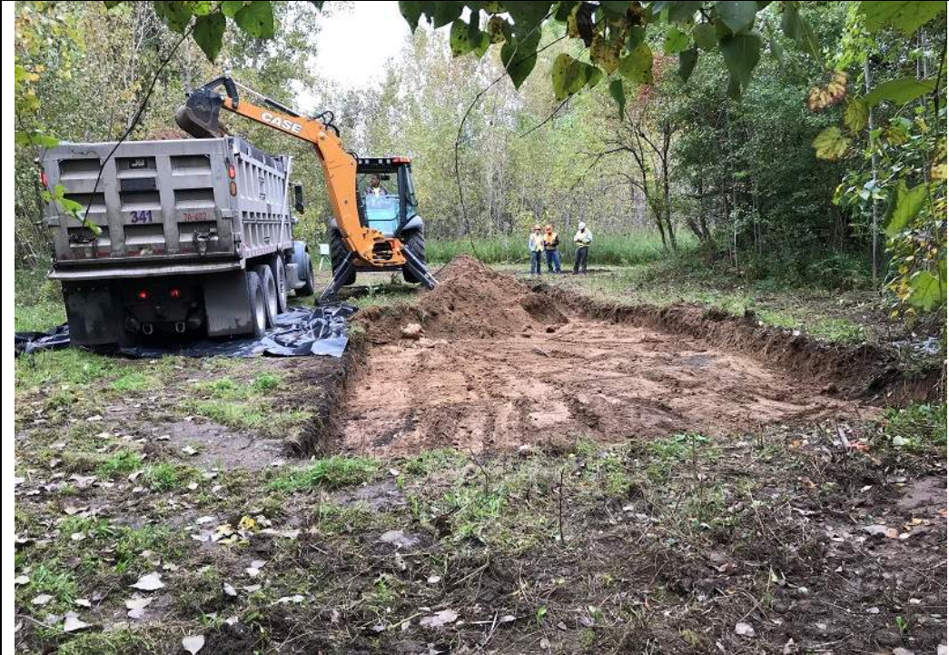
Date: 10/01/2018 Site Name: Former Lockheed Martin Corporation French Road Facility Photographer's Initials: AG Description: Photograph #16 from the southern portion of Excavation Area LMCU-SS-07 facing north showing soil removed to target depth in the southern portion of this area.
