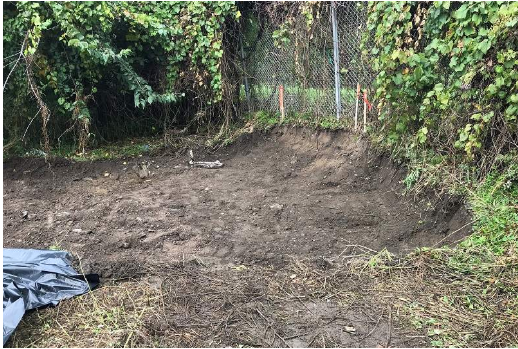
Date: 09/28/2018 Site Name: Former Lockheed Martin Corporation French Road Facility Photographer's Initials: AG Description: Photograph 10 from the eastern portion of Excavation Area LMCU-SS-21 facing west showing soil removed to target depth from the northern portion of this area.
