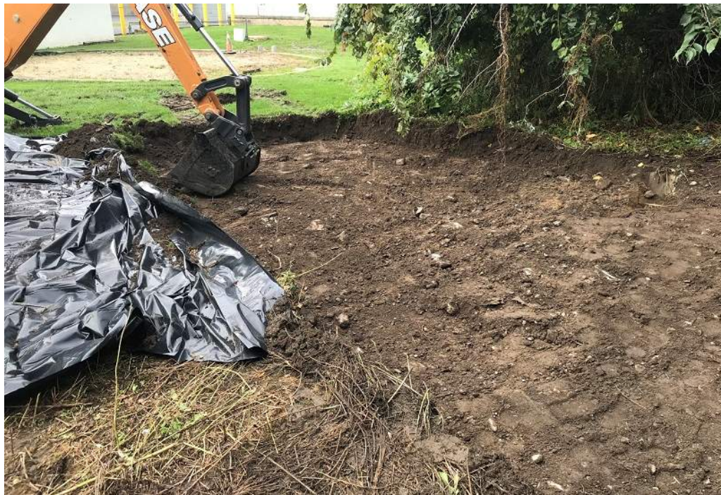
Date: 09/28/2018 Site Name: Former Lockheed Martin Corporation French Road Facility Photographer's Initials: AG Description: Photograph #11 from the eastern portion of Excavation Area LMCU-SS-21 facing south showing soil removed to target depth from the northern portion of this area.
