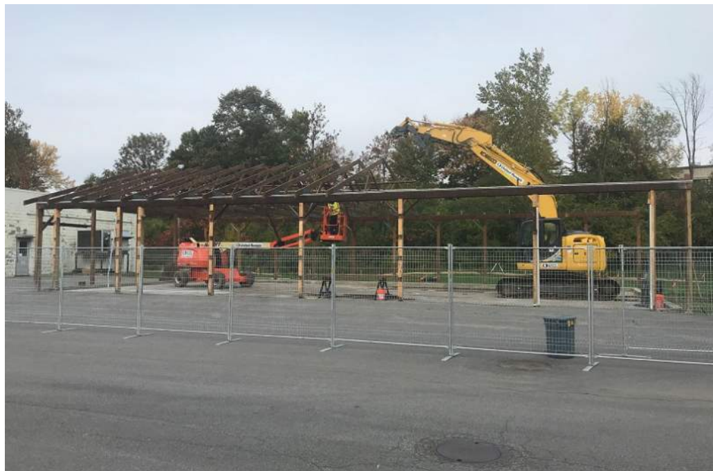
Date: 10/08/2018 Site Name: Former Lockheed Martin Corporation French Road Facility Photographer's Initials: AG Description: Photograph #7 from the southern side of the pole barn building facing north showing removal of pole barn roof trusses.
