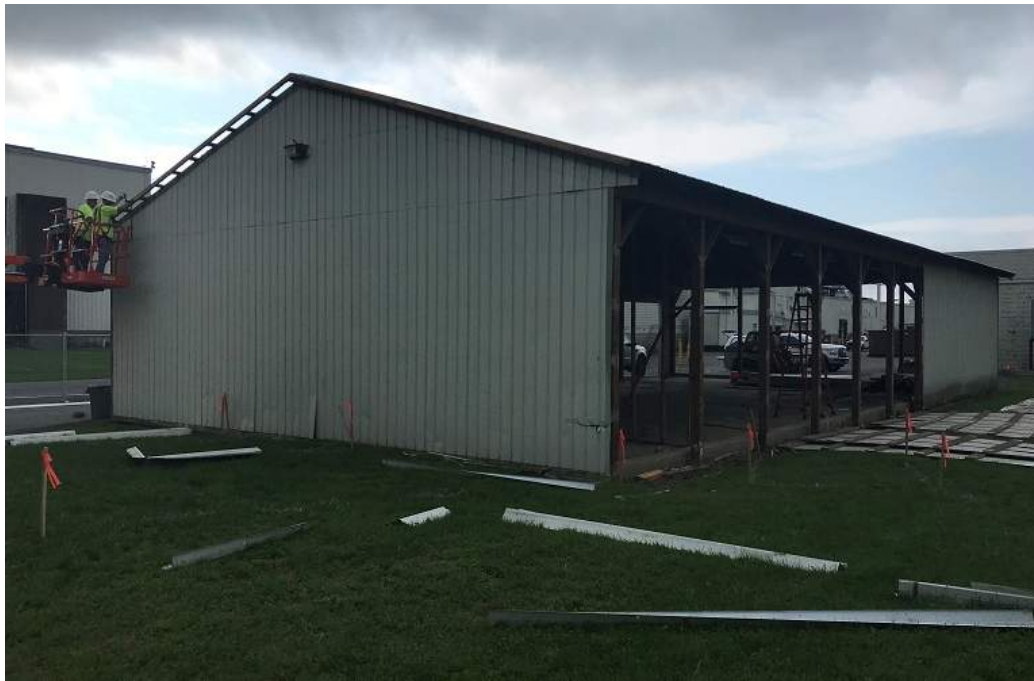
Date: 09/21/2018 Site Name: Former Lockheed Martin Corporation French Road Facility Photographer's Initials: AG Description: Photograph #4 from the northeast corner of the pole barn building showing siding removed from the northern side of the building.
