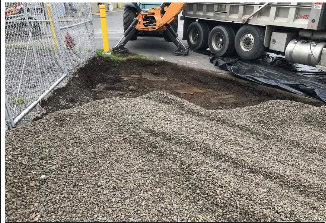
Date: 09/28/2018 Site Name: Former Lockheed Martin Corporation French Road Facility Photographer's Initials: AG Description: Photograph #14 from the central portion of Excavation Area LMCU-SS-20 facing east showing crushed stone backfill placed in the western and central portions of this area (foreground) and soil removed to target depth in the eastern portion of this area (background).
