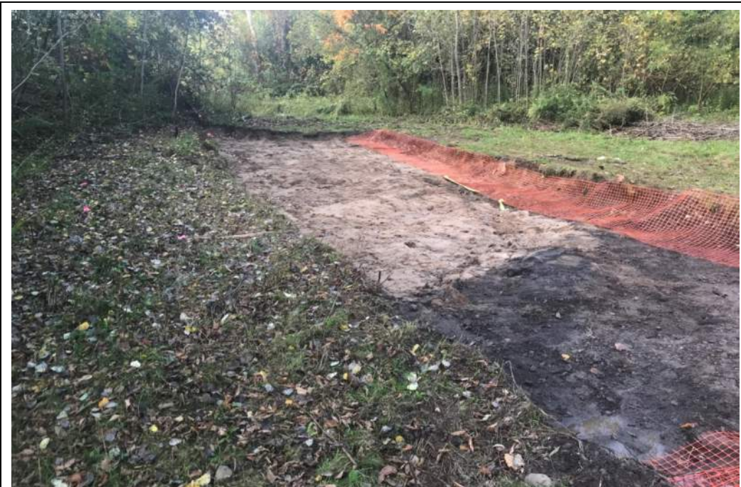
Date: 10/10/2018 Site Name: Former Lockheed Martin Corporation French Road Facility Photographer's Initials: AG Description: Photograph #17 from the northeastern portion of Excavation Area LMCU-SS-07 facing south showing soil removed from the southern portion of this area to target depth. Photograph also shows orange snow fence placed on the western sidewall of this area.
