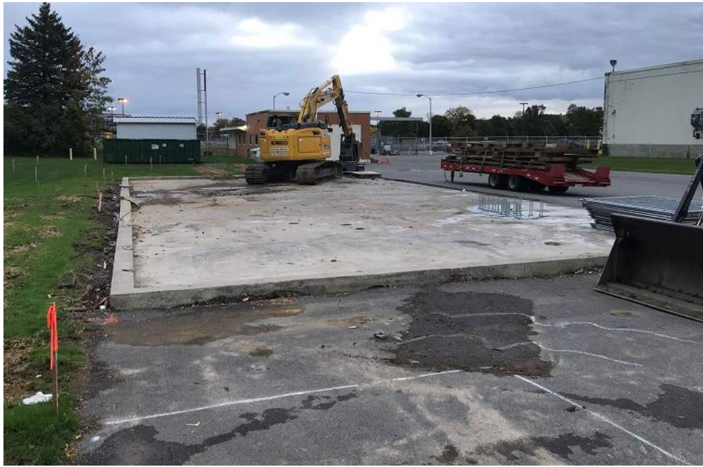
Date: 10/12/2019 Site Name: Former Lockheed Martin Corporation French Road Facility Photographer's Initials: AG Description: Photograph #8 from the western side of the former pole barn foundation facing east showing the building superstructure removed and the foundation left in-place.
