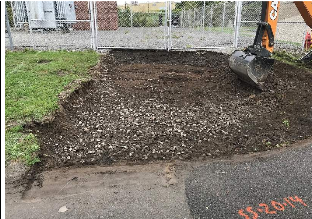
Date: 09/28/2018 Site Name: Former Lockheed Martin Corporation French Road Facility Photographer's Initials: AG Description: Photograph #13 from the southern portion of Excavation Area LMCU-SS-20 facing north showing soil removed to target depth in the western portion of this area.
