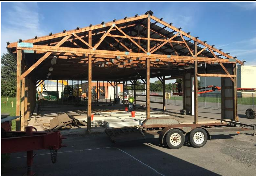
Date: 09/24/2018 Site Name: Former Lockheed Martin Corporation French Road Facility Photographer's Initials: AG Description: Photograph #5 from the western side of the pole barn building showing removal of siding from the building.
