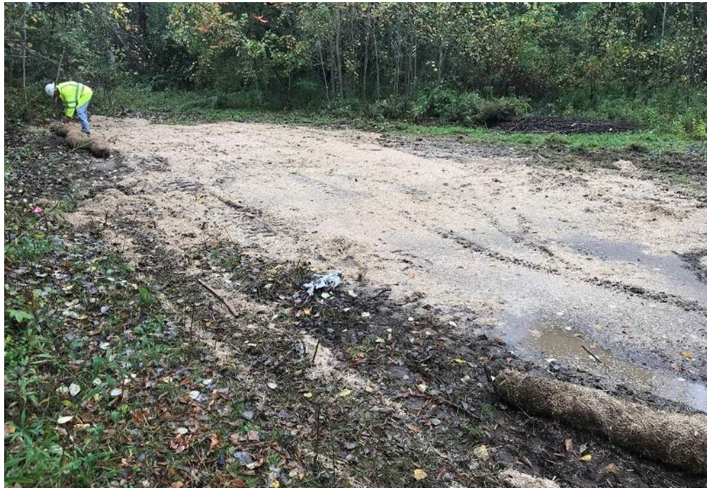
Date: 10/11/2018 Site Name: Former Lockheed Martin Corporation French Road Facility Photographer's Initials: AG Description: Photograph #20 from the northeastern portion of Excavation Area LMCU-SS-07 facing south showing seed and straw being spread at this location.
