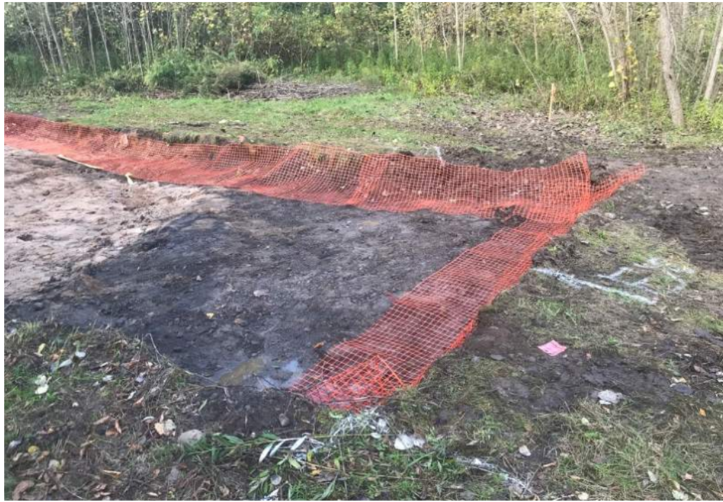
Date: 10/10/2018 Site Name: Former Lockheed Martin Corporation French Road Facility Photographer's Initials: AG Description: Photograph #18 from the northeastern portion of Excavation Area LMCU-SS-07 facing west showing soil removed from the northern portion of this area to target depth. Photograph also shows orange snow fence placed on the northern and western sidewalls of this area.
