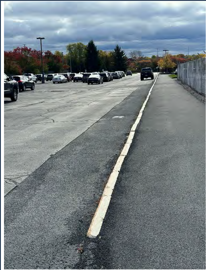
Photograph No.: 023 Comments: East side – showing parking/pavement area – looking South.
