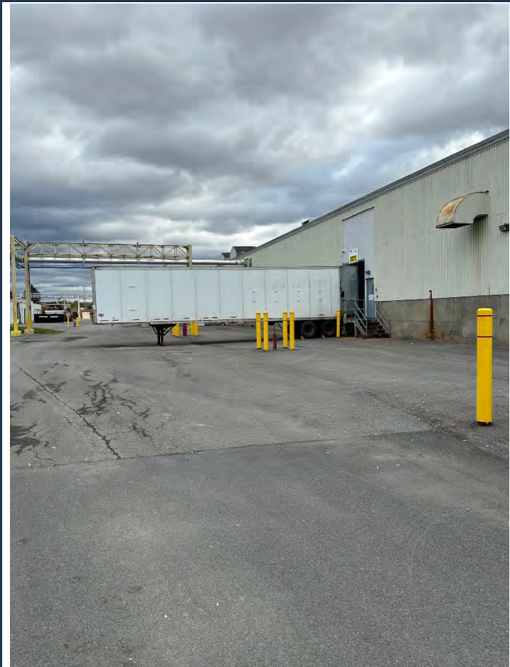
Photograph No.: 011 Comments: North side, West end of building – looking East.
