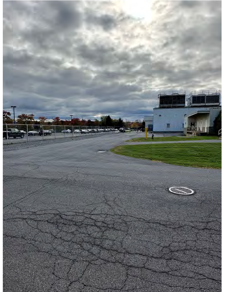
Photograph No.: 020 Comments: East side, along security fence line – looking South.
