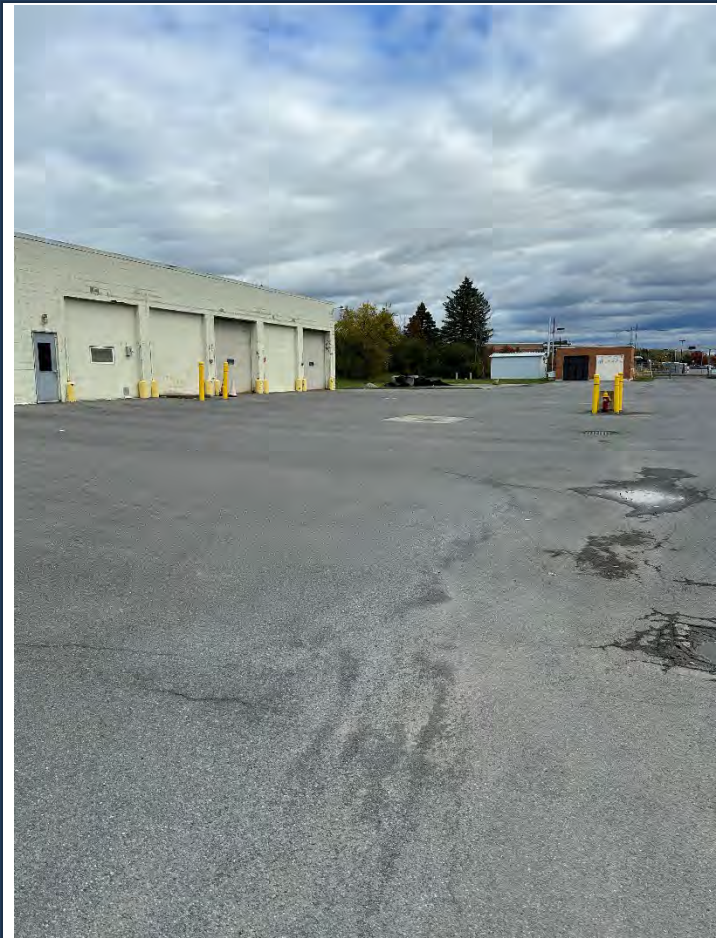
Photograph No.: 017 Comments: North side – loading dock area – looking Northeast.
