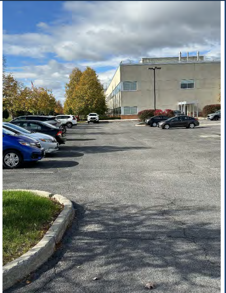
Photograph No.: 026 Comments: East side – showing parking/pavement area and main building – looking West.
