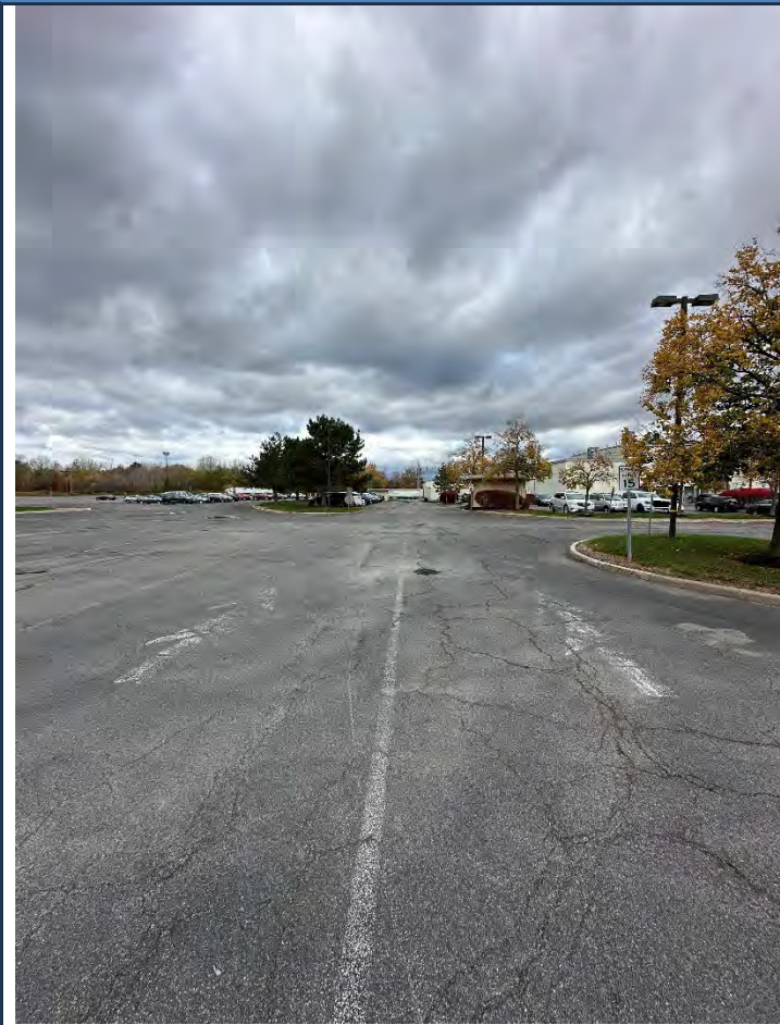
Photograph No.: 005 Comments: West side, typical parking pavement – looking North.
