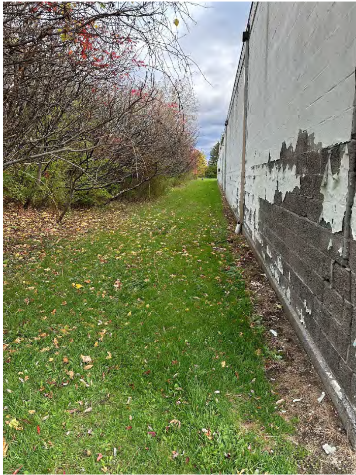
Photograph No.: 015 Comments: Northside area, North of maintenance building – looking East.
