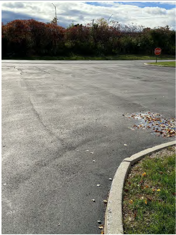
Photograph No.: 027 Comments: East side – showing parking/pavement area – looking South.
