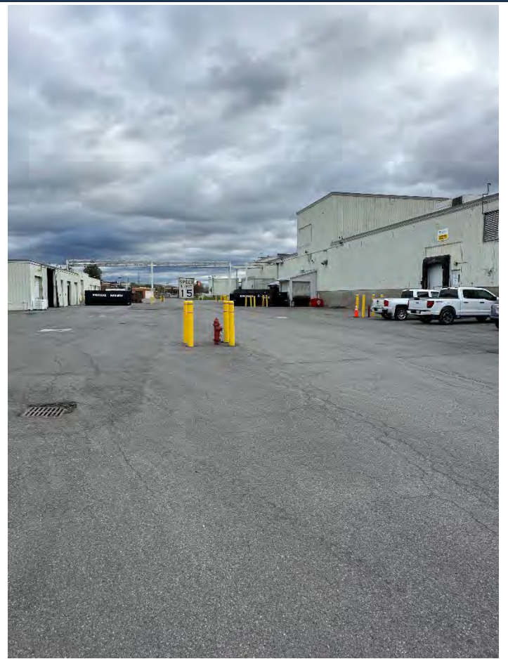
Photograph No.: 014 Comments: North side - Central area main building - looking East.
