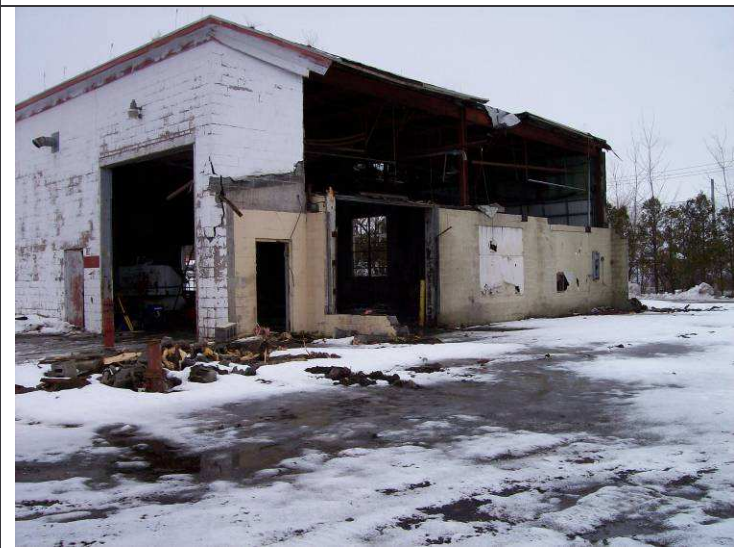
View of Warehouse Portion and slab after demolition (facing west).
