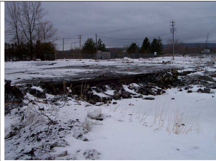
View of slab and loading dock area with treatment system shed in background (facing northeast).
