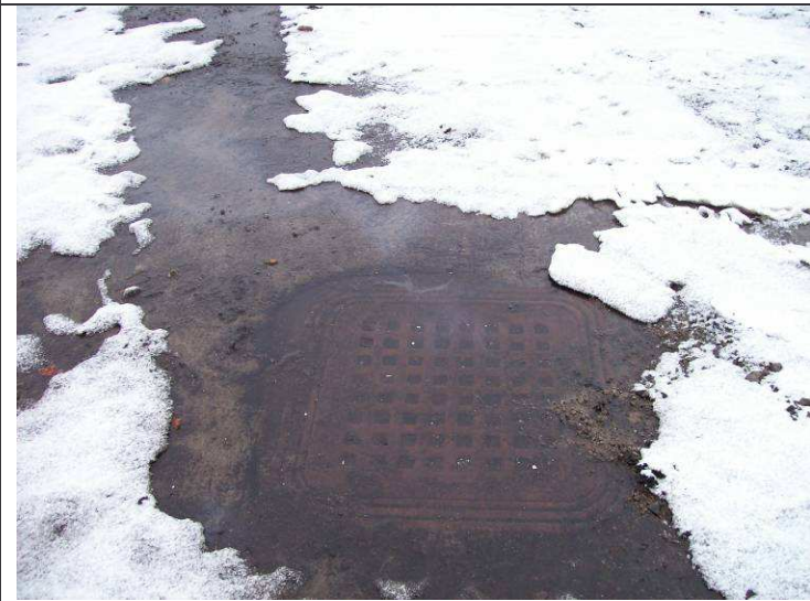
Drain observed in slab.
