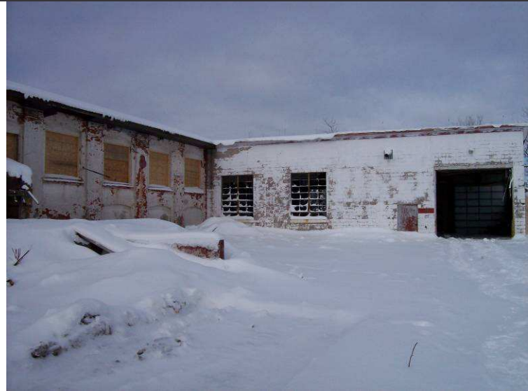
Looking west at Courtyard Area, with the Main Building to the left and the Warehouse portion to the right.
