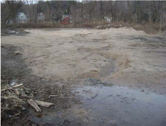
1/10/08 View of settlement within backfilled IRM excavation
