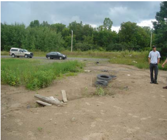
8/13/08 View of settlement areas filled with debris within backfilled IRM excavation
