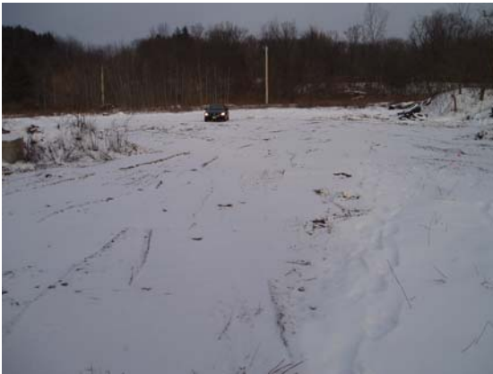
12/10/07 View of backfilled IRM excavation looking east
