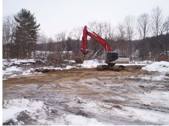
12/6/07 View of backfill activities looking southwest
