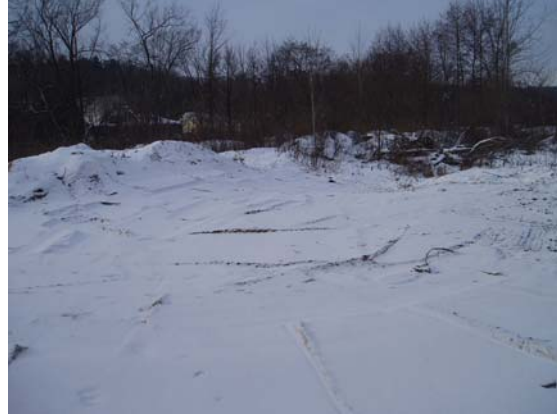
12/10/07 view of backfilled IRM excavation looking northwest
