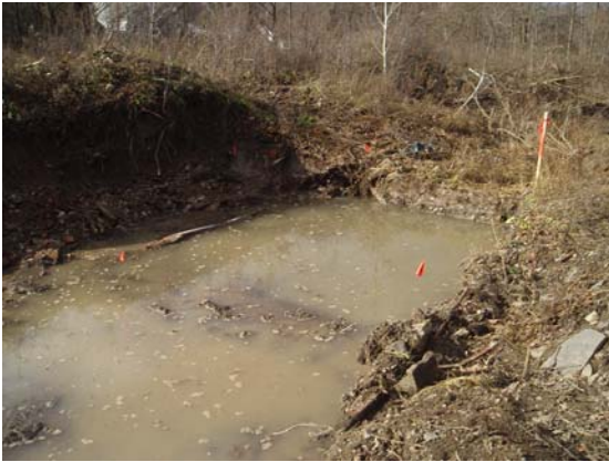
11/26/07 Water infiltration in the IRM excavation at the head of the Unnamed Ditch
