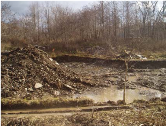
11/27/07 View of central portion of the two-foot IRM excavation looking southeast
