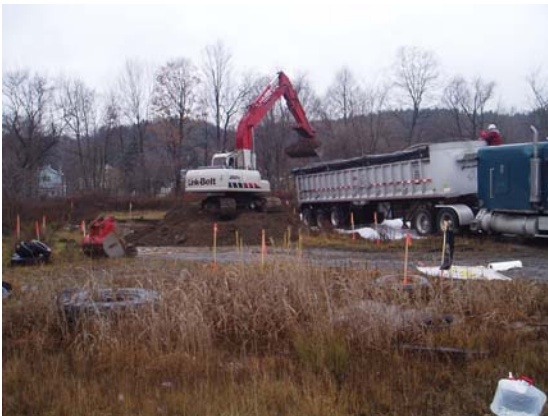
11/26/07 Loading PCB-impacted soil looking southwest
