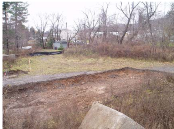
11/26/07 Southwest portion of the two-foot IRM excavation
