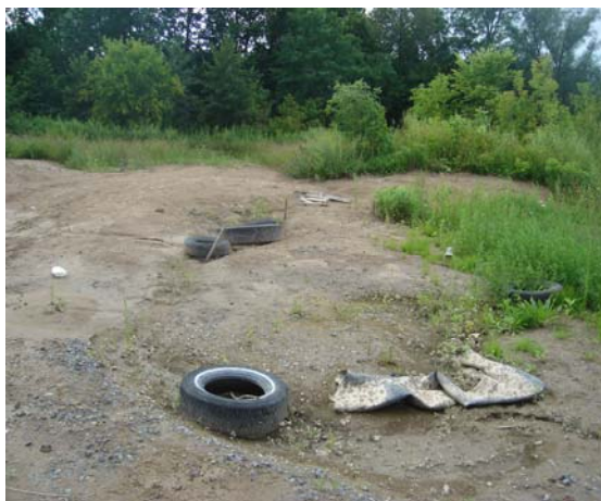
8/13/08 View of settlement areas filled with debris within backfilled IRM excavation
