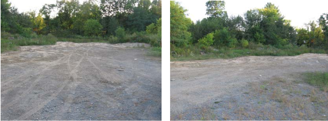
9/21/2008 View of Final Restoration of IRM excavation area
