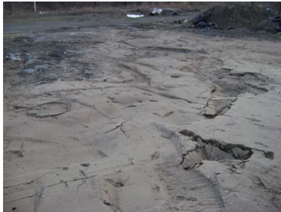
1/10/08 View of settlement within backfilled IRM excavation
