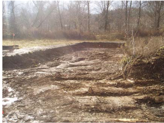
11/27/07 View of central and southern portion of the two-foot IRM excavation
