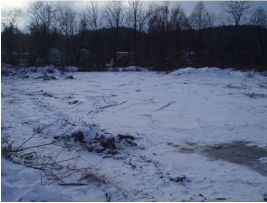
12/10/07 View of backfilled IRM excavation looking west
