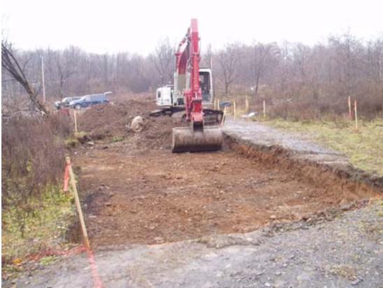
11/26/07 Two-foot excavation looking northeast
