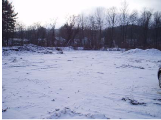
12/10/07 View of backfilled IRM excavation looking southwest
