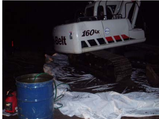
11/27/07 Decontamination pad with pump for decontamination of excavator tracks
