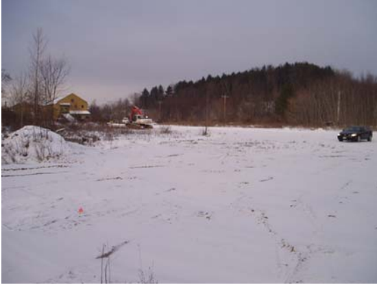
12/10/07 View of backfilled IRM excavation looking north
