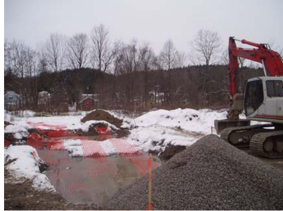
12/6/07 View of completed IRM excavation with snow fencing in place
