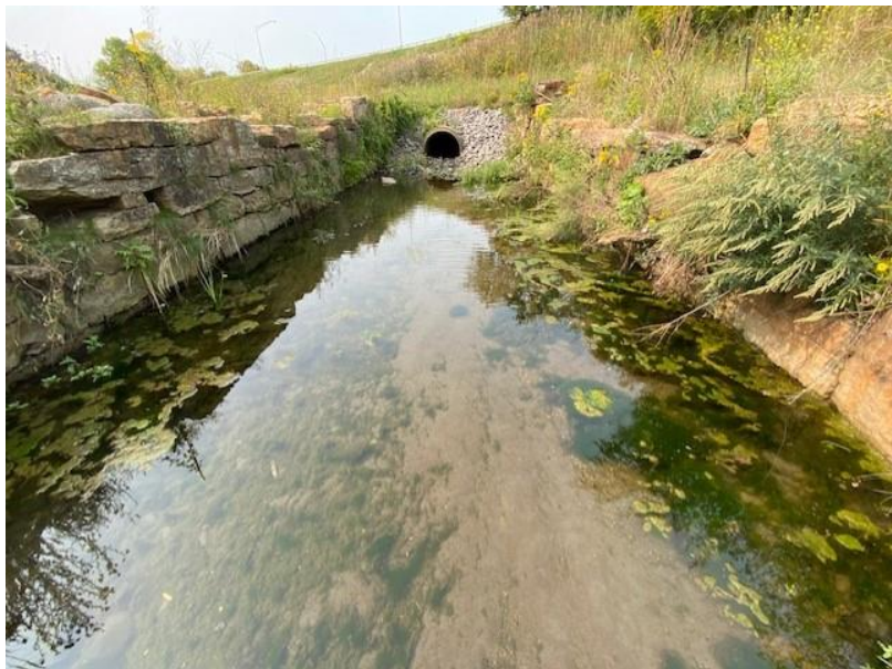
Segment A looking west at French Rd storm sewer culvert. Since 2018, road sand from culvert discharge has deposited on the restored canal bed.
