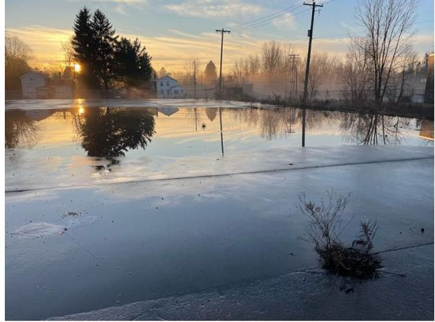
Ponding on northeast building slab
