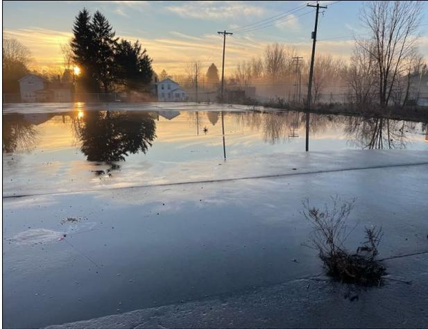
Ponding on the building slab on the northeast side of the site
