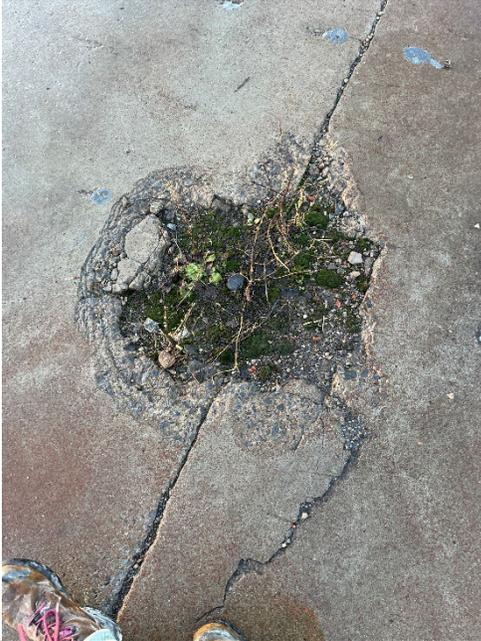
Minor Cracking and damage to building slab
