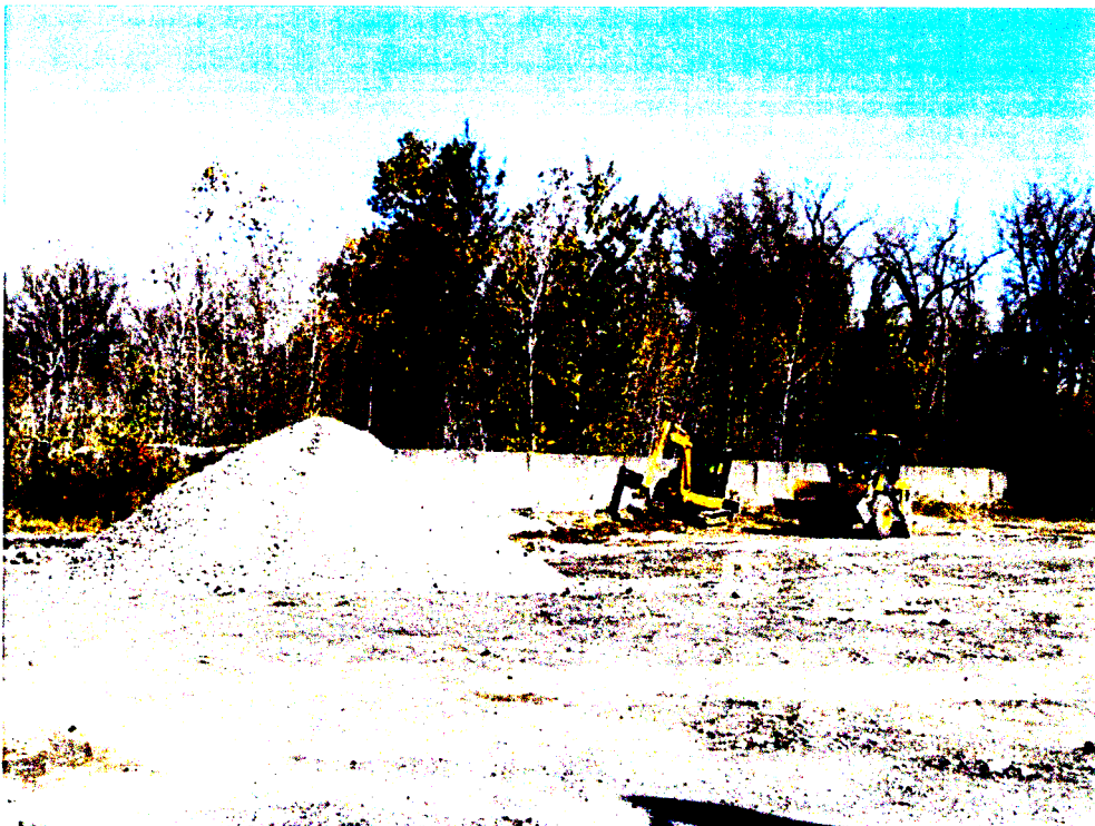
Photo #10: October 10, 2011 – Trenching drainage ditch around northern property line.
