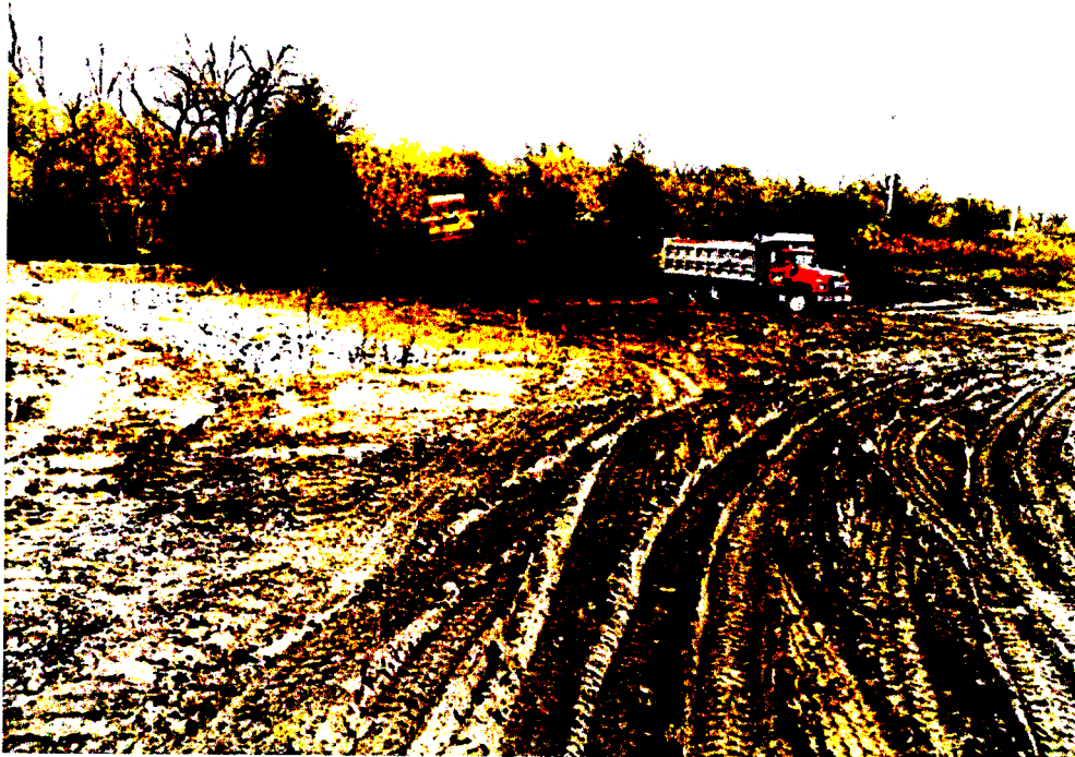
Photo #21: October 17, 2011 – Phase I: Loaded dump truck moving stage soil to new windrows.
