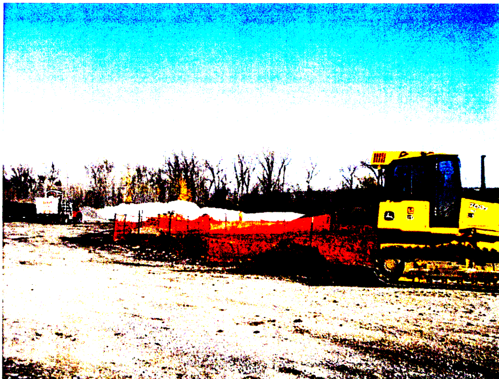
Photo #43: November 1, 2011 –Phase I: Completion of excavations and windows, winterization of site with orange snow fencing.
