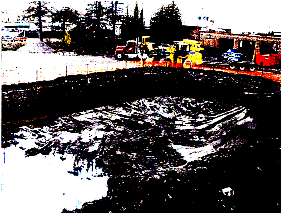
Photo #37: October 28, 2011 –Phase I: Completion of Excavation 3.
