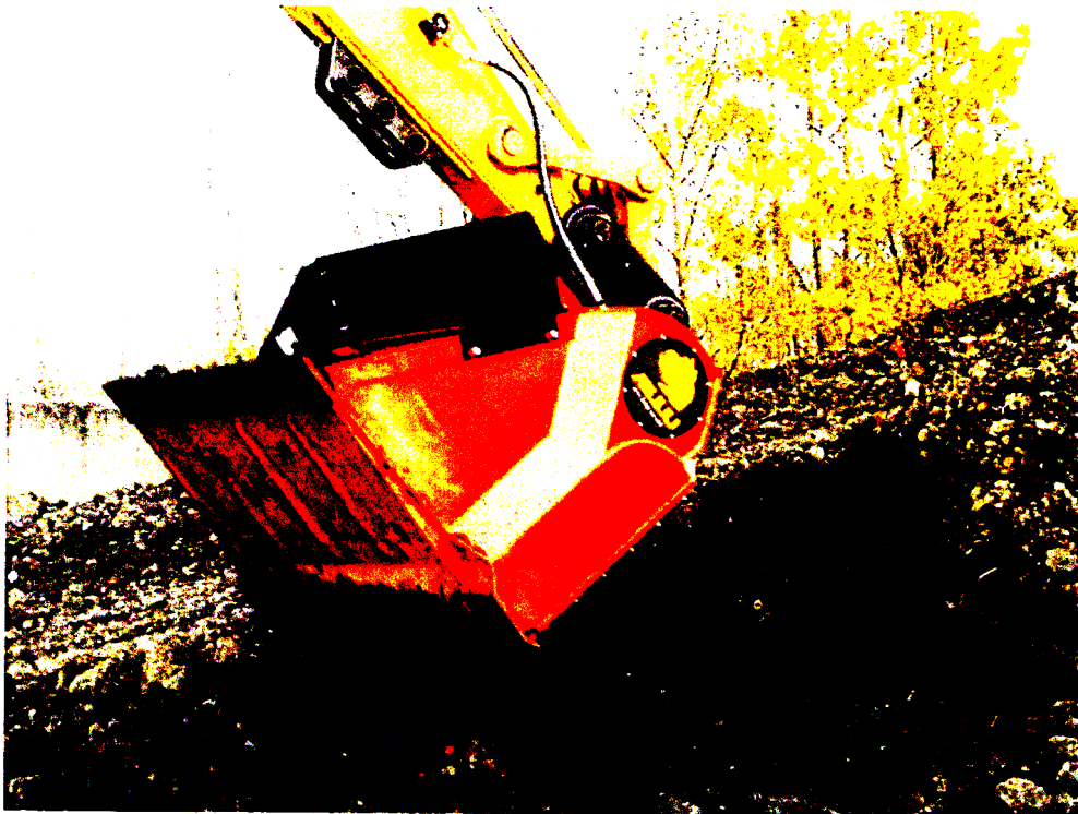
Photo #24: October 19, 2011 – Beginning of Phase II: Aeration of Windrow 1 via Allu excavator.
