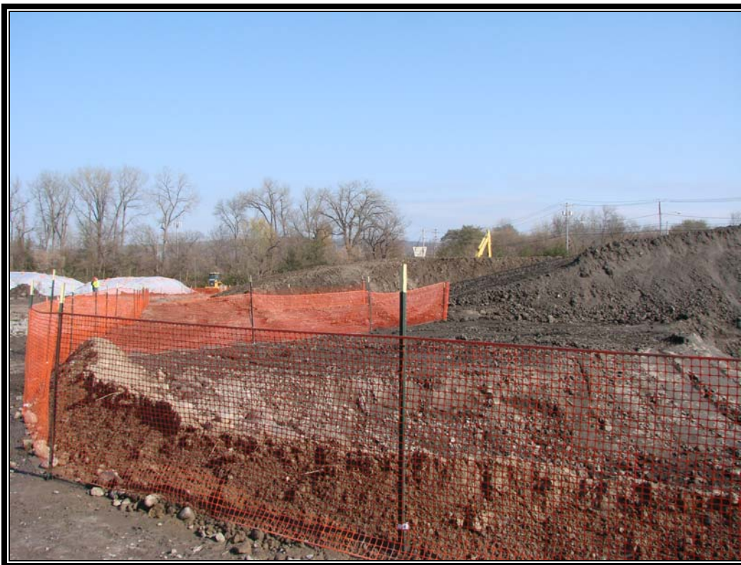
Photo #42: November 1, 2011 –Phase I: Completion of excavations and windows, winterization of site with orange snow fencing.
