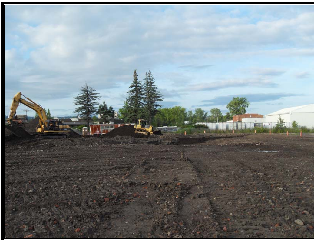
Photo #87: August 13, 2012 – Phase II: Continue backfilling and alluing soils
