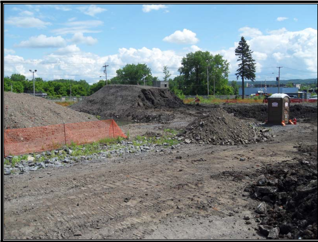
Photo #65: June 7, 2012 –Phase II: Start excavating and alluving Windrow 5 within the excavation area.
