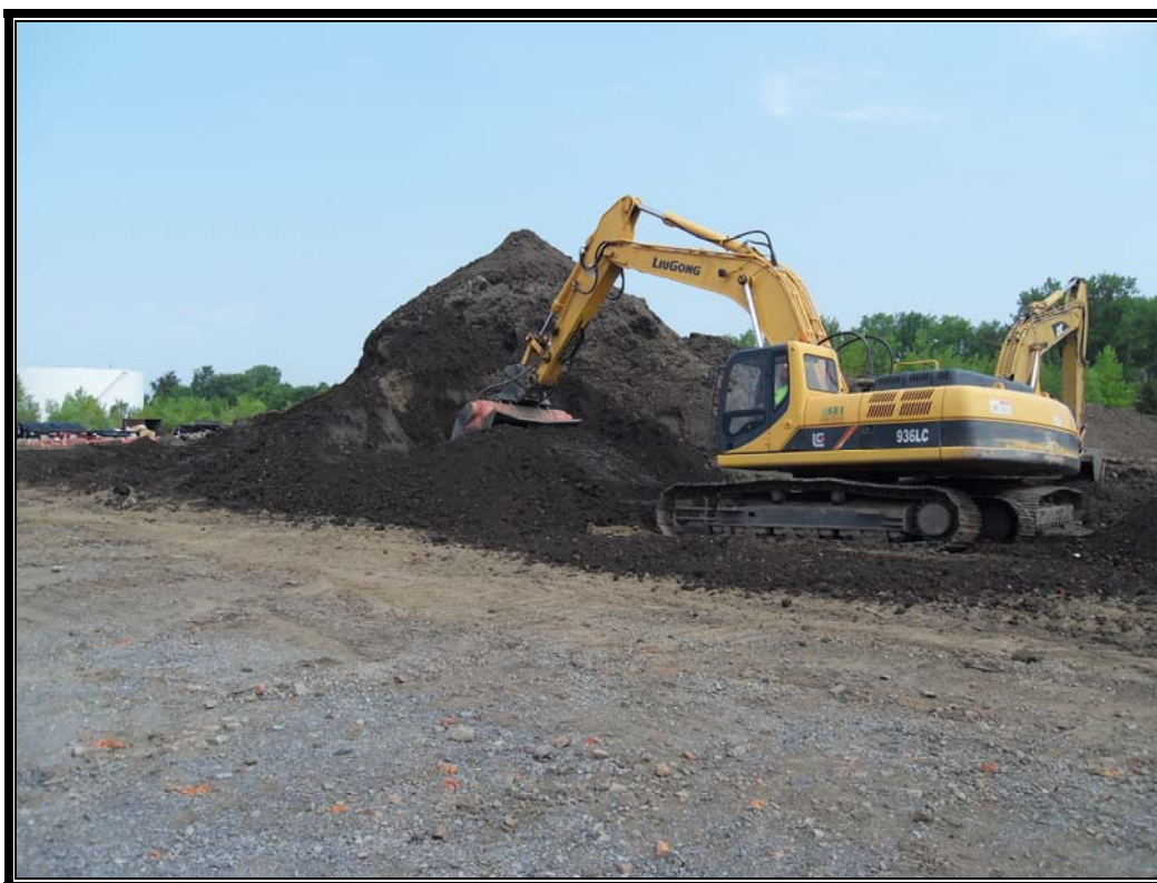
Photo #82: July 17, 2012 – Phase II: Continue Alluvium.
