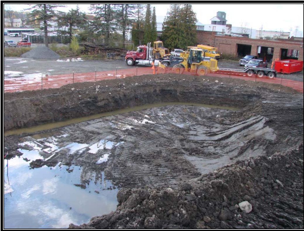
Photo #37: October 28, 2011 –Phase I: Completion of Excavation 3.
