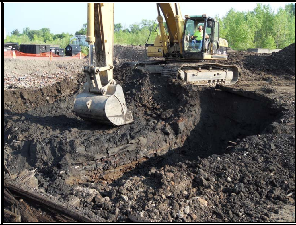
Photo #79: July 10, 2012 – Phase II: Continue excavating east of the former building.
