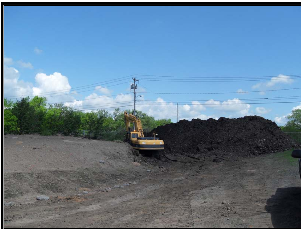
Photo #62: May 23, 2012 –Phase II: Continue alluing Windrow 3 into stockpile.
