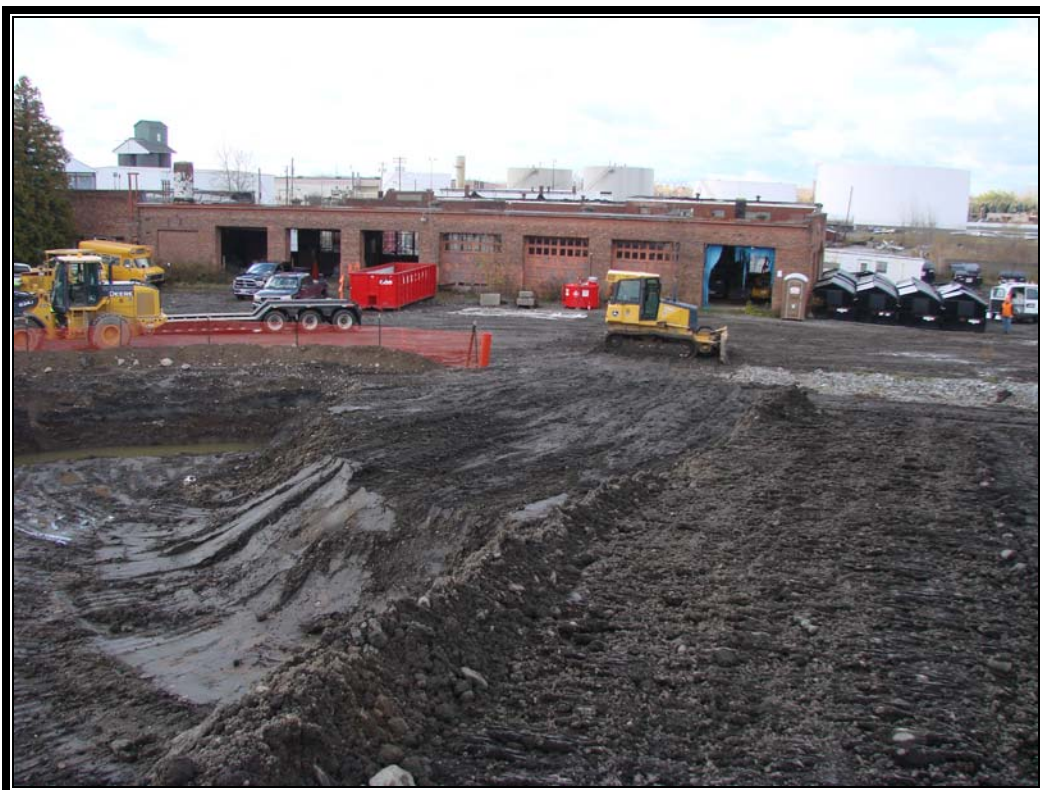
Photo #38: October 28, 2011 –Phase I: Completion of Excavation 3, and Windrow 5.
