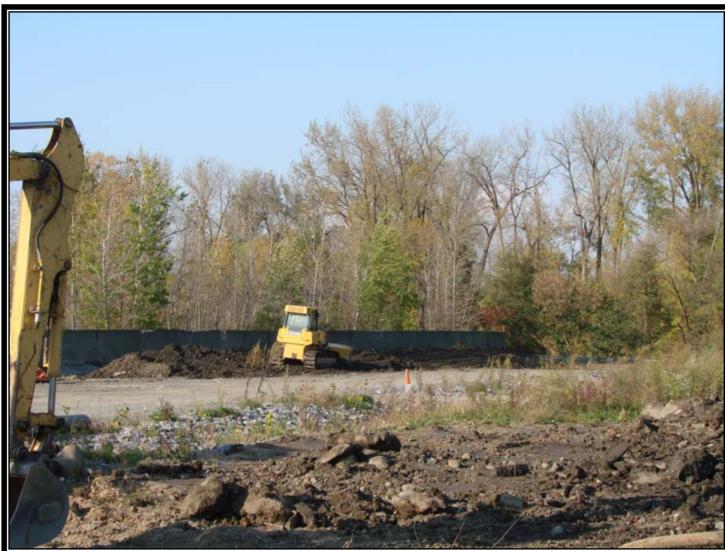
Photo #12: October 10, 2011 – Phase I: Staging new windrows in northwest corner of property.
