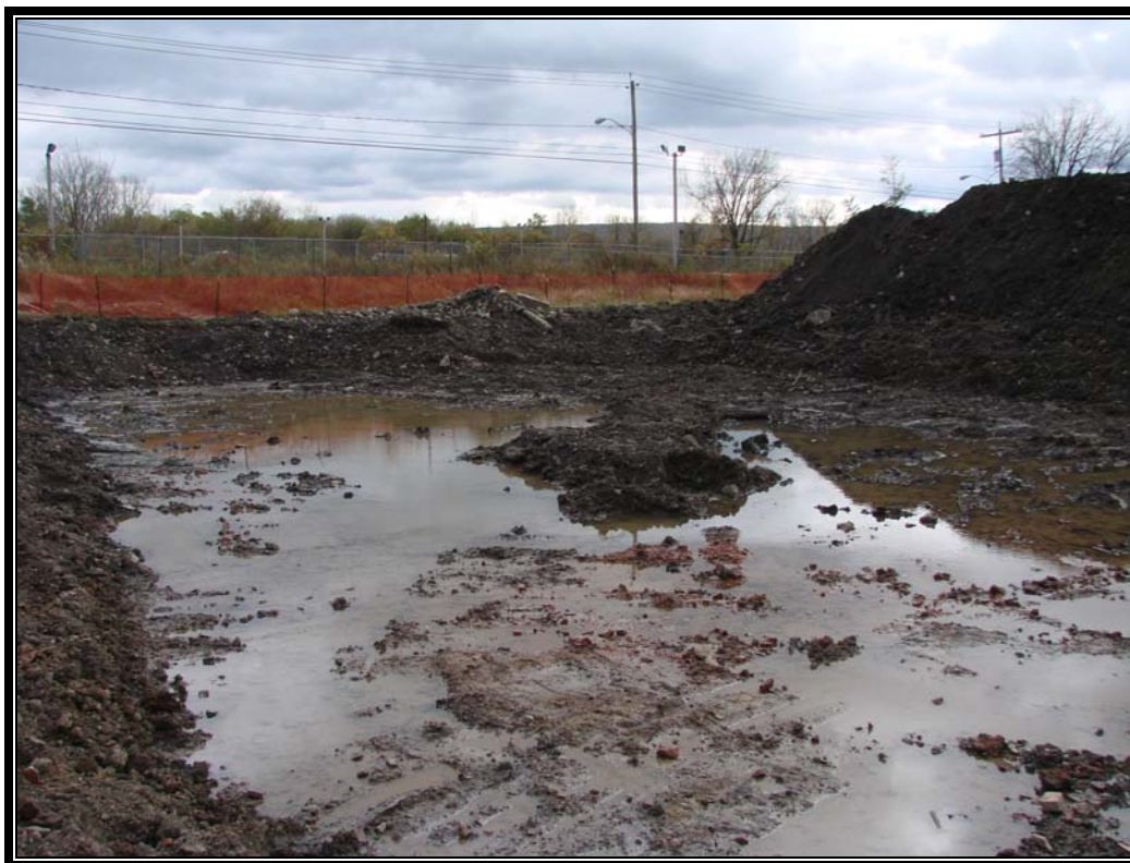
Photo #29: October 21, 2011 –Phase I: Completion of Excavation 1.
