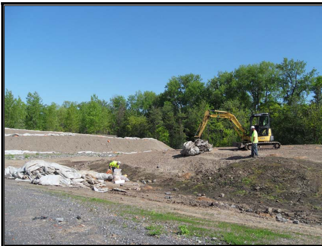
Photo #56: May 21, 2012 –Phase II: Removing plastic sheeting from 2011 winterization activities.
