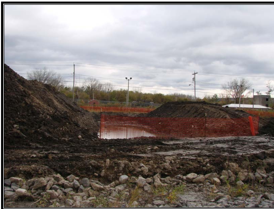
Photo #30: October 21, 2011 –Phase I: Completion of Excavation 2, to ~4.5 to 5 fbg.
