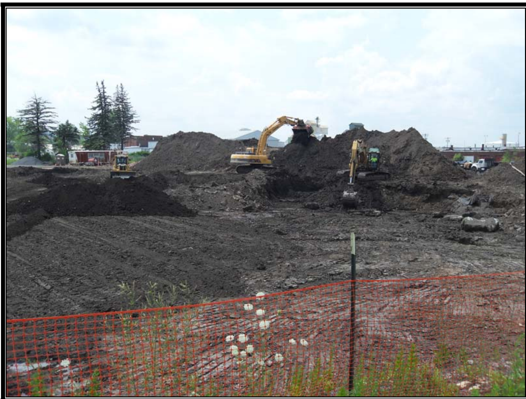
Photo #80: July 16, 2012 – Phase II: Continue excavating and alluing.
