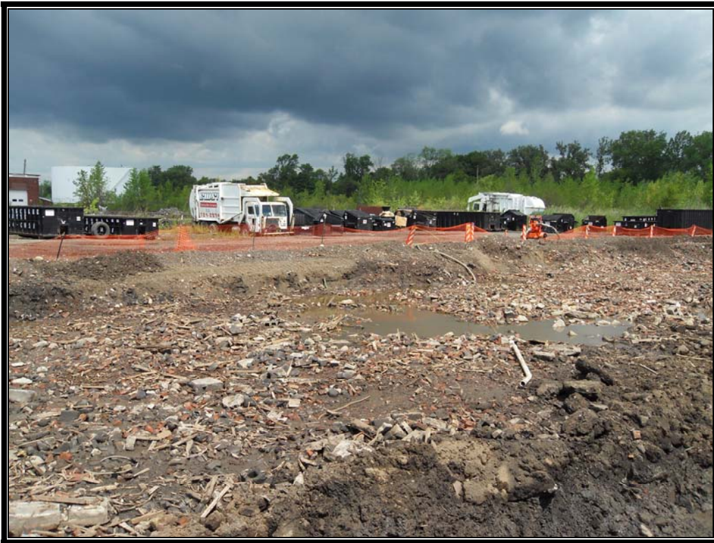
Photo #85: July 24, 2012 – Phase II: Former building excavation backfilled with brick.
