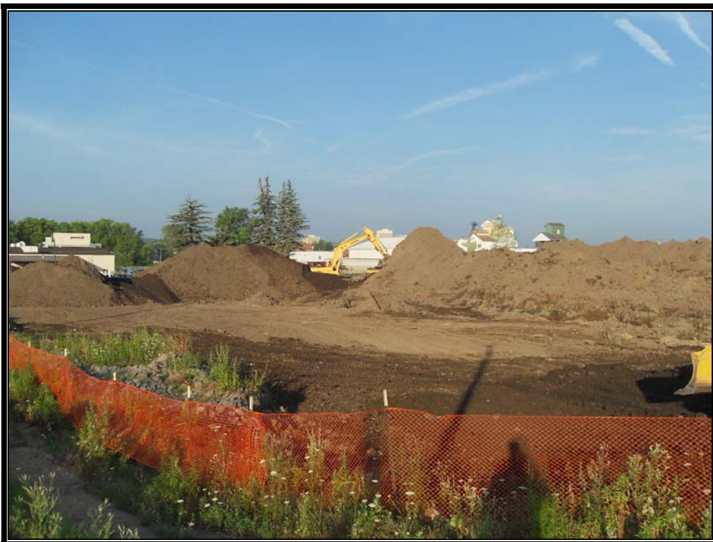
Photo #84: July 19, 2012 – Phase II: Backfilled excavation and remaining soil to be alluded.
