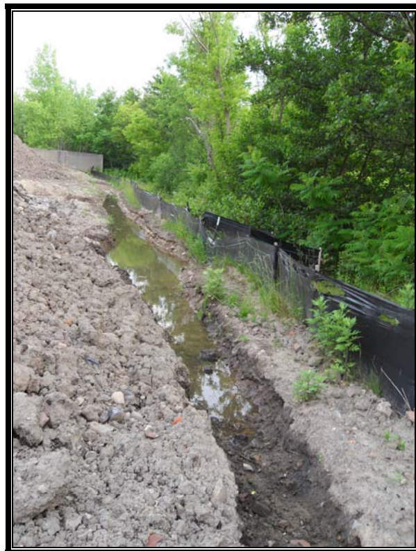
Photo #72: June 8, 2012 – Phase II: Dewatering activities. On-site drainage trench.
