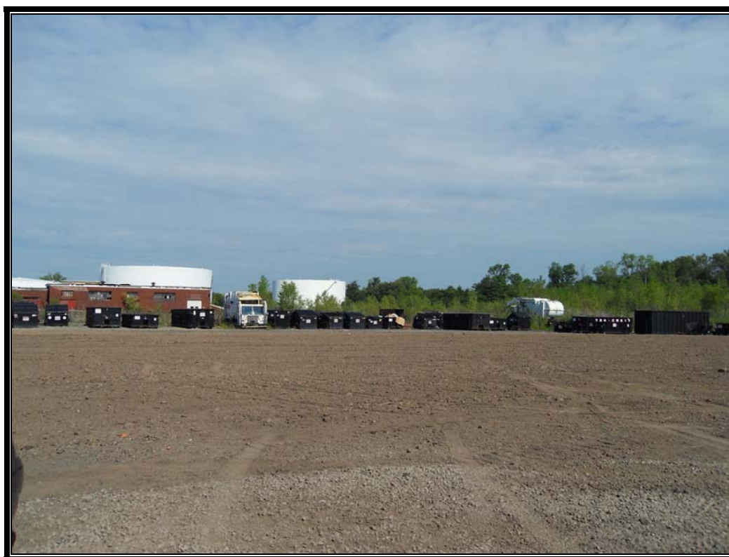
Photo #96: August 20, 2012 –Phase II: Final restoration and grading.
