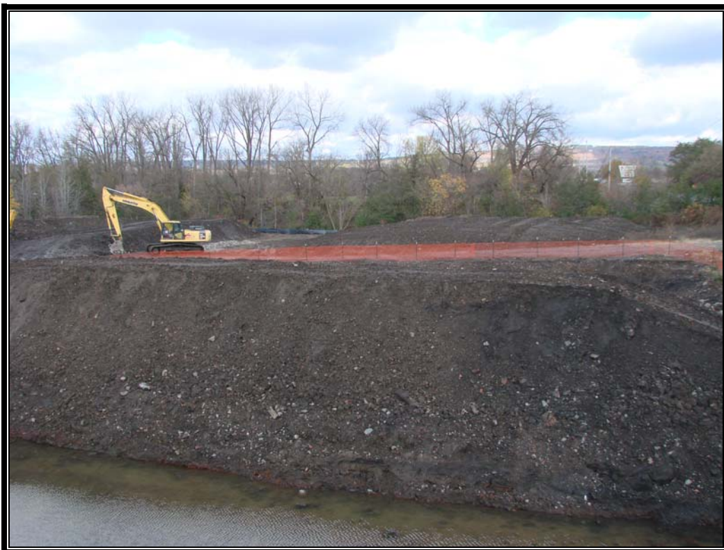
Photo #40: October 28, 2011 –Phase I: Completion of dressing Windrow 3.
