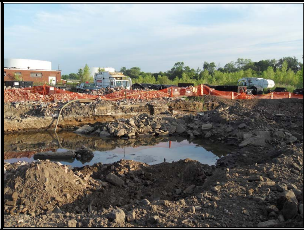
Photo #83: July 19, 2012 – Phase II: Dewatering excavation under former building.
