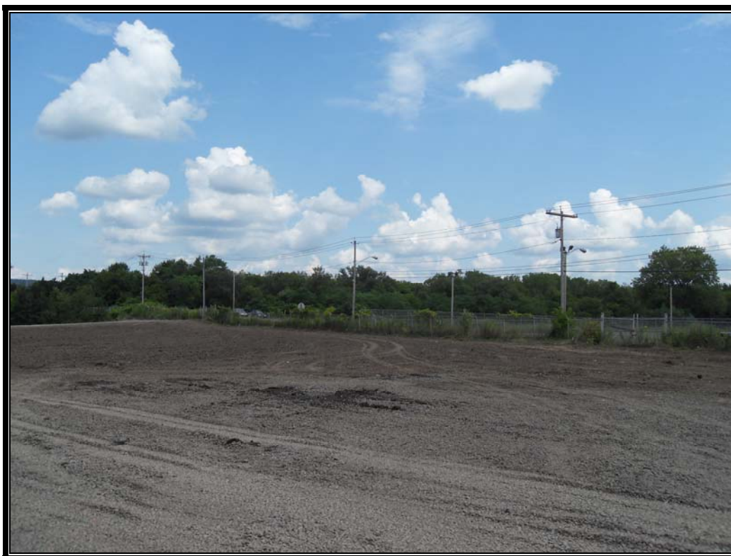
Photo #98: August 20, 2012 –Phase II: Final restoration and grading.
