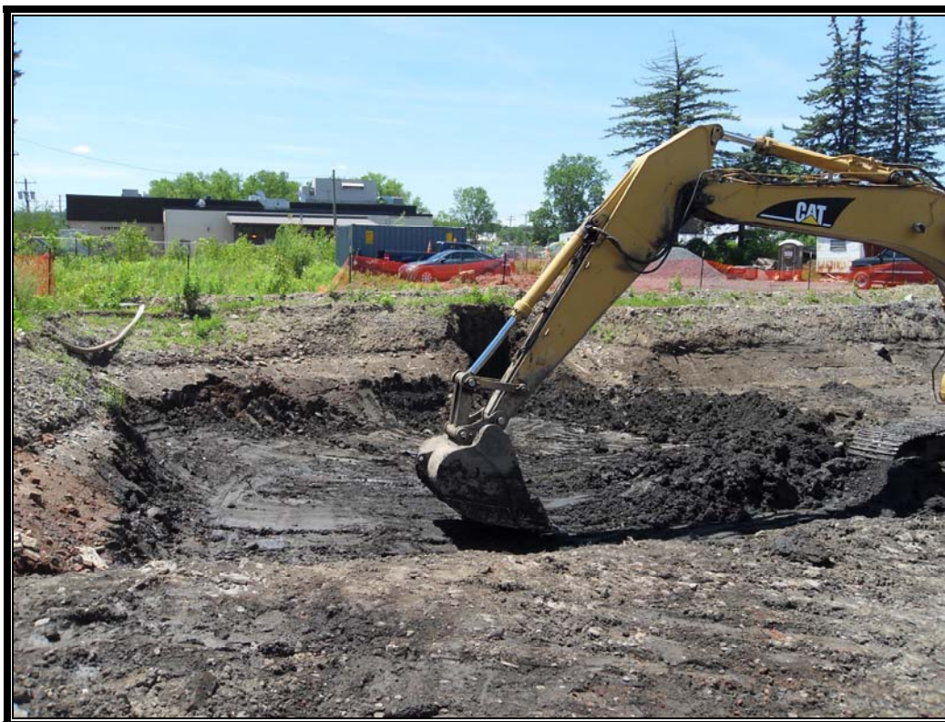
Photo #73: June 14, 2012 – Phase II: Started excavating within excavation 3.
