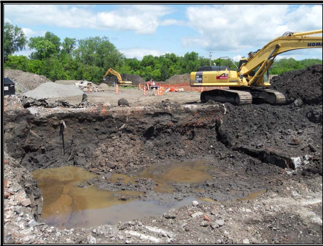
Photo #64: May 31, 2012 –Phase II: Started alluing Windrow and started excavating under the former building.
