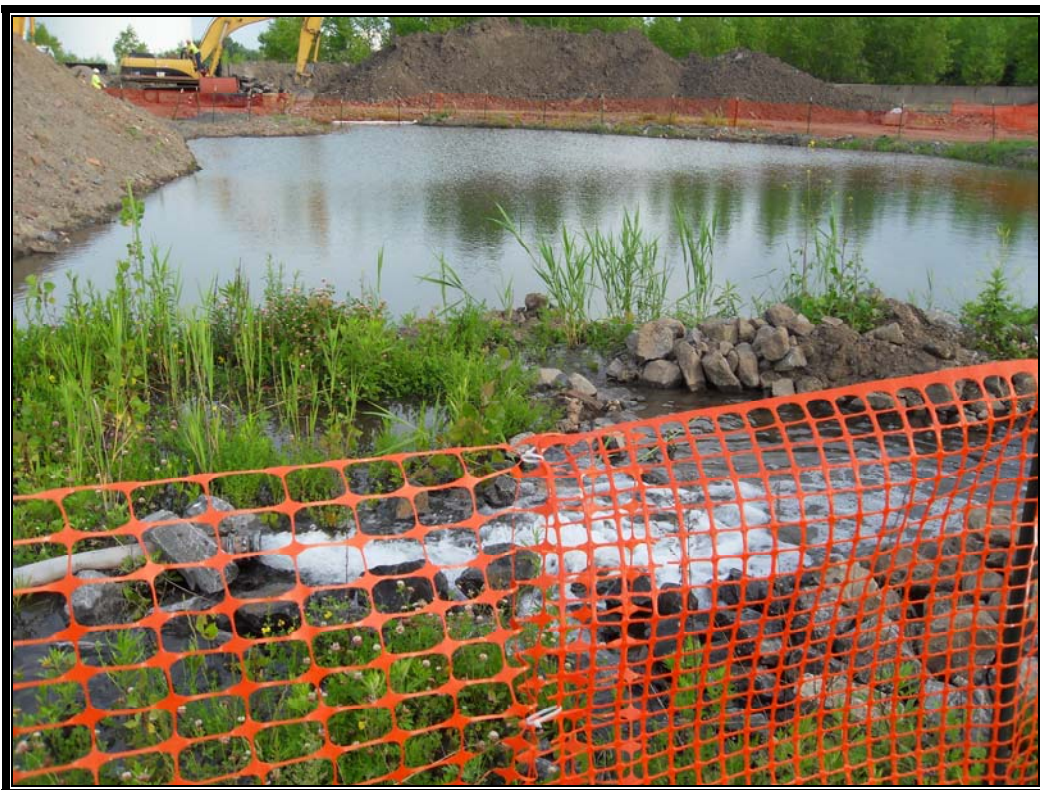
Photo #68: June 8, 2012 –Phase II: Dewatering activities. Settling pond.
