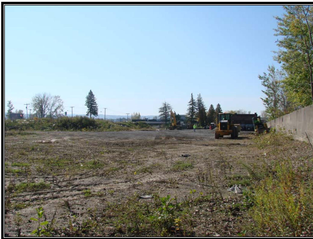
Photo #5: October 10, 2011 – Pre-excavation site photo.
