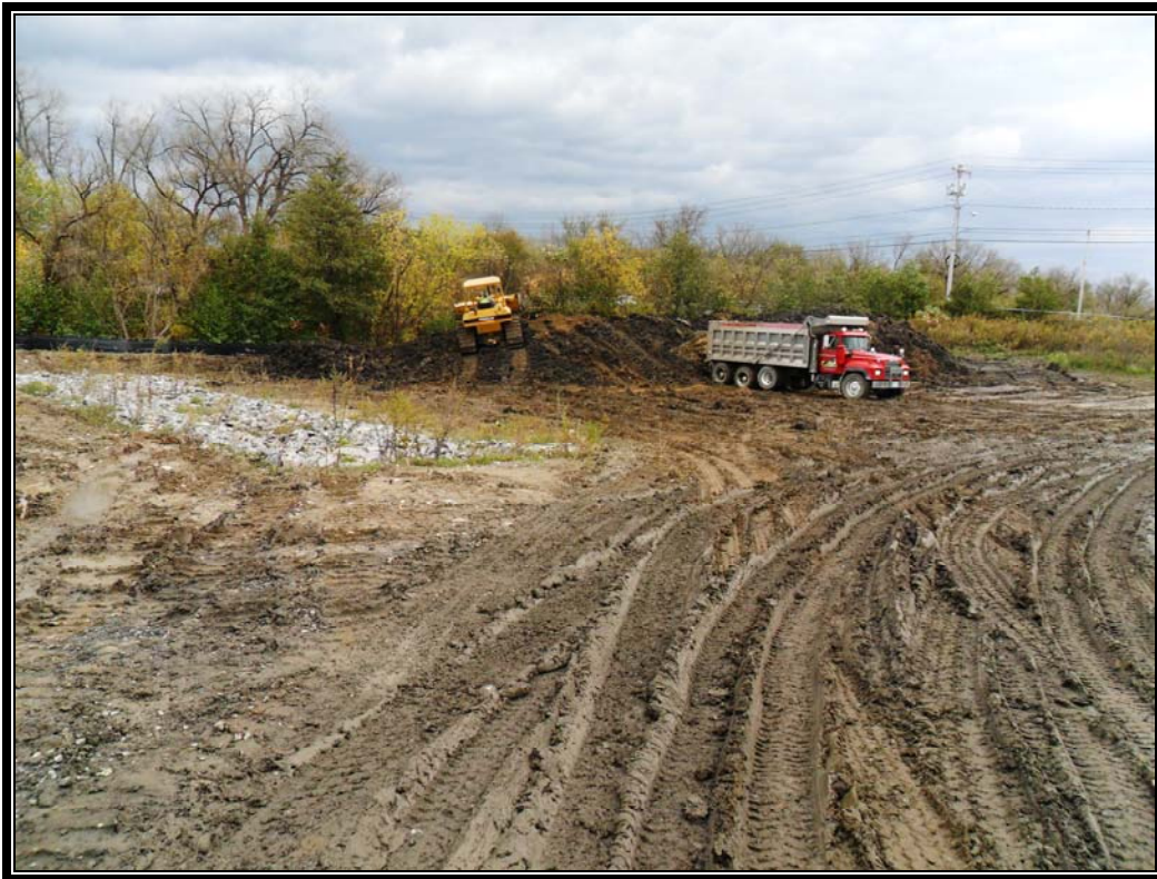
Photo #21: October 17, 2011 – Phase I: Loaded dump truck moving stage soil to new windrows.
