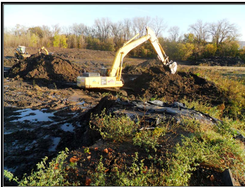
Photo #19: October 17, 2011 – Phase I: Excavating the 3 rd staged soil pile.
