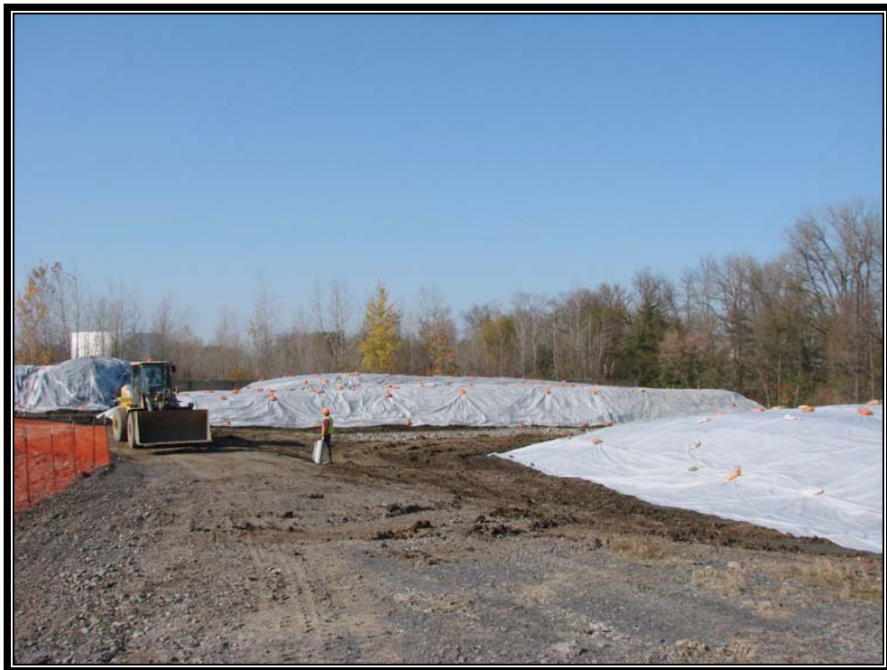
Photo #52: November 1, 2011 –Phase I: Winterization of windrows with plastic sheeting and sand bags to reduce potential run off.
