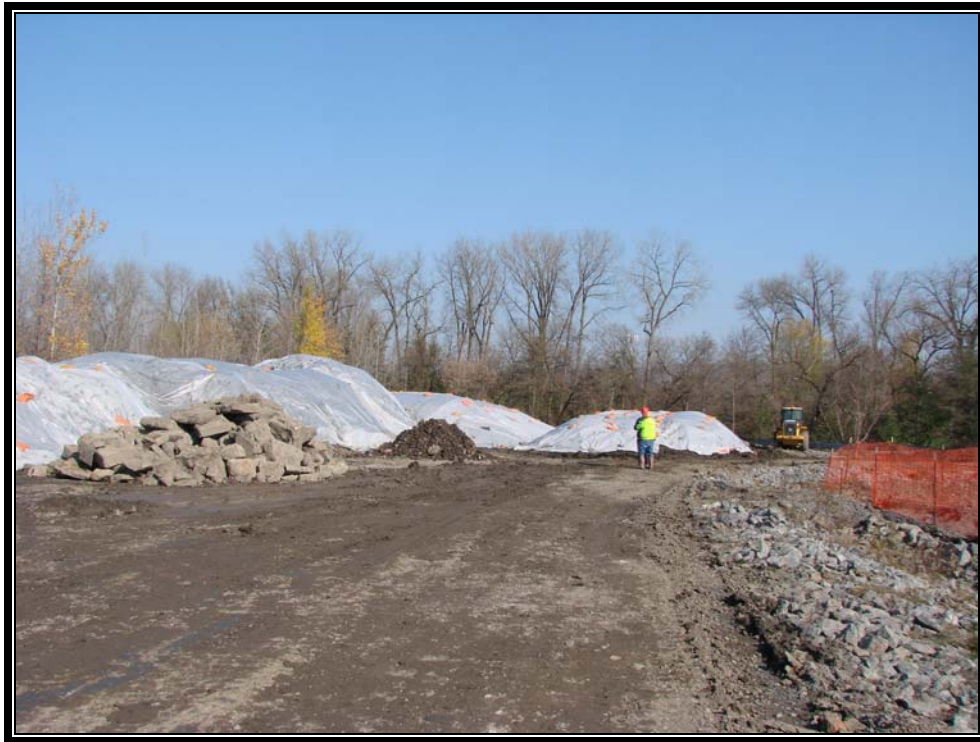
Photo #53: November 1, 2011 –Phase I: Winterization of windrows with plastic sheeting and sand bags to reduce potential run off.
