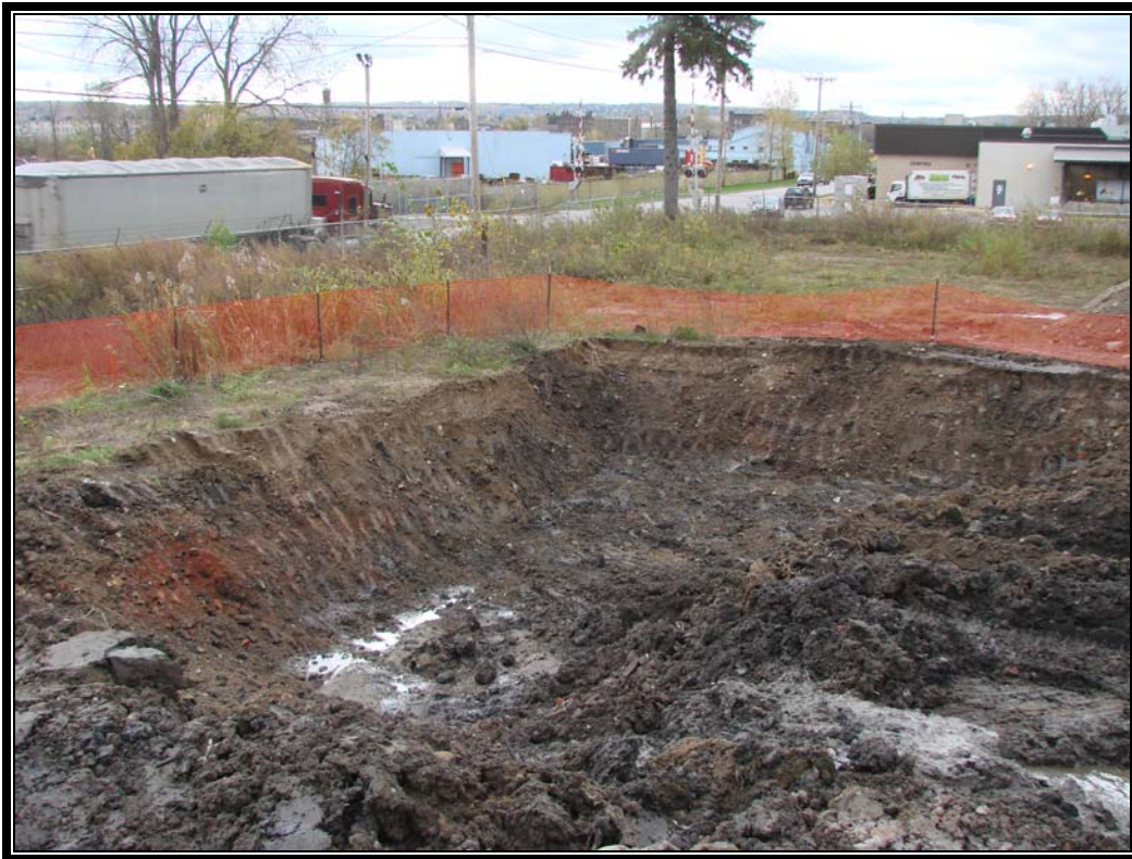
Photo #33: October 21, 2011 –Phase I: Beginning of Excavation 3.
