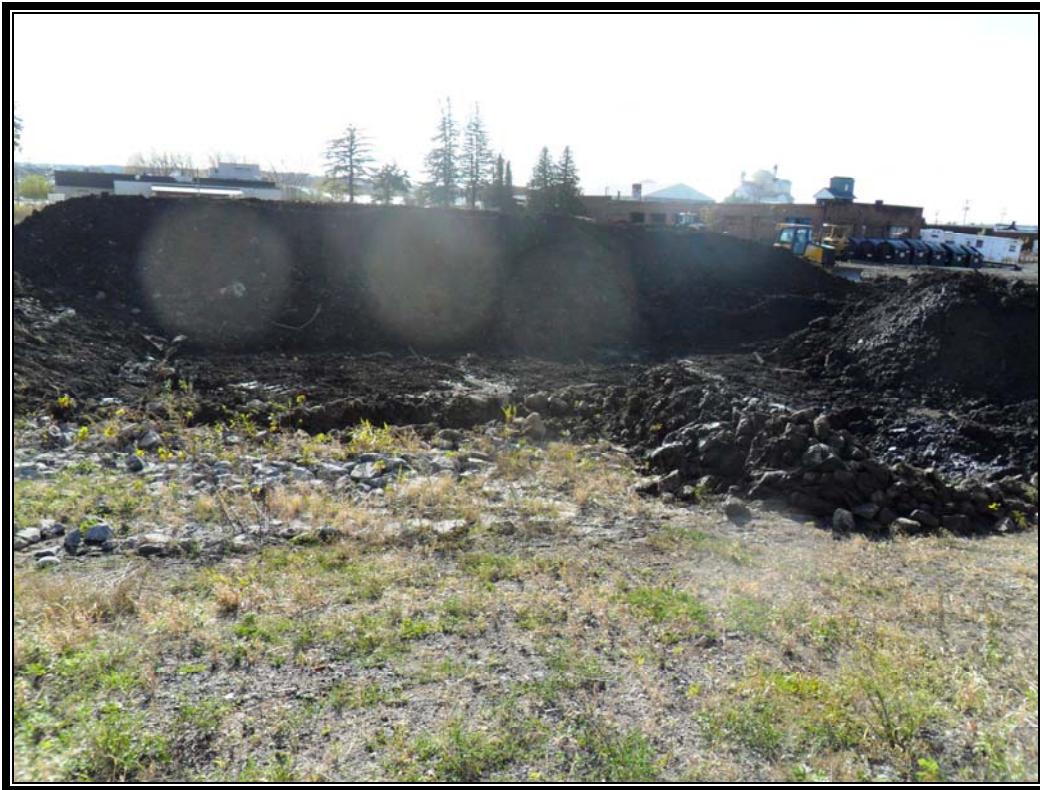
Photo #23: October 18, 2011 – Phase I: Excavation 1 and Window 4.
