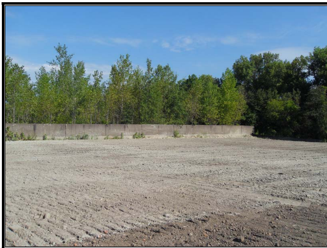
Photo #94: August 20, 2012 –Phase II: Final restoration and grading.
