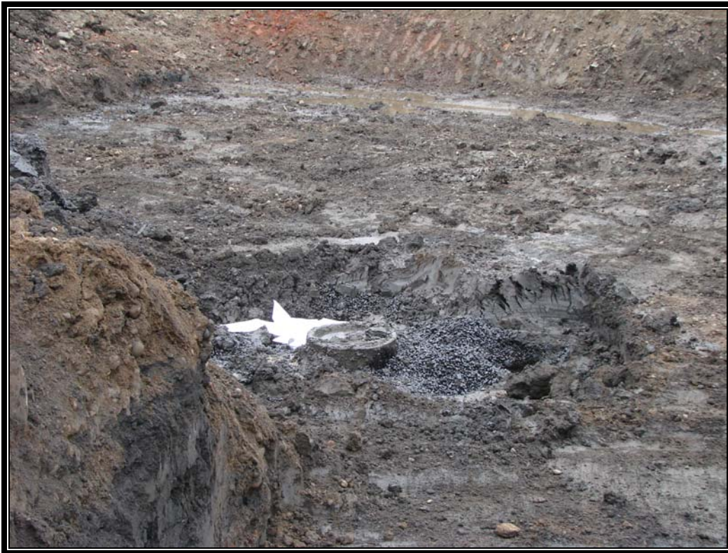
Photo #35: October 24, 2011 –Phase I: Uncovered a former in-active drain within Excavation 3.
