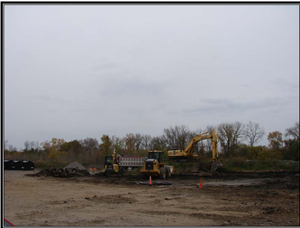
Photo #16: October 12, 2011 – Phase I: Loading staged soil into dump trucks, which then dump into the new windrows.
