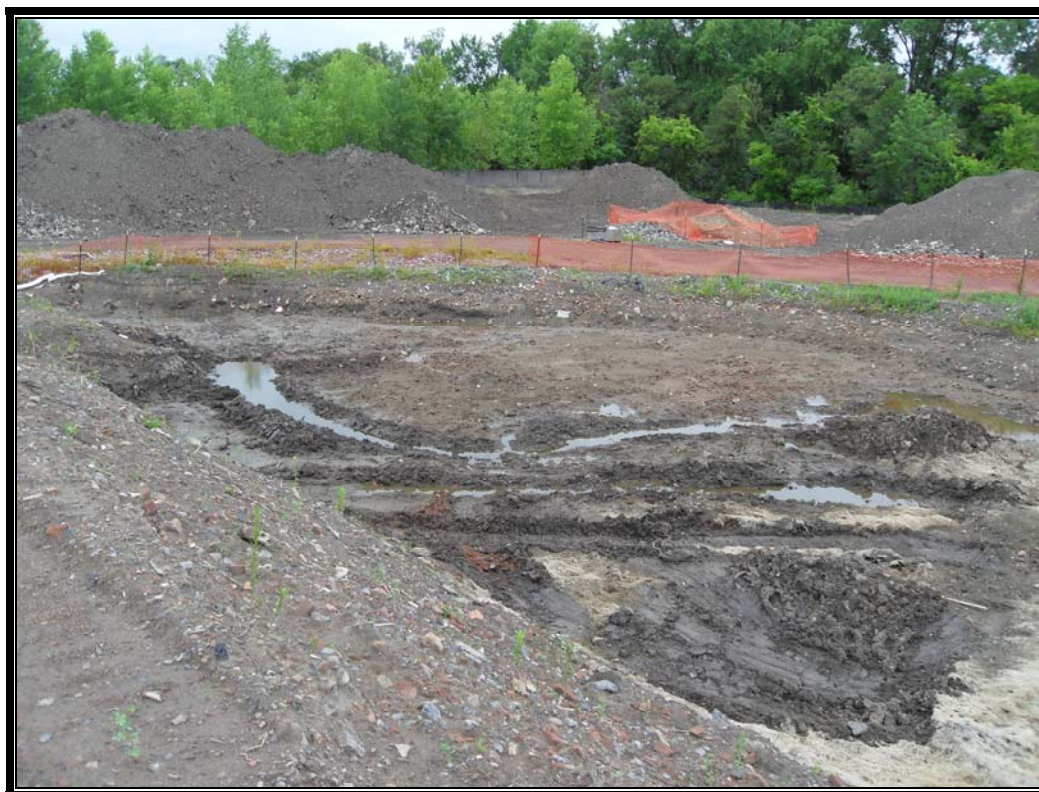
Photo #76: June 26, 2012 – Phase II: Dewatered excavation 1.
