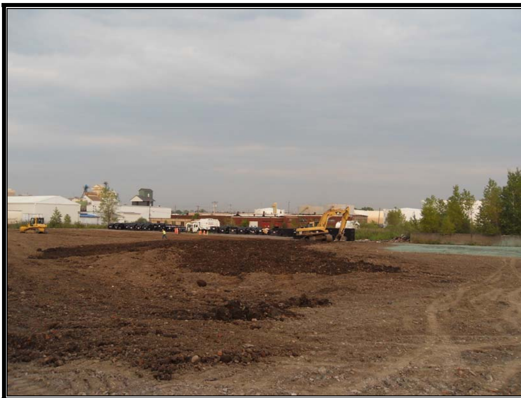
Photo #91: August 17, 2012 –Phase II: Continue grading and alluing remaining soils.
