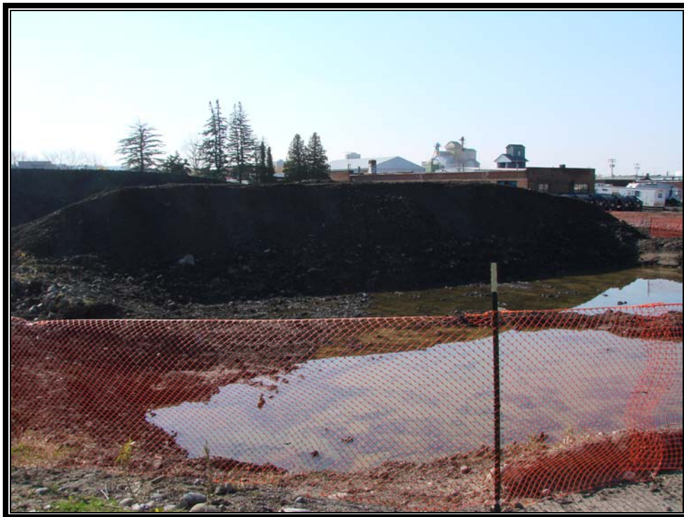
Photo #46: November 1, 2011 –Phase I: Completion of excavations and windows, winterization of site with orange snow fencing.
