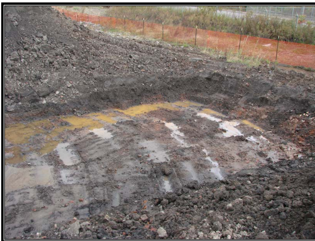
Photo #31: October 21, 2011 –Phase I: Completion of Excavation 2.
