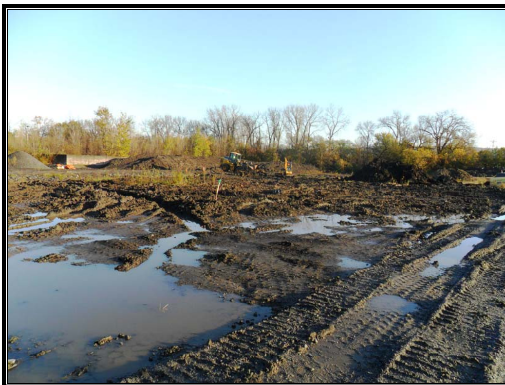
Photo #20: October 17, 2011 – Phase I: 1 st and 2 nd staged soil piles completed.
