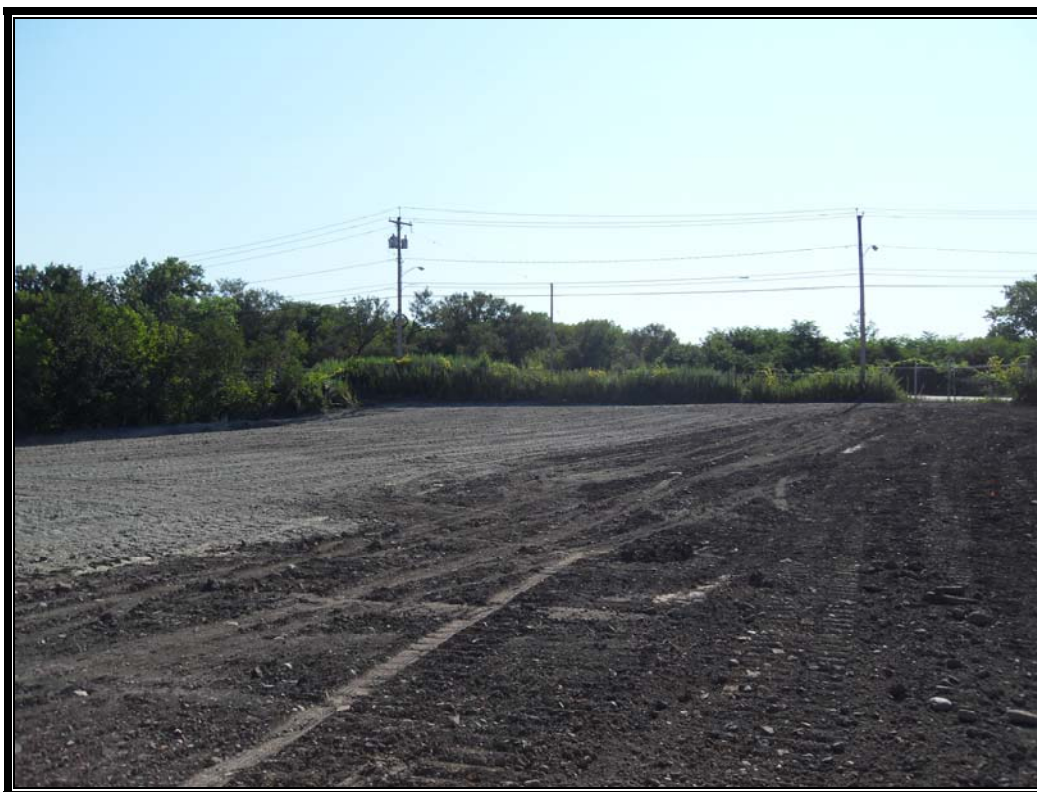
Photo #92: August 20, 2012 –Phase II: Final restoration and grading.
