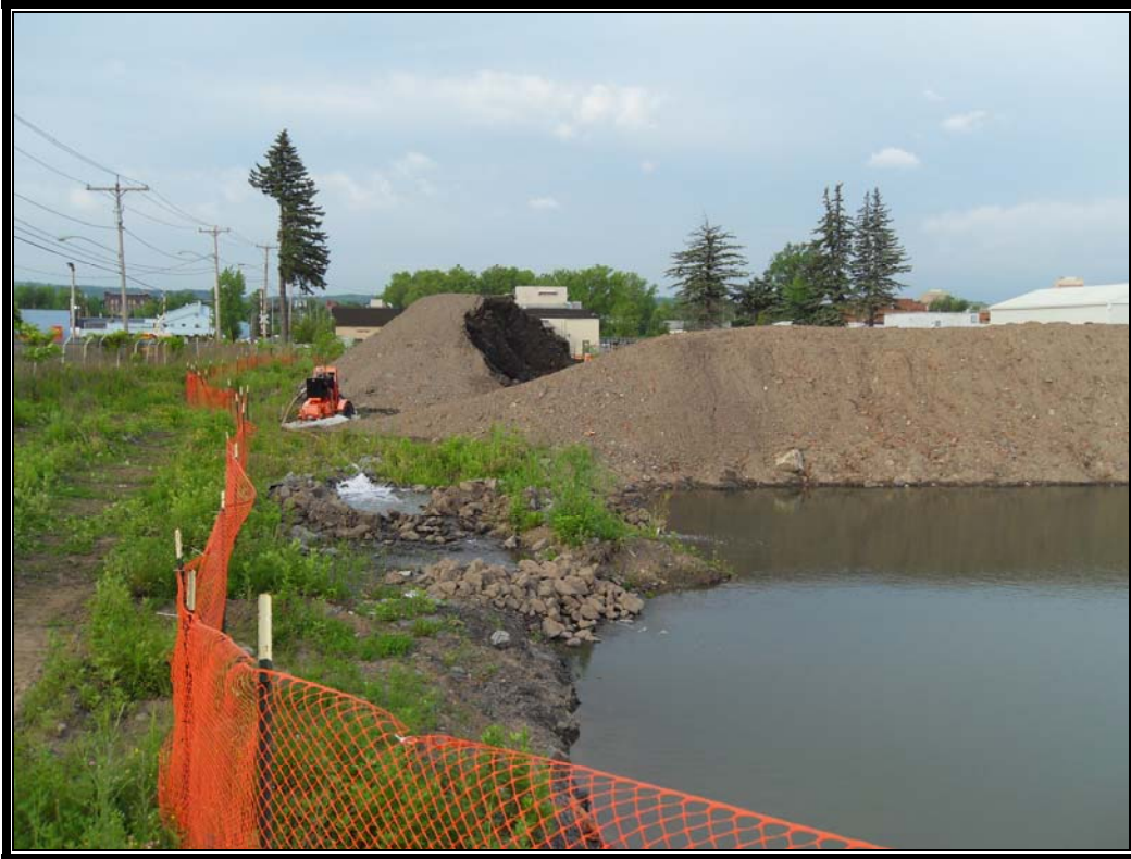
Photo #67: June 8, 2012 –Phase II: Dewatering activities. Pumping from Excavation 2 into Excavation 1.
