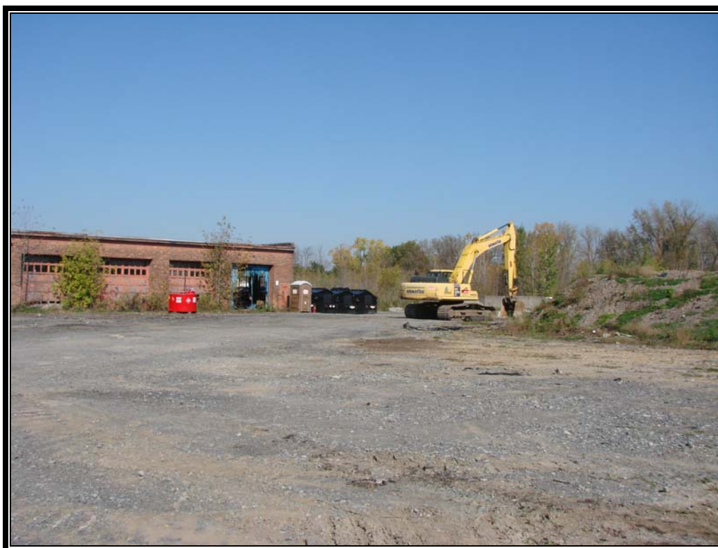
Photo #2: October 10, 2011 – Pre-excavation site photo.
