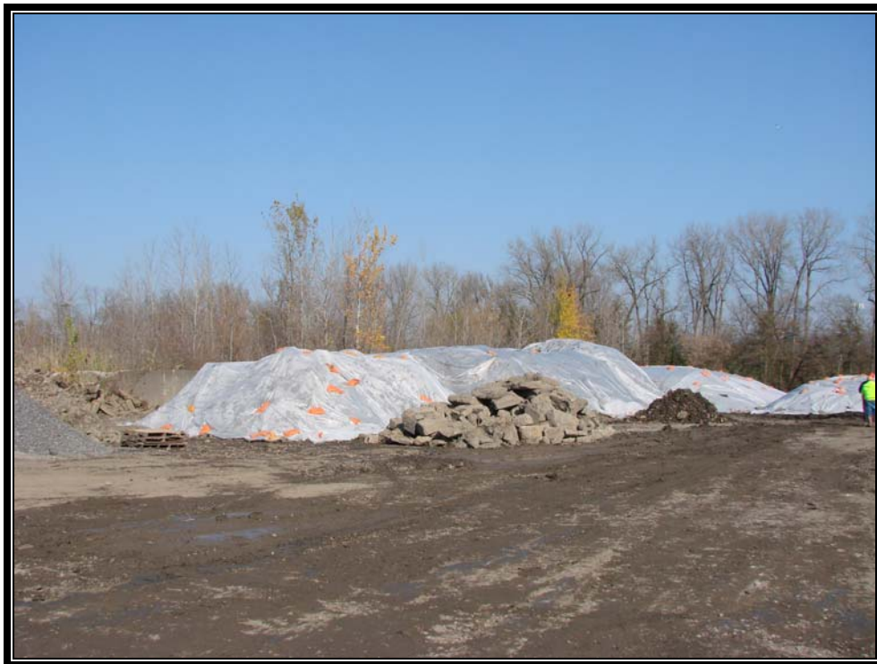
Photo #54: November 1, 2011 –Phase I: Winterization of windrows with plastic sheeting and sand bags to reduce potential run off.
