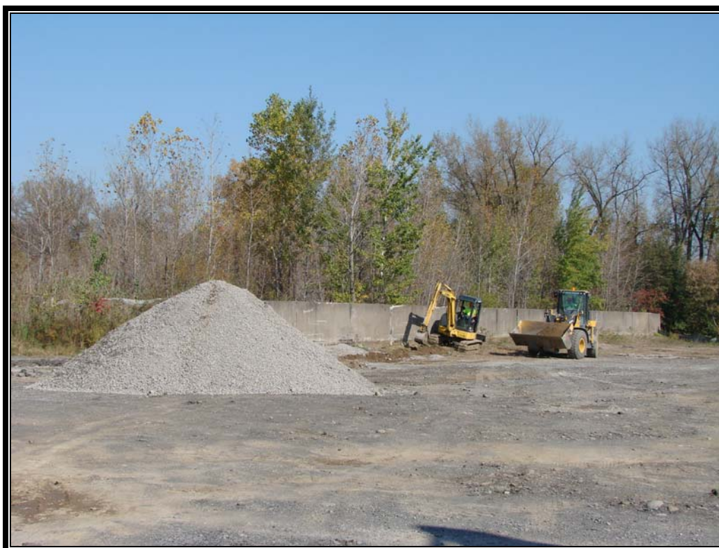
Photo #10: October 10, 2011 – Trenching drainage ditch around northern property line.
