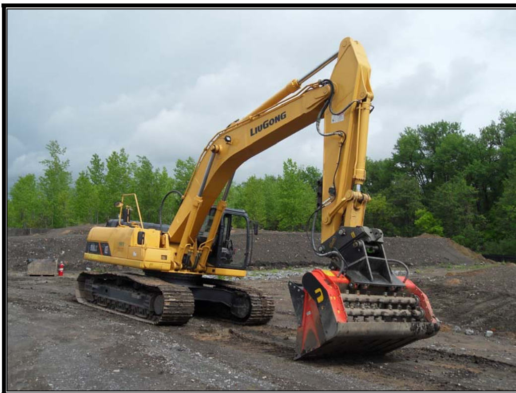
Photo #60: May 22, 2012 –Phase II: Allu TM Excavator.
