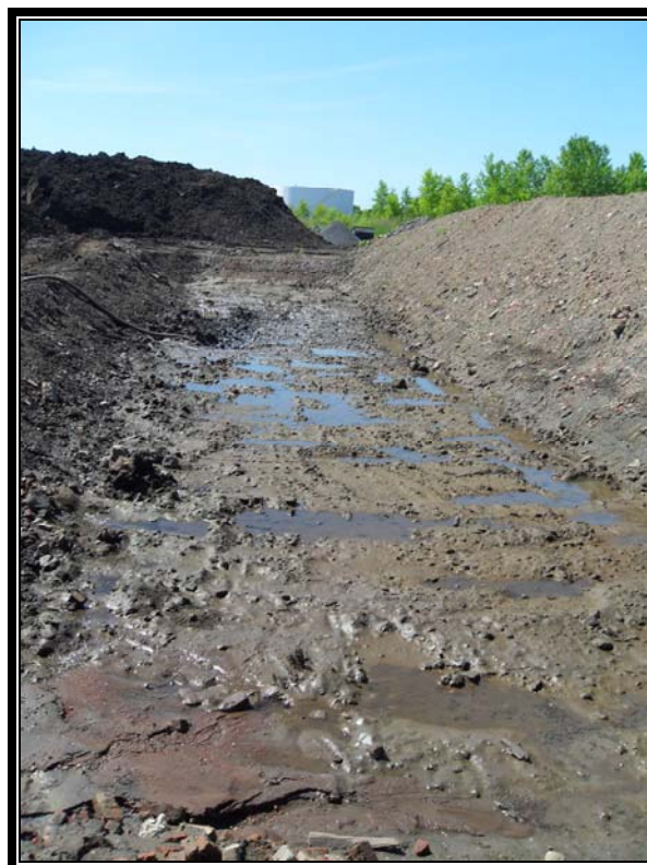
Photo #74: June 14, 2012 – Phase II: Dewatered excavation 2.
