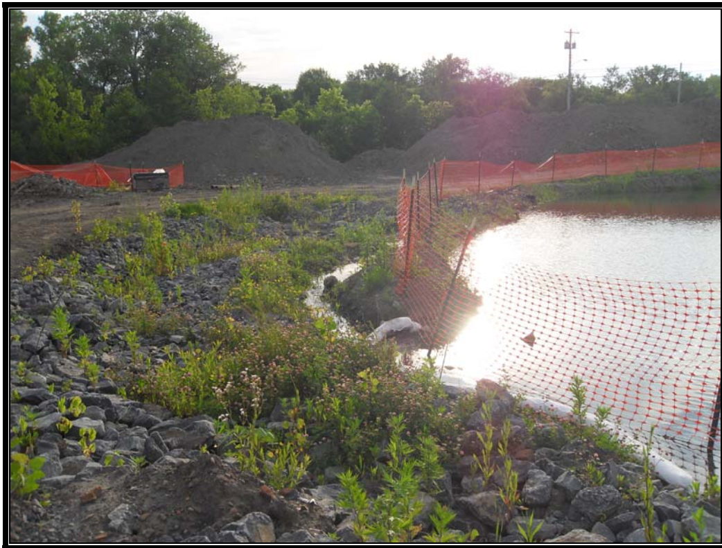
Photo #70: June 8, 2012 –Phase II: Dewatering activities. Water flowing out of Excavation 1 along the NW side.
