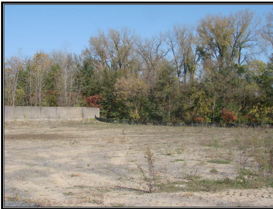
Photo #9: October 10, 2011 – Installation of silt fencing along northern property line.
