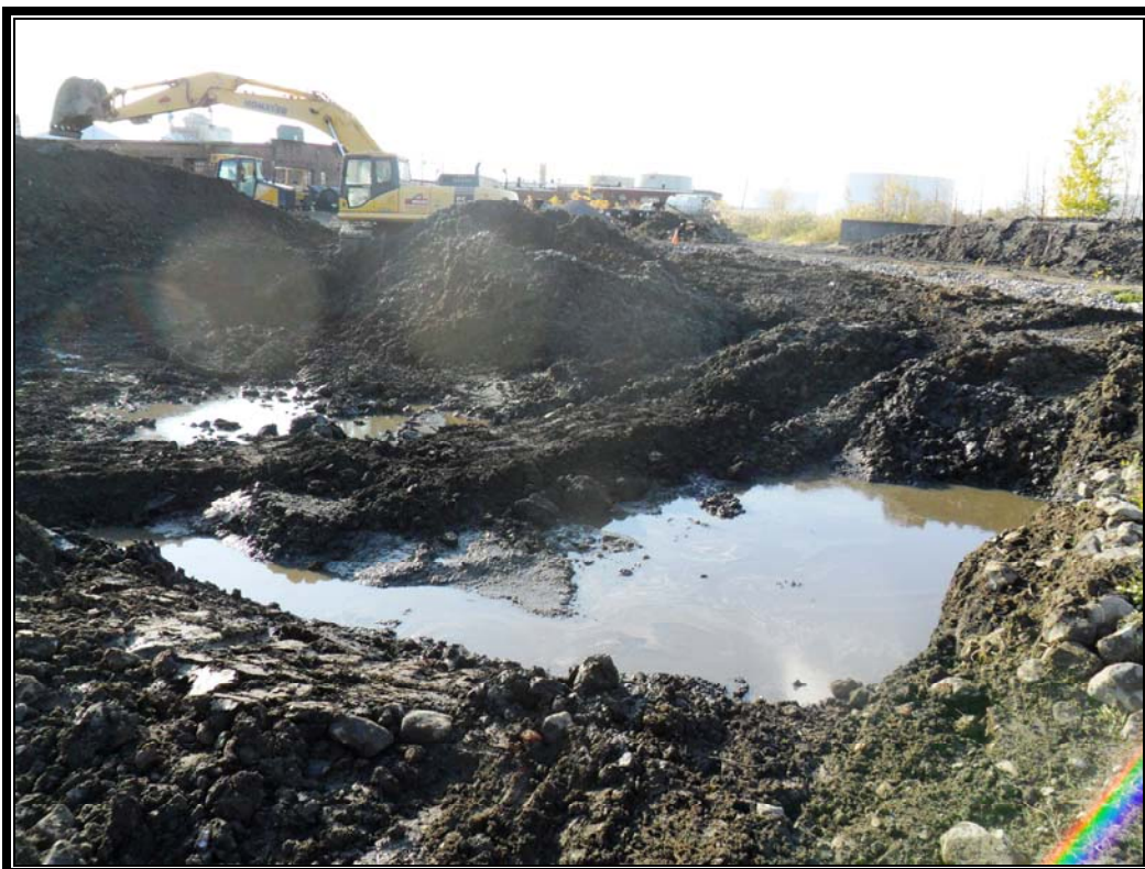
Photo #22: October 18, 2011 – Phase I: Beginning Excavation 1, and staging new Windrow 4.
