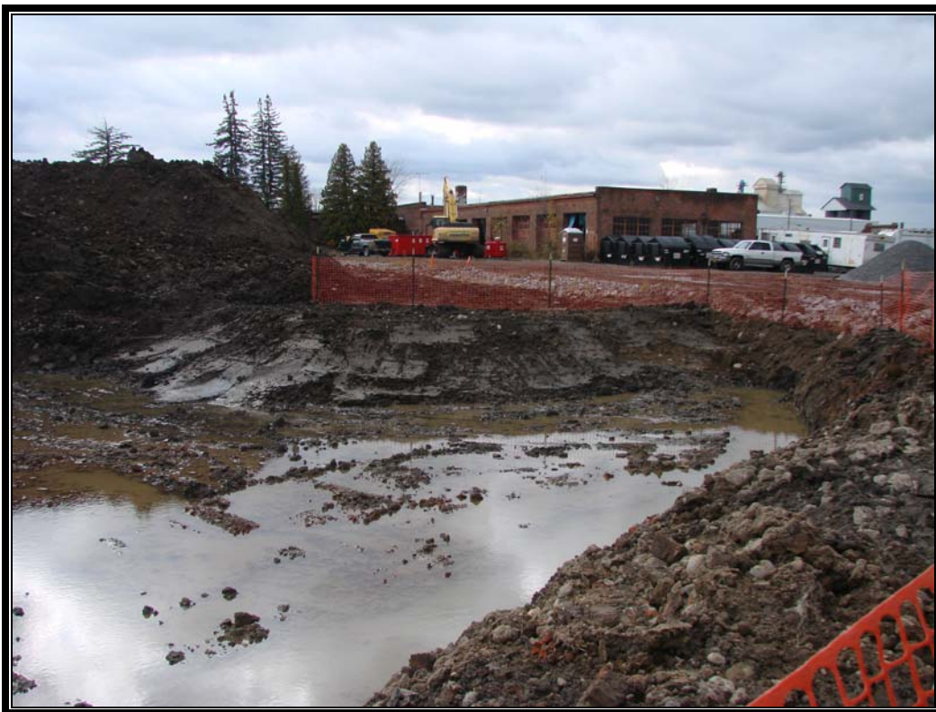
Photo #28: October 21, 2011 –Phase I: Completion of Excavation 1, to ~5 to 5.5 feet below grade (fbg), in the northwest corner of the excavation.
