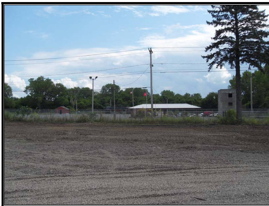
Photo #99: August 20, 2012 –Phase II: Final restoration and grading.
