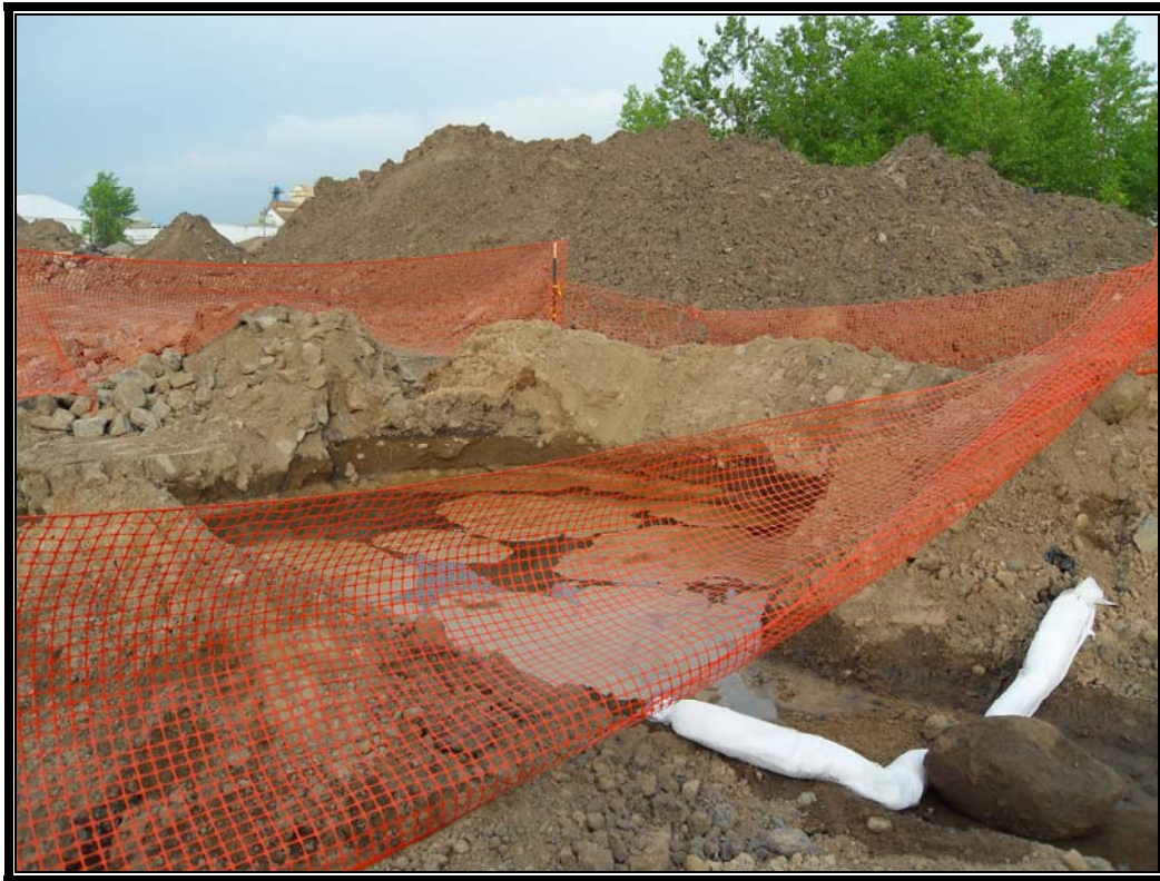
Photo #71: June 8, 2012 –Phase II: Dewatering activities. Water flows into this filtration pond, overflow passes thru 2 nd boom and into the onsite drainage trench.
