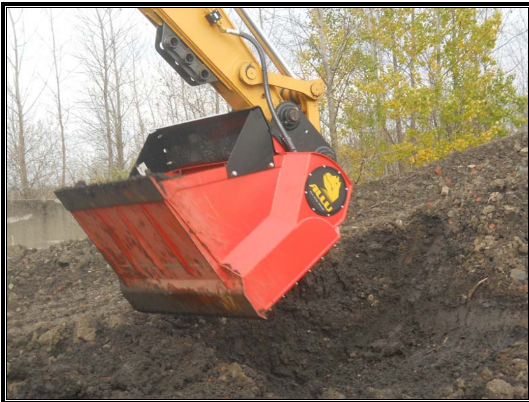
Photo #24: October 19, 2011 – Beginning of Phase II: Aeration of Windrow 1 via Allu excavator.
