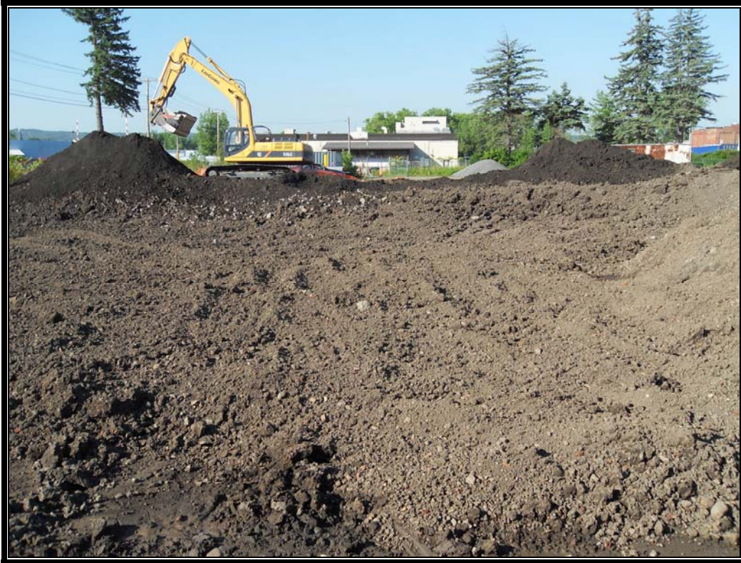
Photo #77: June 28, 2012 – Phase II: Excavation 3 and 2 backfilled.
