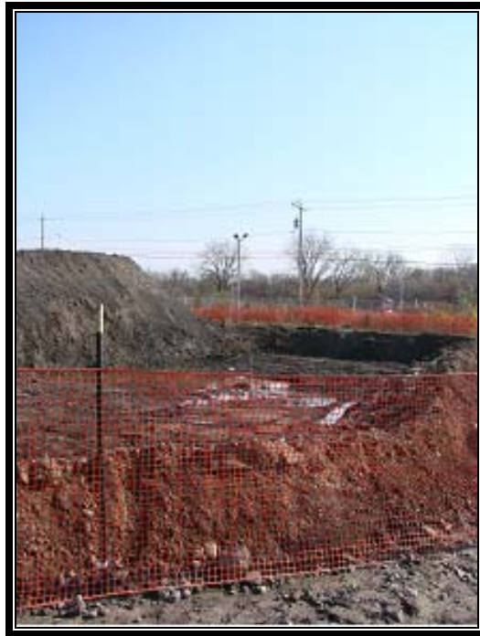
Photo #41: November 1, 2011 –Phase I: Completion of excavations and windows, winterization of site with orange snow fencing.
