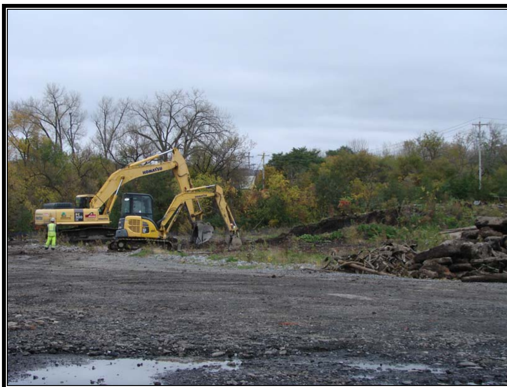
Photo #18: October 13, 2011 – Phase I: Excavating the 3 rd staged soil pile, excavated ~1062 yd 3 to date.
