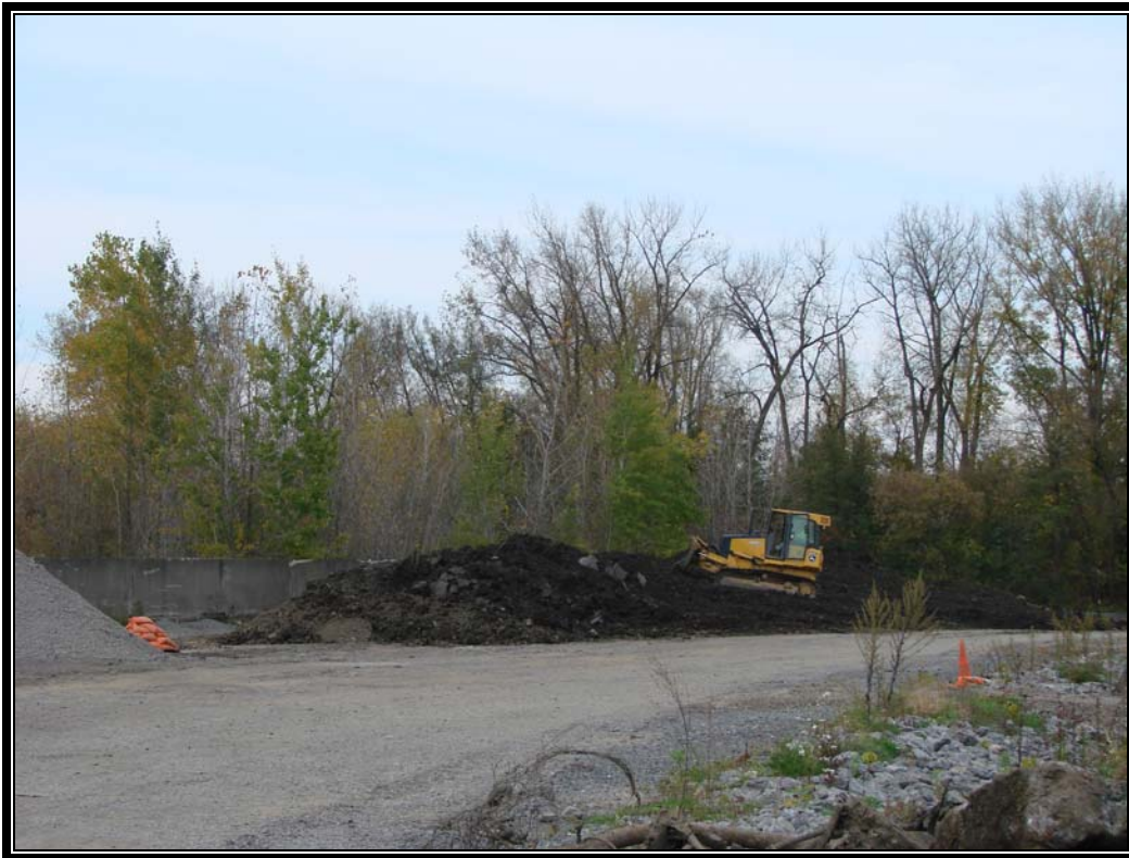
Photo #15: October 11, 2011 – Phase I: Shaping new Windrow 1.
