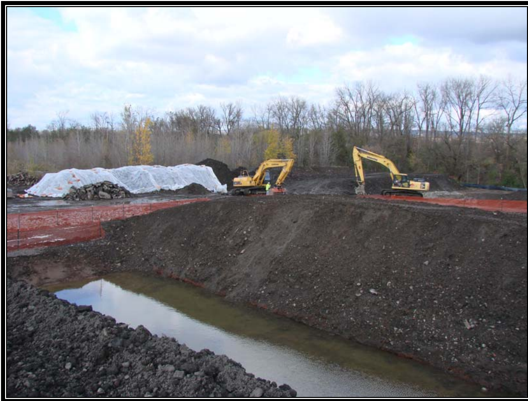
Photo #39: October 28, 2011 –Phase I: Completion of dressing Windrow 4, covering Allu soil pile 1 and dressing Windrows 1 and 2.
