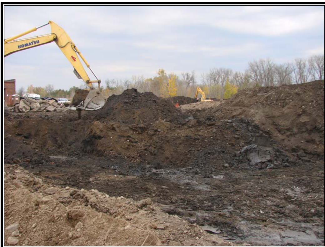
Photo #34: October 24, 2011 –Phase I: Continuation of Excavation 3.
