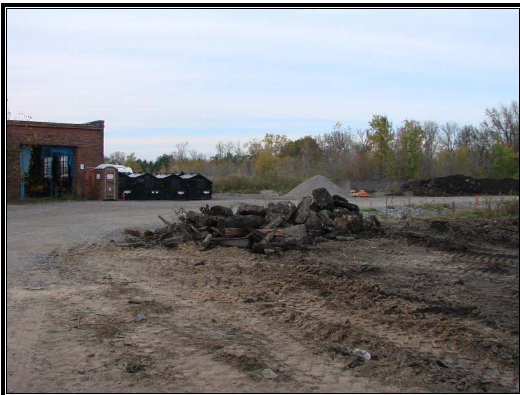
Photo #14: October 11, 2011 – Phase I: Separating out large debris and concrete.
