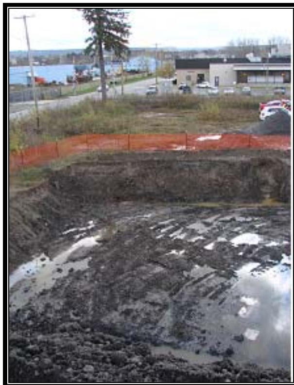
Photo #36: October 28, 2011 –Phase I: Completion of Excavation 3, ~4.5 to 5 fbg.
