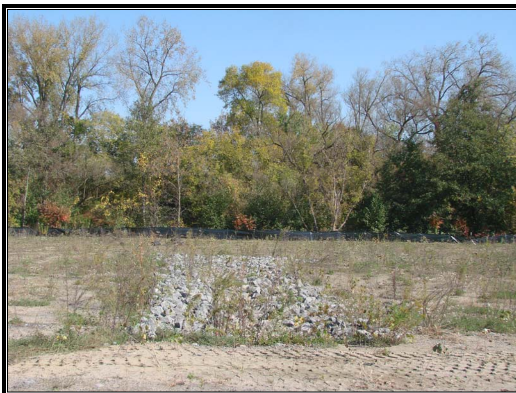
Photo #8: October 10, 2011 – Installation of silt fencing along northern property line.
