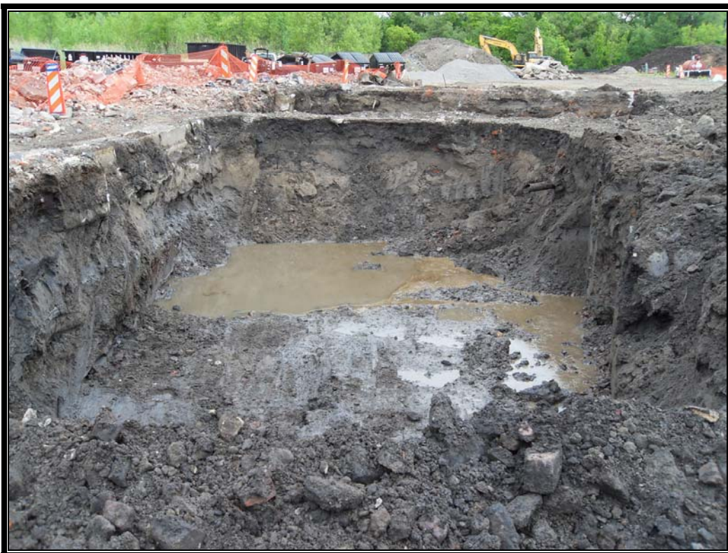
Photo #65: June 1, 2012 –Phase II: Continue excavation activities under the former building.
