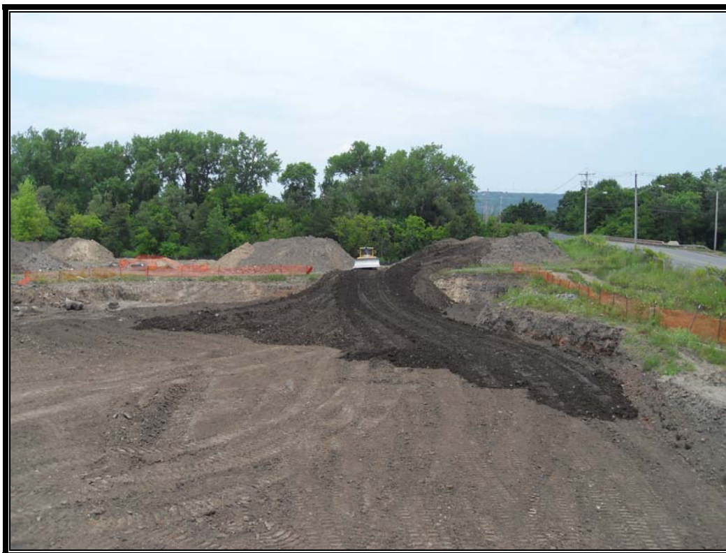
Photo #81: July 17, 2012 – Phase II: Backfilling excavation with dozer.
