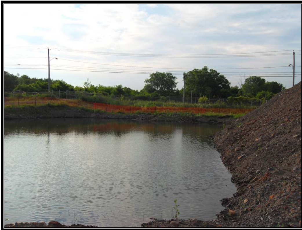
Photo #69: June 8, 2012 –Phase II: Dewatering activities. Settling pond in the SE corner of Excavation 1.
