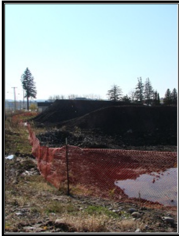
Photo #49: November 1, 2011 –Phase I: Completion of excavations and windrows, winterization of site with orange snow fencing.
