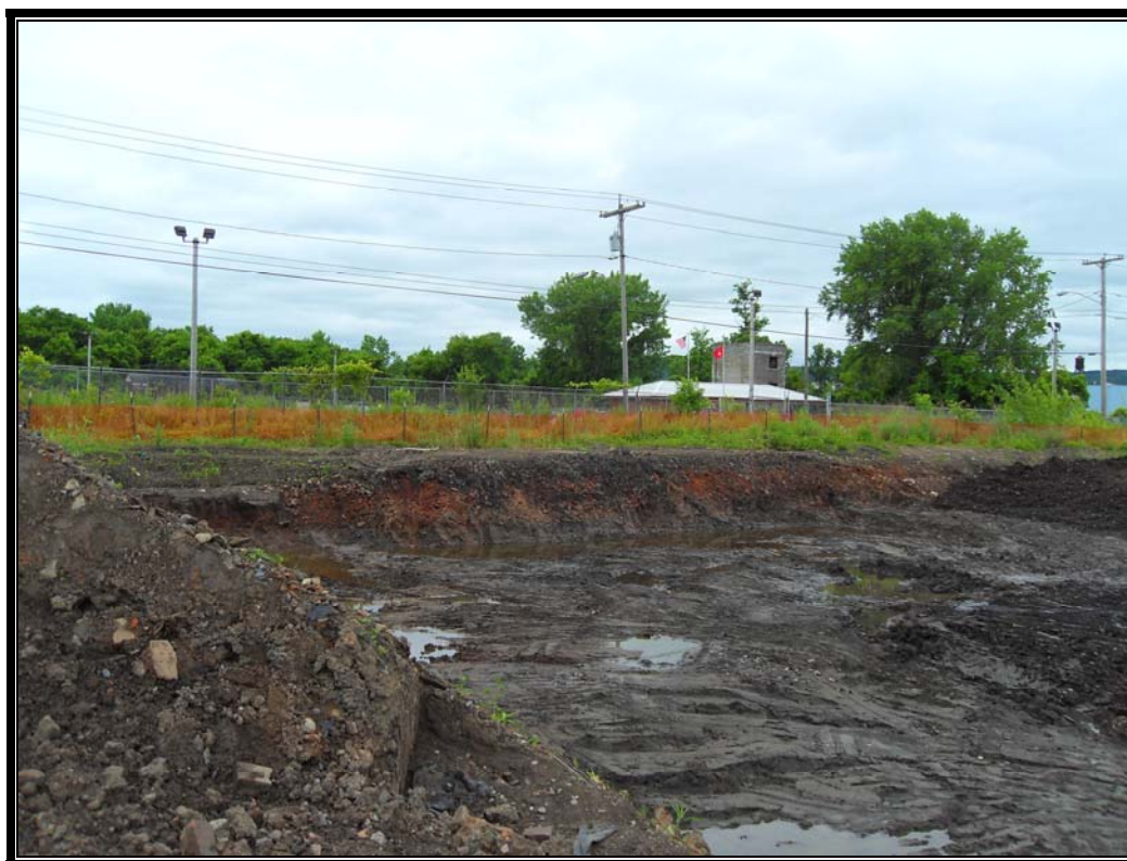
Photo #75: June 26, 2012 – Phase II: Started excavating within excavation 2.
