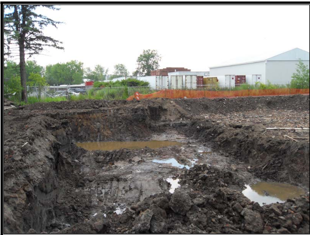
Photo #86: July 24, 2012 – Phase II: Excavation east of former building down to clay layer.
