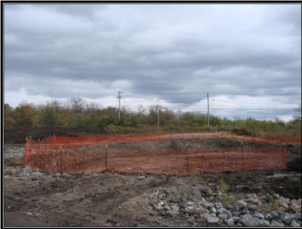
Photo #27: October 21, 2011 –Phase I: Completion of Excavation 1.
