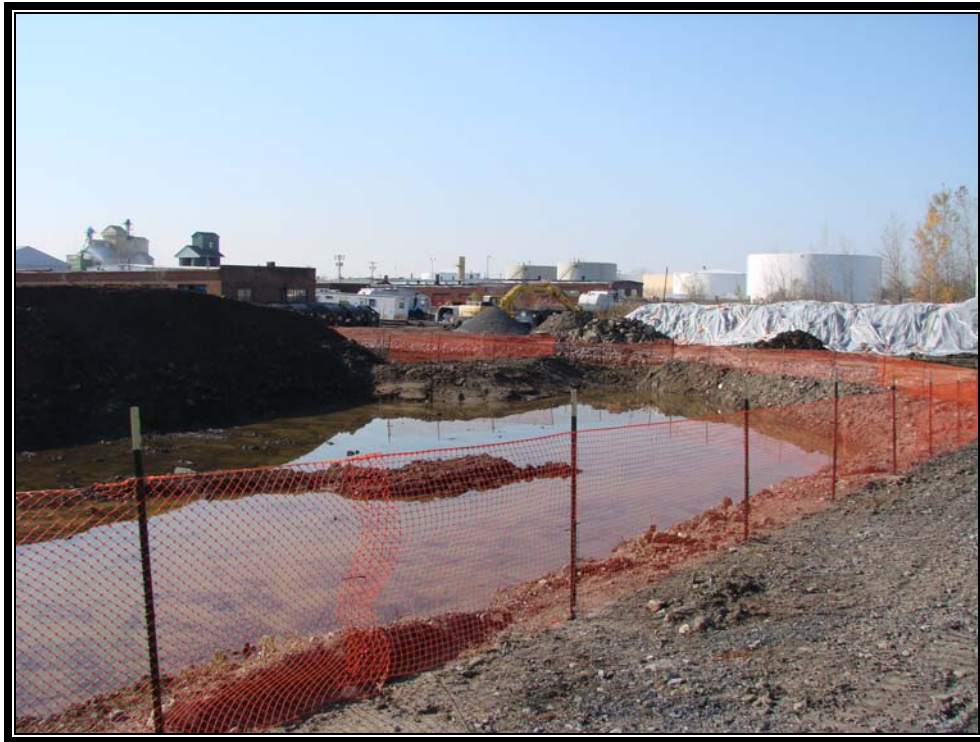
Photo #47: November 1, 2011 –Phase I: Completion of excavations and windows, winterization of site with orange snow fencing.
