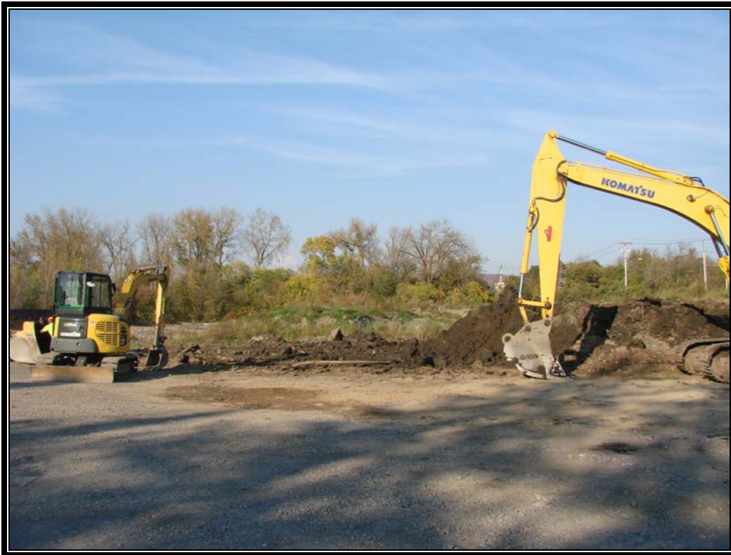
Photo #11: October 10, 2011 – Beginning Phase I: Moving staged soil to new windrows.
