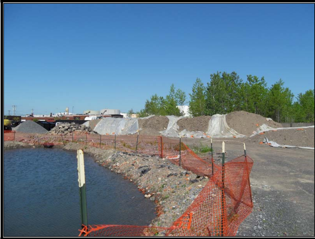
Photo #57: May 21, 2012 –Phase II: Removing plastic sheeting from 2011 winterization activities.
