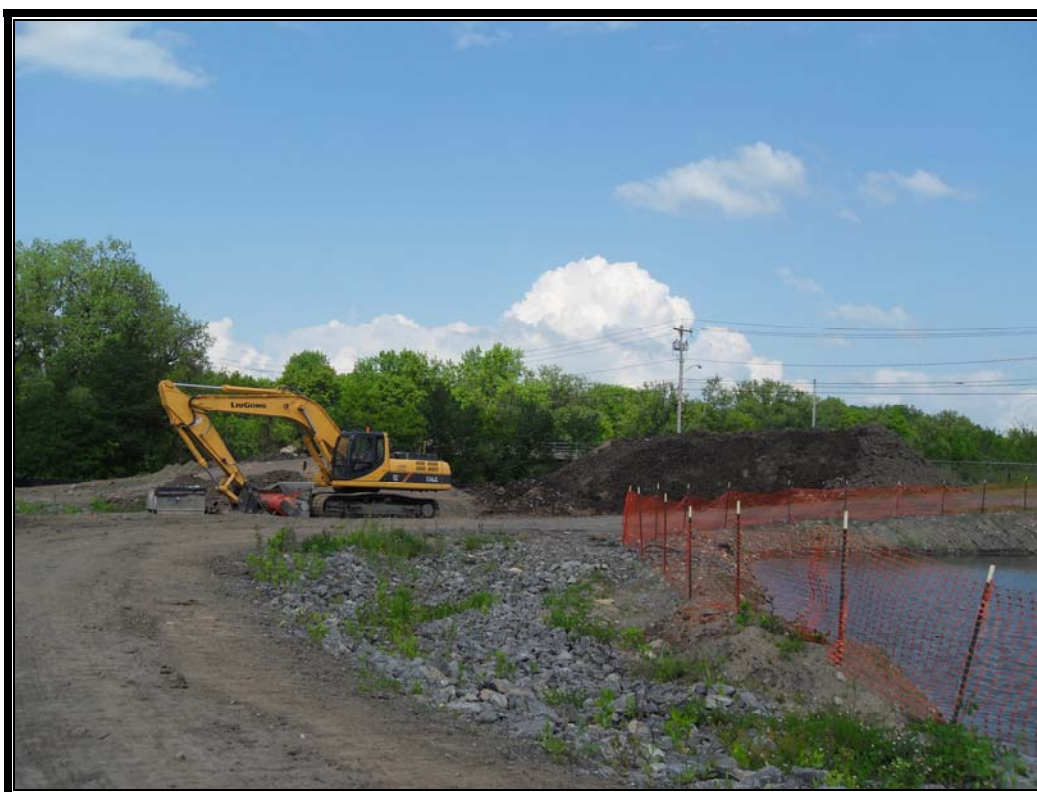
Photo #63: May 24, 2012 –Phase II: Continue alluing Windrow 3 into stockpile.
