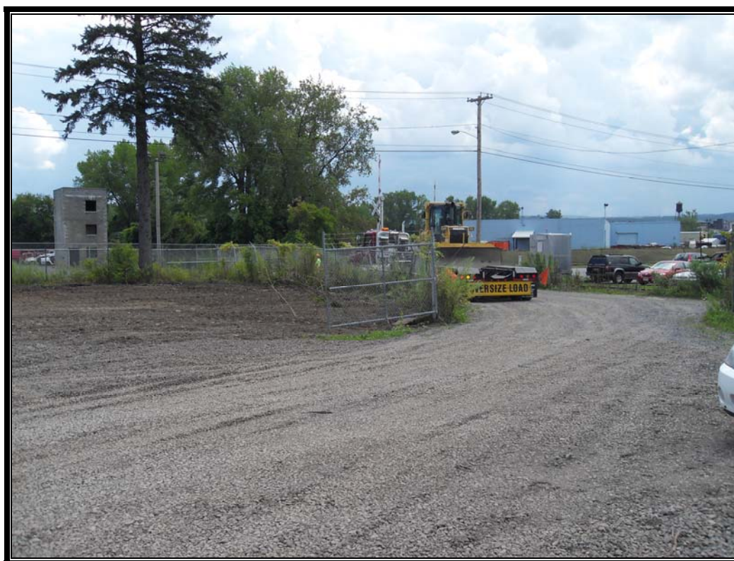
Photo #100: August 20, 2012 –Phase II: Final restoration and grading.
