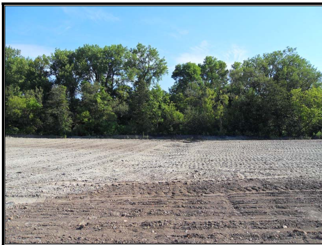
Photo #93: August 20, 2012 –Phase II: Final restoration and grading.
