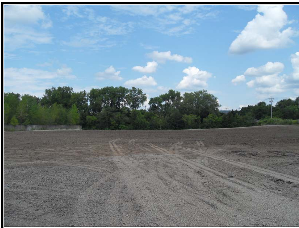
Photo #97: August 20, 2012 –Phase II: Final restoration and grading.
