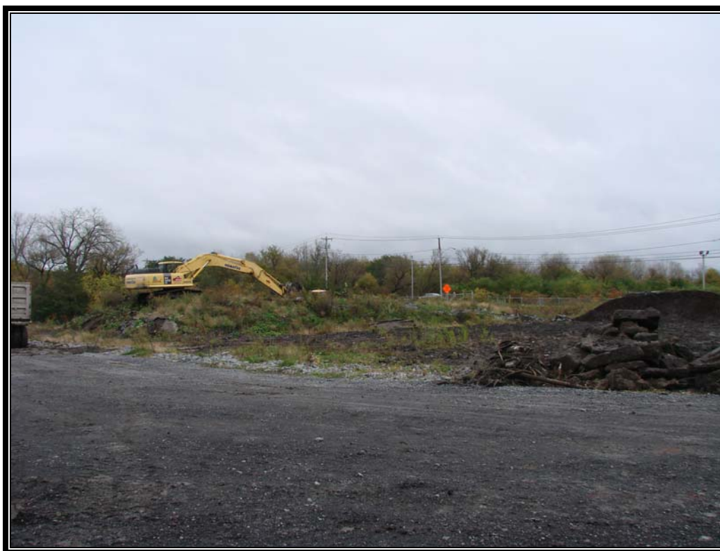
Photo #17: October 13, 2011 – Phase I: Excavating the 3 rd staged soil pile.
