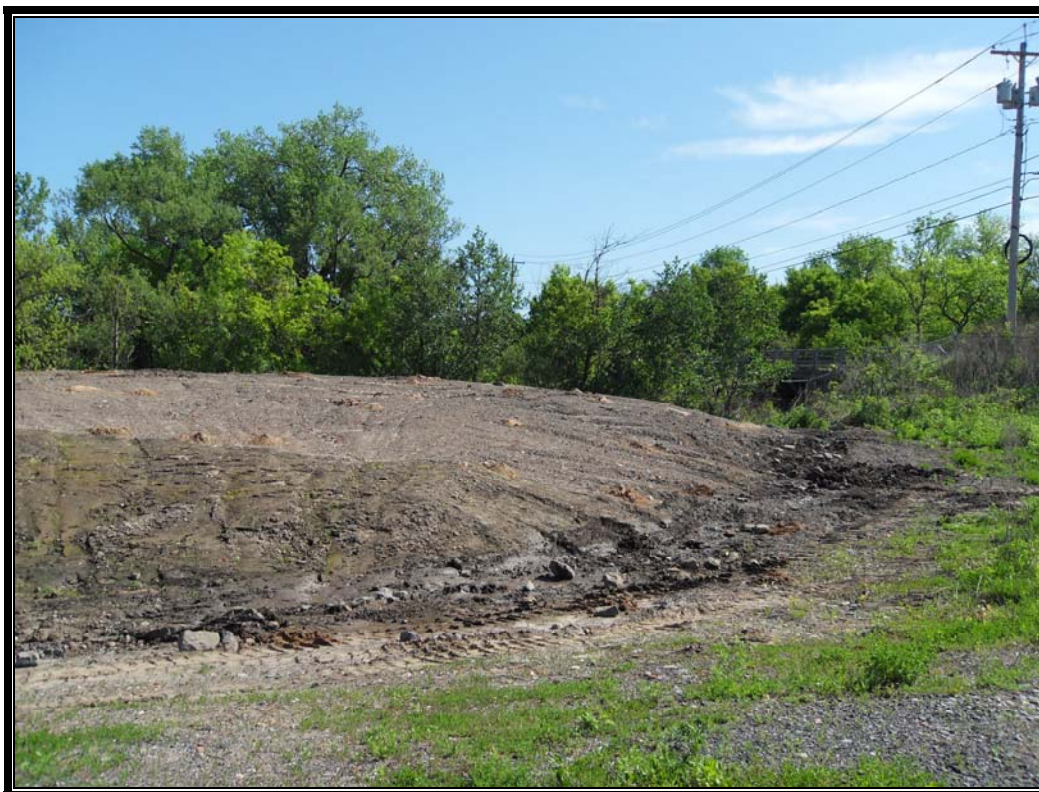
Photo #55: May 21, 2012 –Phase II: Removing plastic sheeting from 2011 winterization activities.
