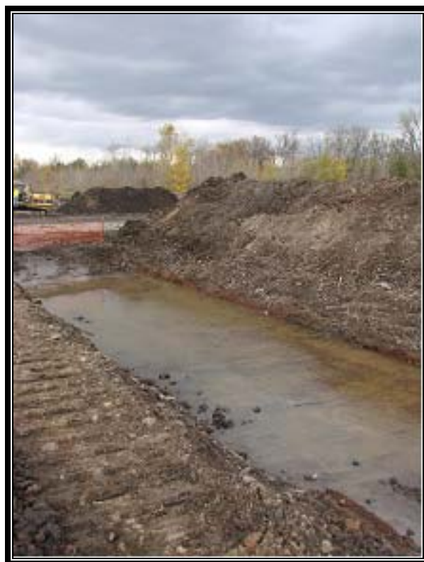
Photo #32: October 21, 2011 –Phase I: Completion of Excavation 2.
