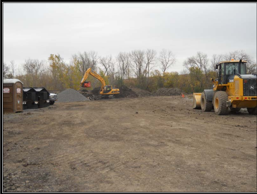
Photo #25: October 19, 2011 –Phase II: Aeration of Windrow 1 via Allu excavator.
