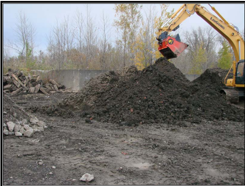
Photo #26: October 20, 2011 –Phase II: Aeration of Windrow 1 via Allu excavator.
