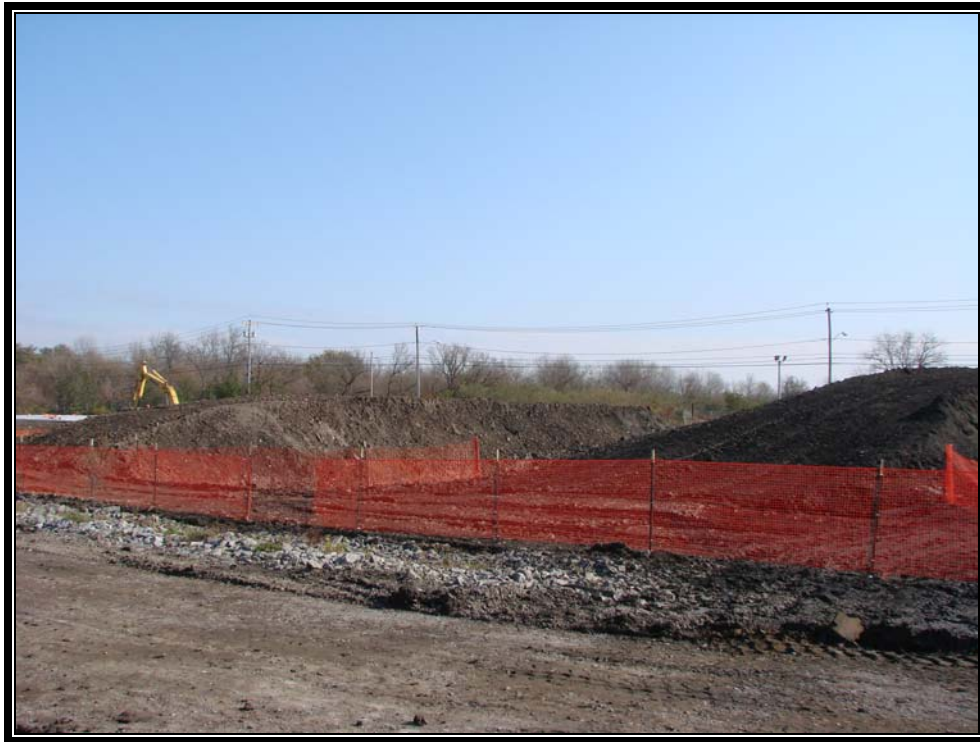
Photo #45: November 1, 2011 –Phase I: Completion of excavations and windows, winterization of site with orange snow fencing.
