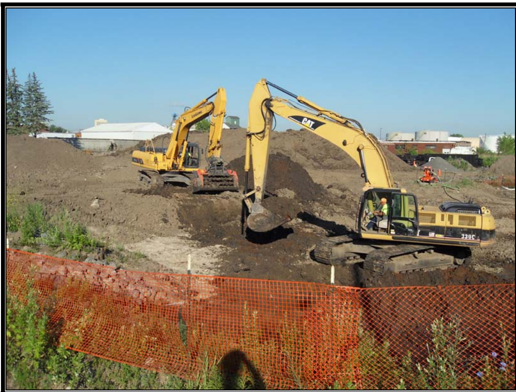
Photo #78: July 7, 2012 – Phase II: Started excavating excavation 1.
