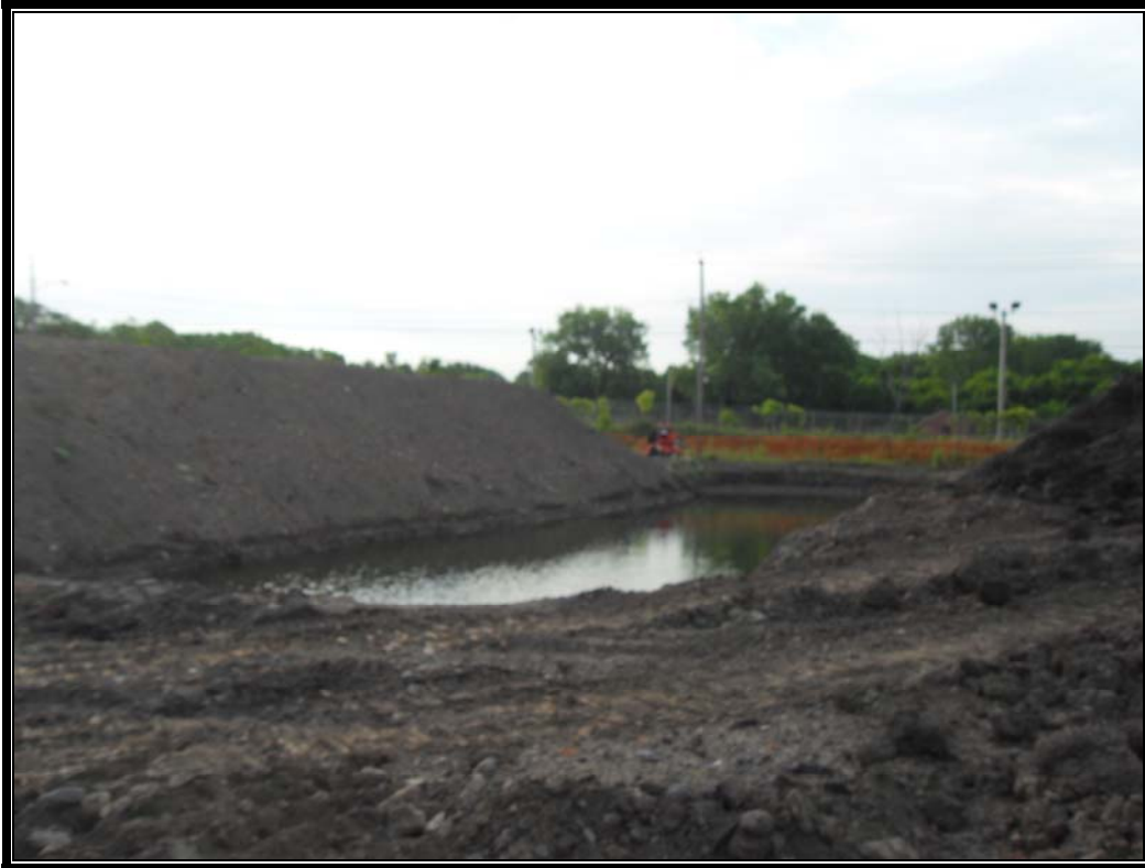
Photo #66: June 8, 2012 –Phase II: Start dewater activities. Pumping from Excavation 2 into Excavation 1.
