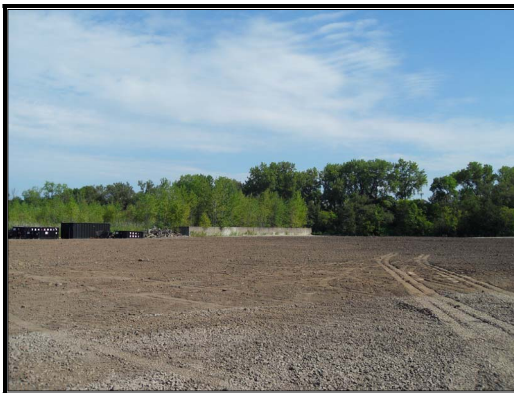
Photo #95: August 20, 2012 –Phase II: Final restoration and grading.
