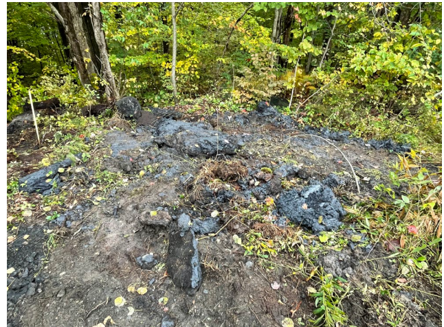
Photo 10: Backfilled test pit E3. Creosote visible on ground surface.
