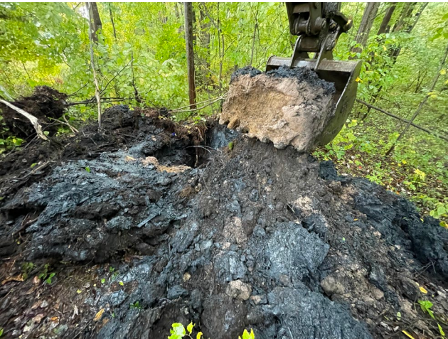
Photo 3: Surficial creosote in test pit E11.
