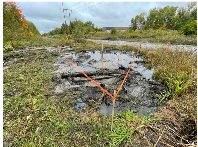
Photo 12: Backfilled test pit.
