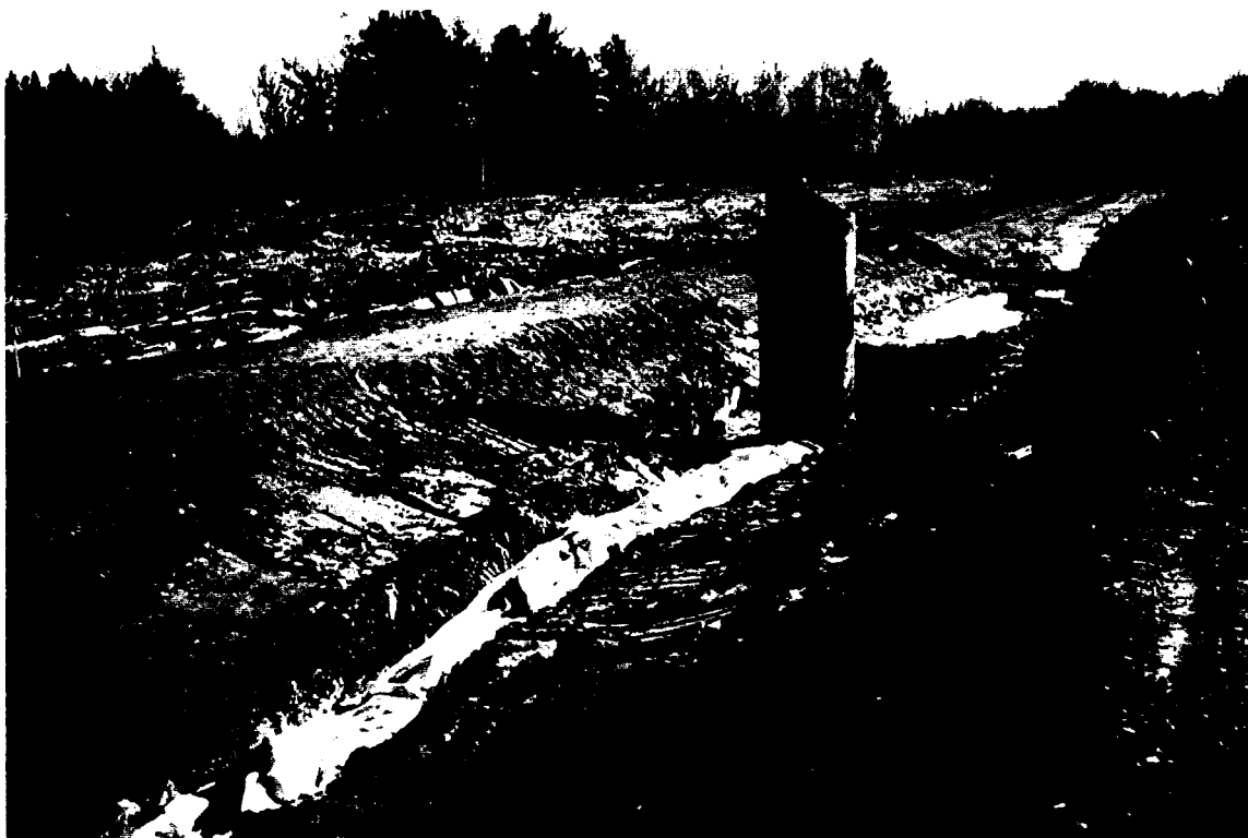
Photo Number 923 Date: May 16, 1995 Work Area: Landfill Description: Leachate collection trench with perforated pipe, drainage stone, filter fabric, and monitoring manhole (MH-602) installed. Wetlands "stressed area" prior to final remediation at left. Clay dike between Landfill and Wetlands.
