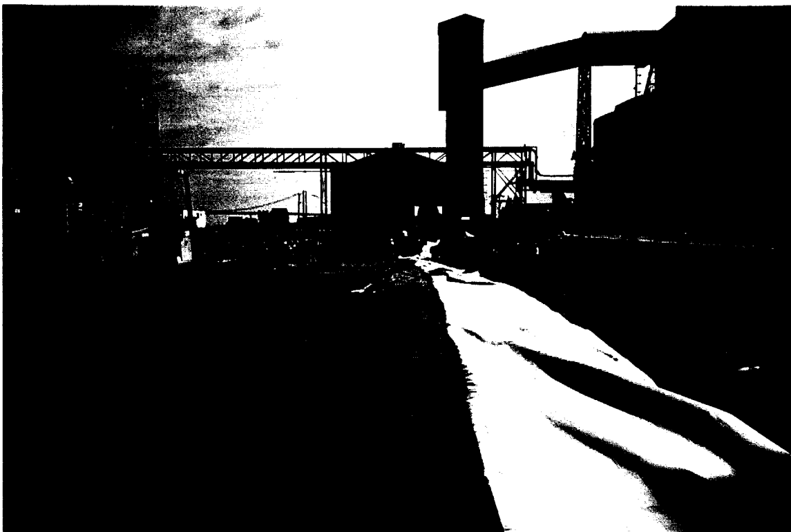
Photo Number: 1010 Date: September 3, 1995 Work Area: North Yard Description: Restoration of the busy rail yard, including grading the cured flowable fill and installing geotextile cushion and geomembrane liner. Note that the rail tracks are temporarily removed.
