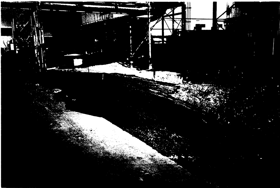
Photo Number: 1007 Date: August 30, 1995 Work Area: North Yard Description: Placing “flowable fill” near Carbon Plant Facility 22. This innovative, high-quality backfill material allowed critical remediation areas to be quickly returned to service.
