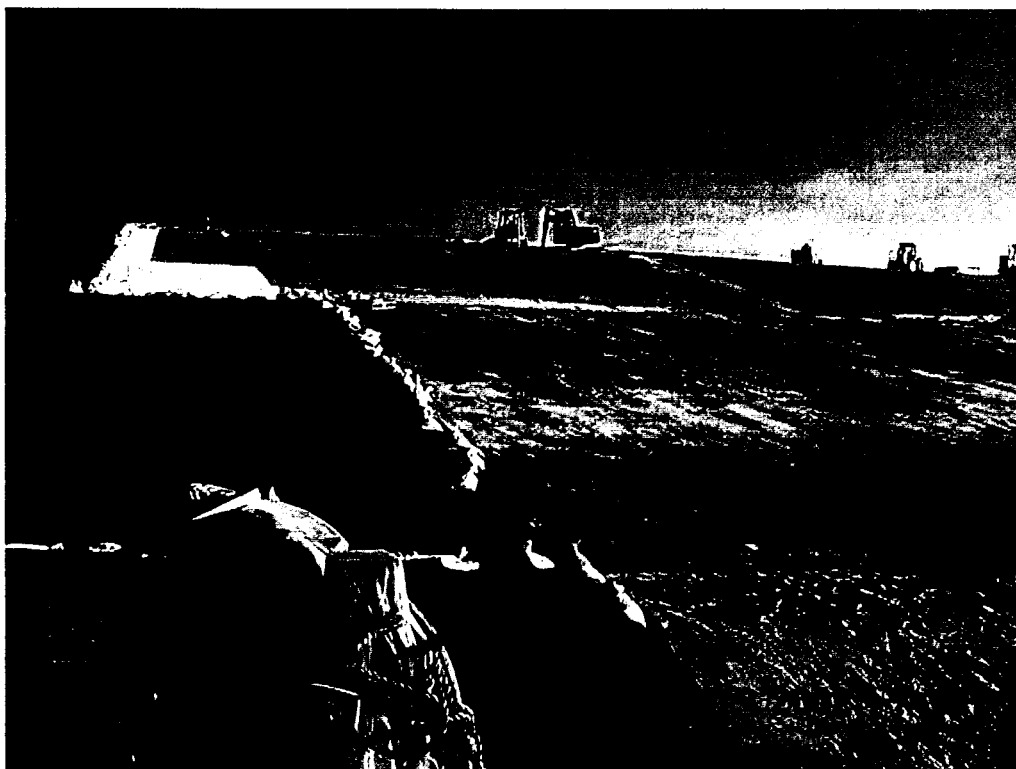
Photo Number: 1550 Date: July 31, 2002 Work Area: Landfill Description: Installation of RCRA cap. Prepared subgrade on the right. Geomembrane liner on the left. Horizontal benches on the slopes.
