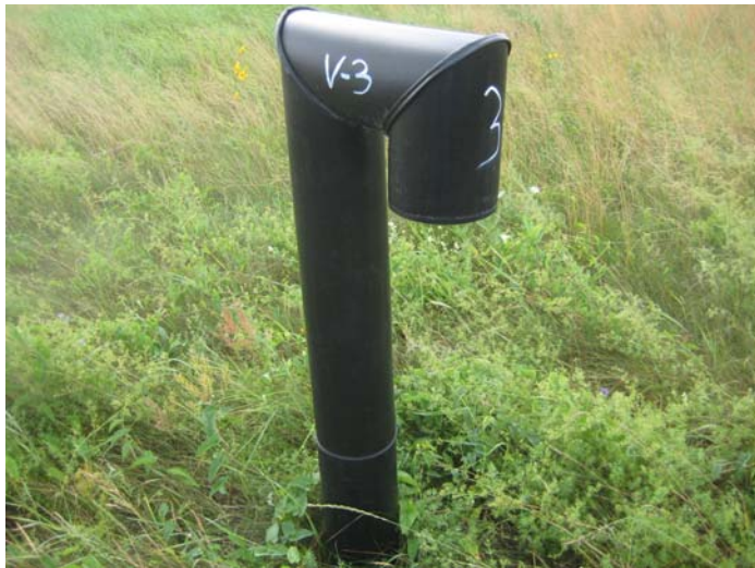
Disposal Cell Vent V-3
