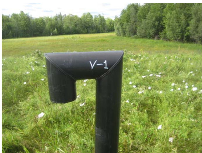
Disposal Cell Vent V-1
