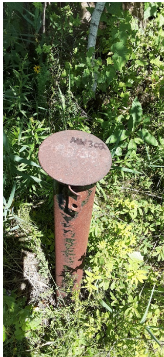
MW-302 Protective Casing
