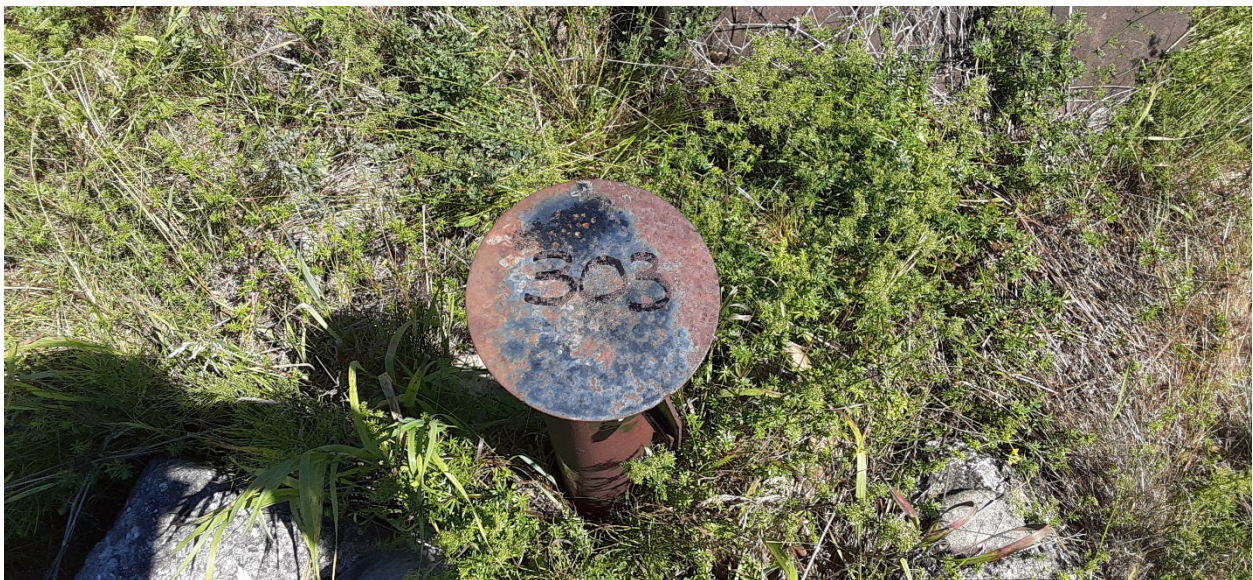
MW-303 Protective Casing
