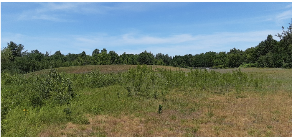
Fenced Disposal Cell Area Looking North
