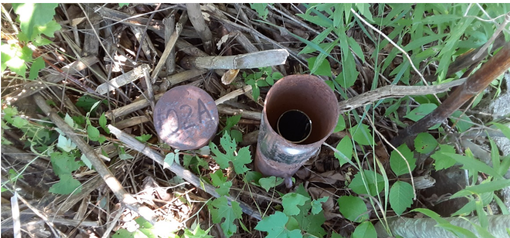
MW-102A Protective Casing and Monitoring Well
