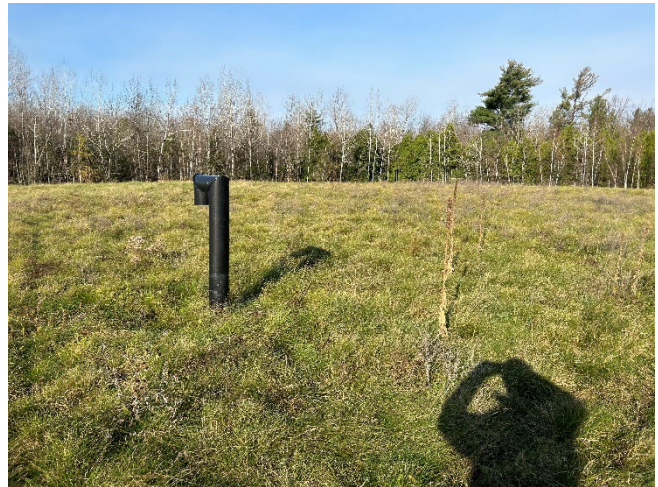
Top of landfill cap with gooseneck before mowing
