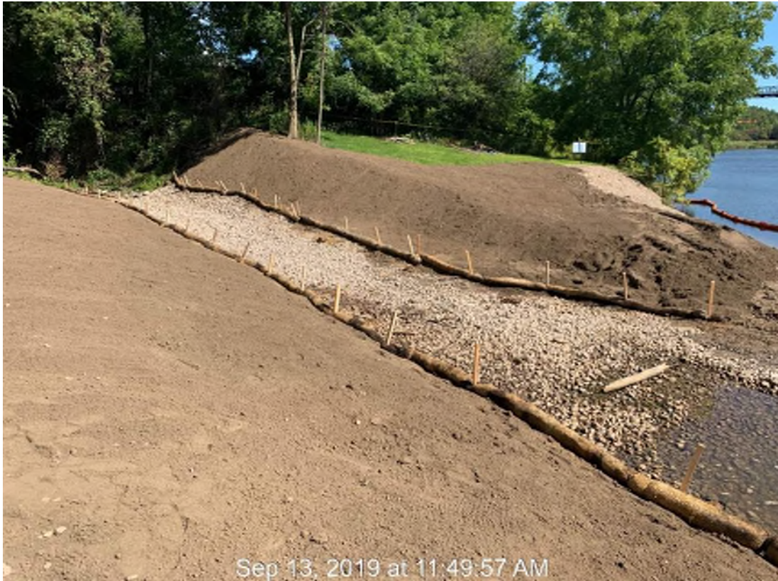
Looking North/East: Topsoil In Place and Graded
