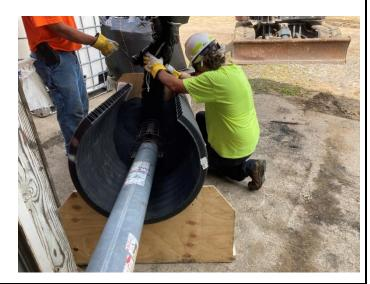
PHOTOGRAPH 24: NRC workers loading carbon from a super sack suspended by an excavator, into a tube auger for elevation of the carbon into the carbon vessel.
