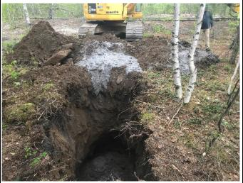
**PHOTOGRAPH 1:** Northerly view of test pit TP-4. Groundwater saturation resulted in cave-ins during the excavation process.
