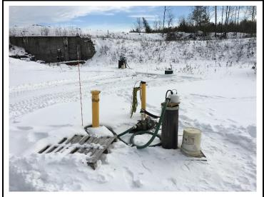
PHOTOGRAPH 5: Southern view of winter jet pump recovery well water depression operations. RW-2 in the foreground and RW-6 in the background.
