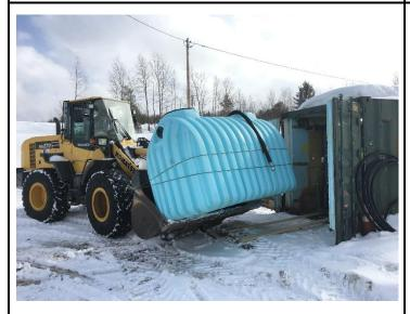
PHOTOGRAPH 15: Loading the new 1,150-gallon recovery well water transfer tank into the conex.
