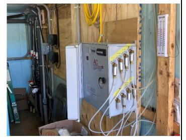
PHOTOGRAPH 21: AC Sipper Controller 2 installed in the groundwater depression pump controls conex building.
