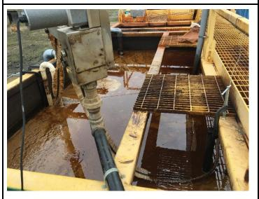
PHOTOGRAPH 19: April 28, 2021 view of water inlet chamber of weir, showing floating oil and emulsified oil. Ambar belt skimmer is operating in foreground.
