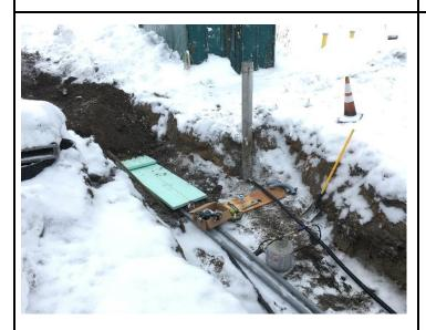
PHOTOGRAPH 11: RW-5 pitless adapter and water line installation. Waterline and conduits for RW-6 are also visible, coming from the left.
