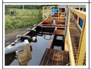
PHOTOGRAPH 27: September 8, 2021 photo of inlet chamber of weir. The photo shows dark free product introduced primarily by recovery trench pumping and vacuum truck skimming operations.
