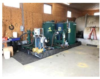
PHOTOGRAPH 2: View of groundwater treatment system components inside the Remediation Building, including water treatment pumps and control box, bag filter units, and activated carbon vessels. The 4,000-gallon oil storage AST and 18,000-gallon AST are visible.
