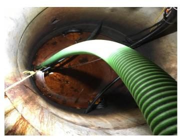
PHOTOGRAPH 4: View down the RTM-2 manhole, depicting vacuum truck oil skimming using a 2-inch vac hose.
