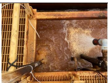
PHOTOGRAPH 4: Top view of central chamber of the weir tank, depicting the aeration blower/diffuser action, the pump sprayer nozzle, and chlorine injection tube.
