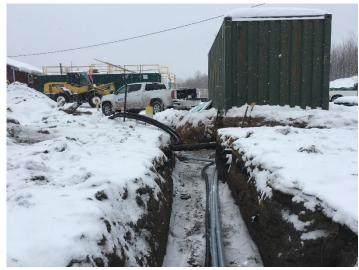
PHOTOGRAPH 10: East view of installation of RW-4 waterline and submersible pump power and AC Sipper air and oil line conduits.
