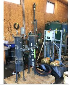
PHOTOGRAPH 20: Photo of additional parallel bag filter pair added for use of 1 micron bag filters to prevent iron precipitate from impacting the carbon vessels.
