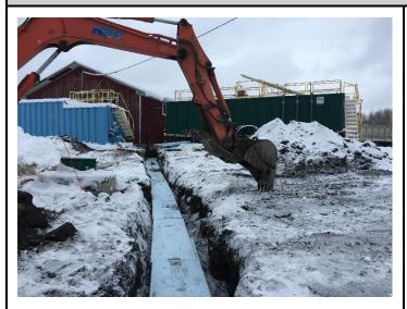
PHOTOGRAPH 9: Northeast view from pump controls conex to Remediation Building, showing installation of two layers of rigid insulation over the recovery well water transfer pipe.
