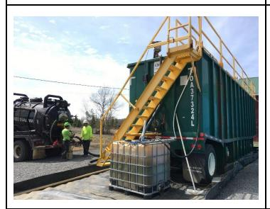
PHOTOGRAPH 3: View of vacuum truck recovery trench oil/water offloading operations. The weir tank oil recovery tote is in the foreground.
