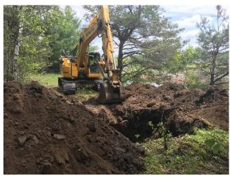
PHOTOGRAPH 2: Easterly view of TP-5, showing excavated sands and gravels with cobbles. The Little River is visible in the background.
