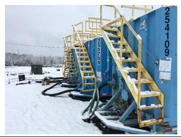
PHOTOGRAPH 17: Westerly view of newly reconnected hoses and initiation of frac tanks for oil/water and iron separation for the 2021 season. The Groundwater depression system pump controls conex building is visible in the background.
