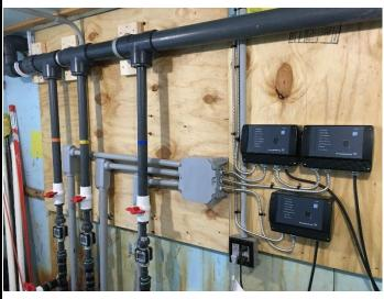
PHOTOGRAPH 14: Interior view of conex, showing submersible pump controllers, electrical conduits and incoming waterlines.
