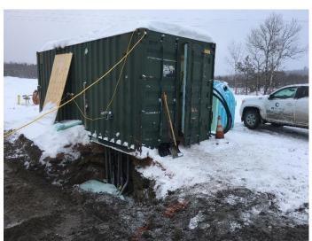
PHOTOGRAPH 12: Westerly view of pump controls conex, depicting waterlines and electrical supply and Sipper air and oil line conduits.
