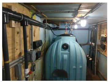
PHOTOGRAPH 16: View inside conex showing (left and right) recovery well waterlines, electrical conduits and pump control boxes.
