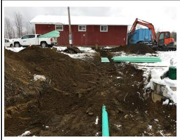
PHOTOGRAPH 7: Northerly view of new treated water discharge line from Remediation building to the Little River, during insulating and backfilling of excavated trench.
