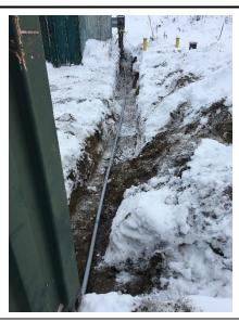
PHOTOGRAPH 8: Installation of new electrical supply line from existing pole and panel box to the groundwater pump controls conex building.
