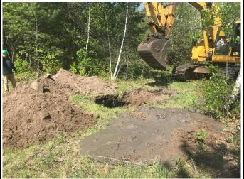
**PHOTOGRAPH 1:** Northwest view of test pit TP-3 upon contacting the groundwater saturation depth.
