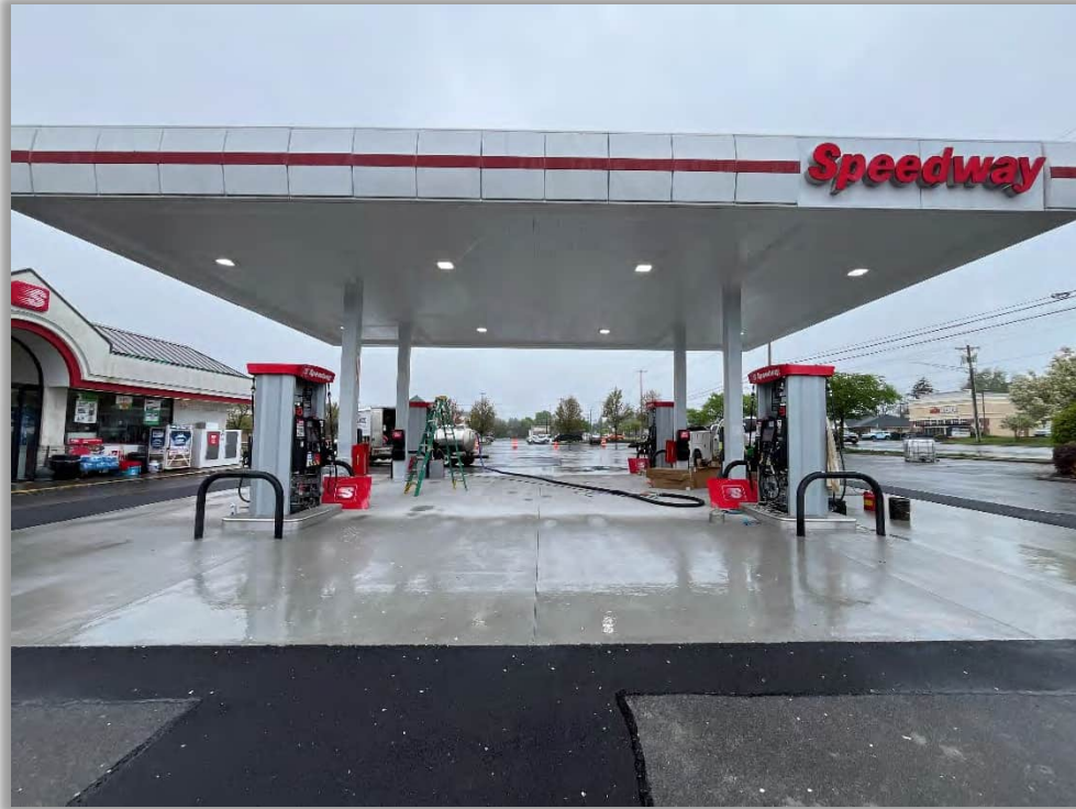
Photograph 13: New dispensers installed and canopy area after new concrete (looking west)
