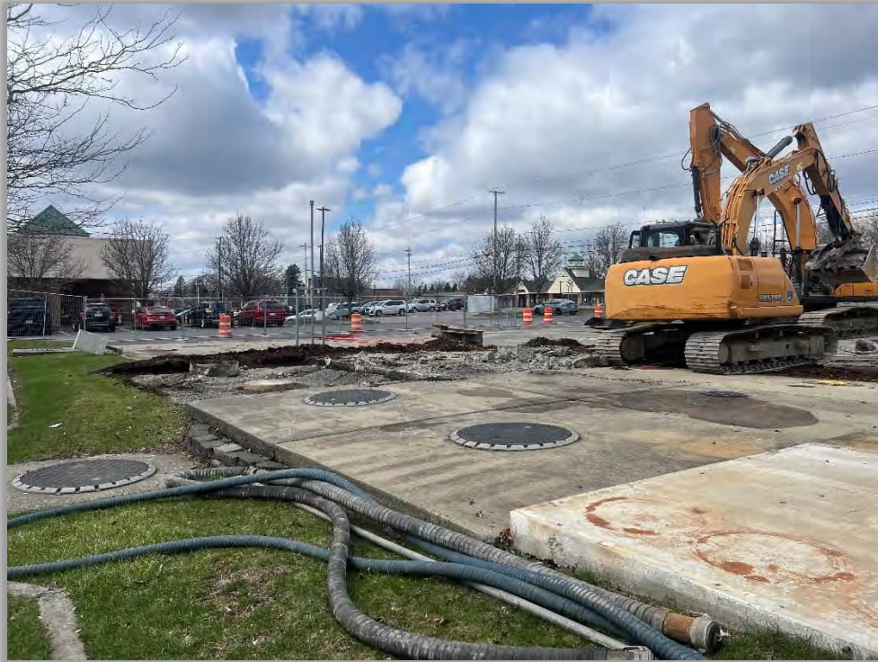
Photograph 1: Tank pad prior to removal activities (looking northwest)
