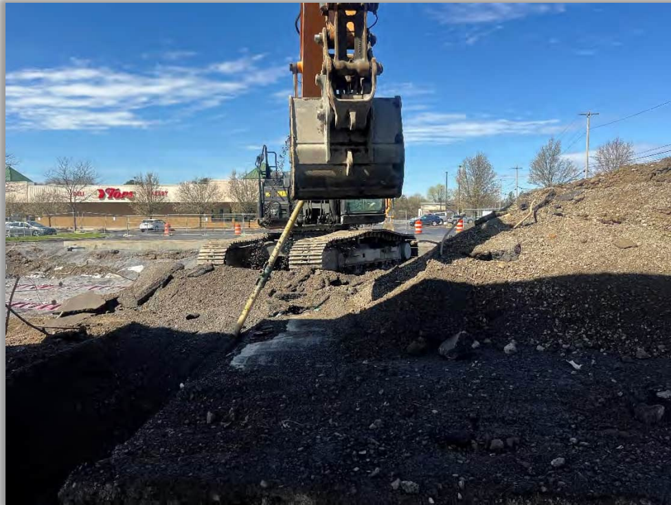
Photograph 12: Removal of old product piping during excavation (looking west)
