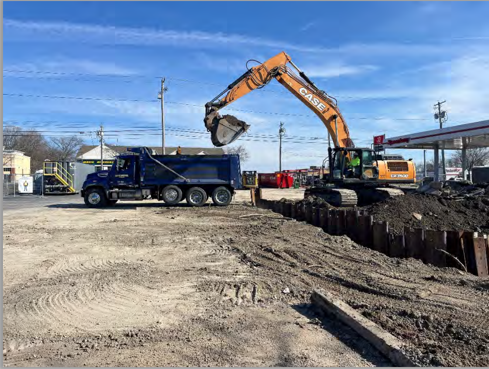
Photograph 7: Removal of soil from tank excavation (looking north)
