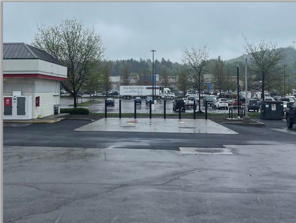
Photograph 14: New UST pad (looking south)
