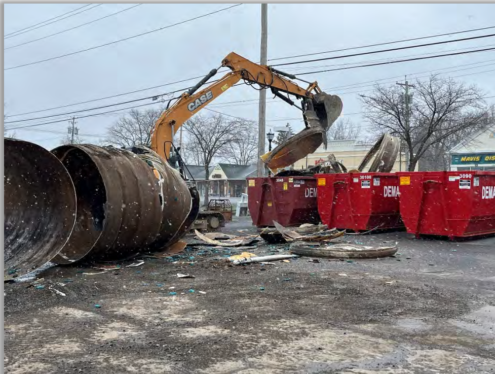
Photograph 6: UST being crushed into onsite roll-off dumpster (typical)
