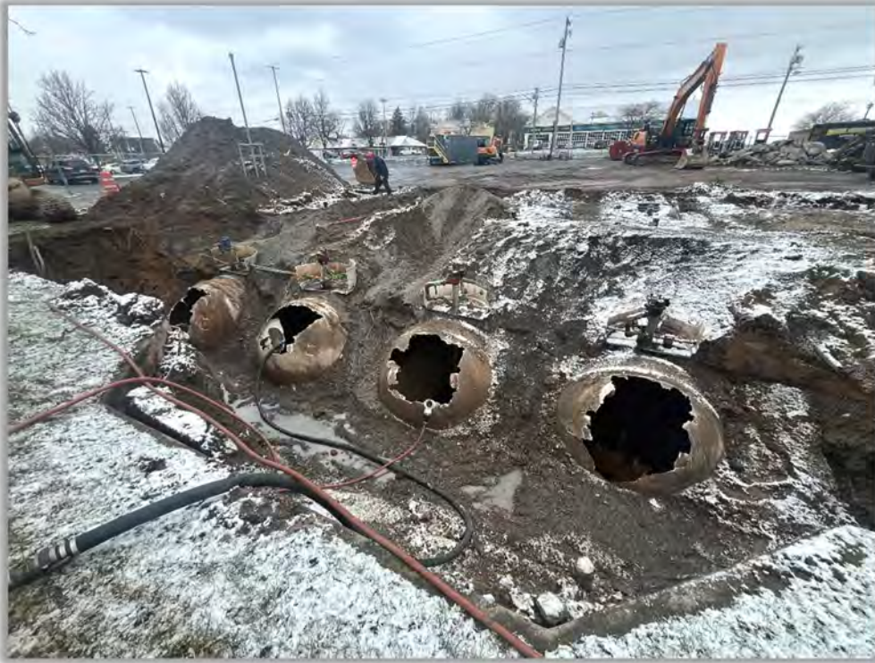
Photograph 3: Tanks exposed and opened for cleaning activities (looking northwest)
