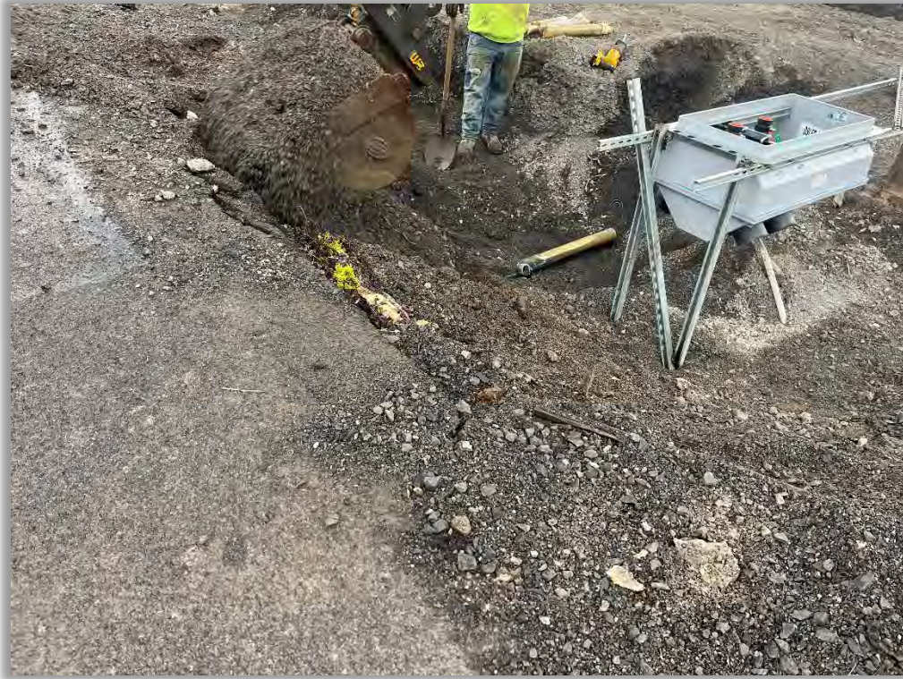
Photograph 11: Canopy area during excavation activities (looking northeast)
