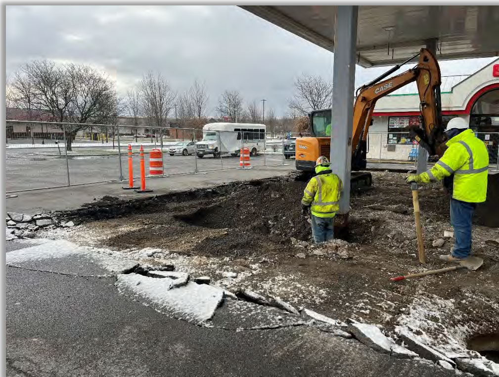
Photograph 10: Canopy area during excavation activities (looking southeast)
