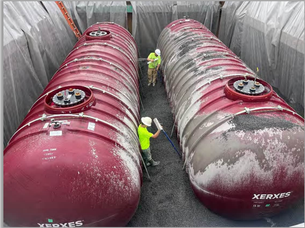
Photograph 9: New UST's during installation (looking south)
