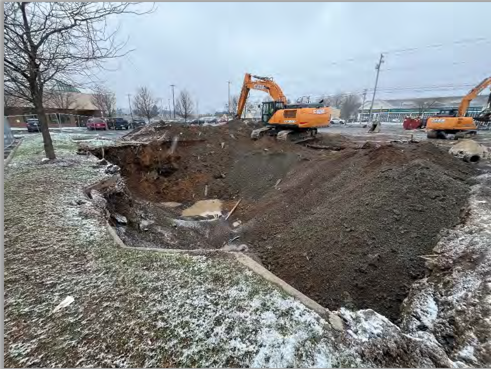
Photograph 5: Excavation following tank removal (looking west)
