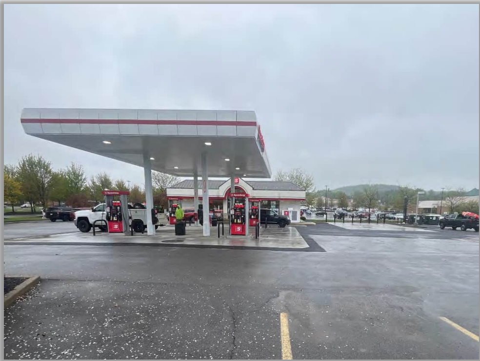
Photograph 16: Overall finished site photo (looking south)
