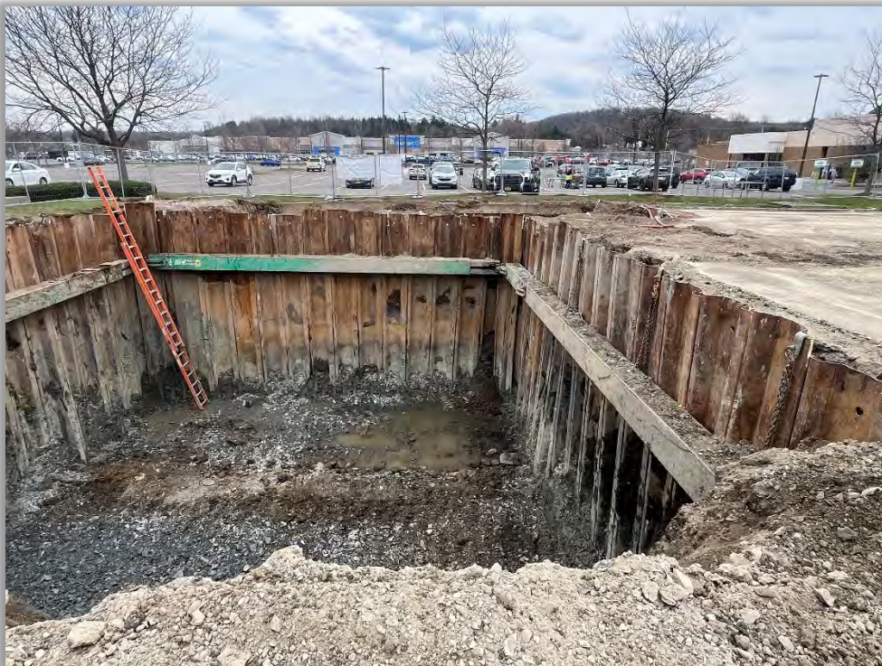
Photograph 8: Shoring installed in new tank hole (looking south)
