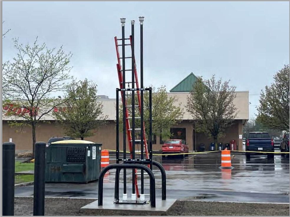
Photograph 15: New vent piping (looking west)
