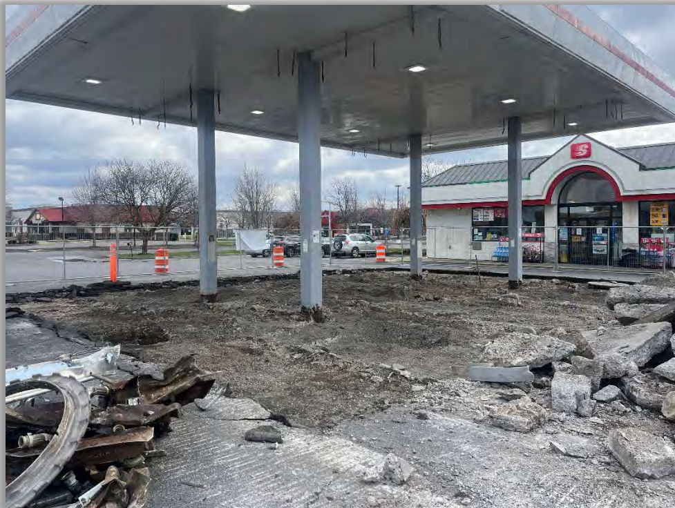
Photograph 2: Canopy Area during excavation activities (looking southeast)
