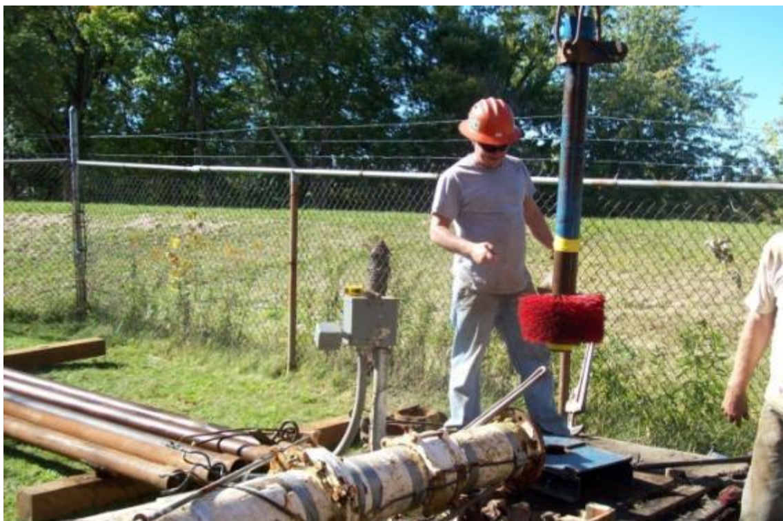
Photo 6: Wire brush assembly used to remove heavy buildup
