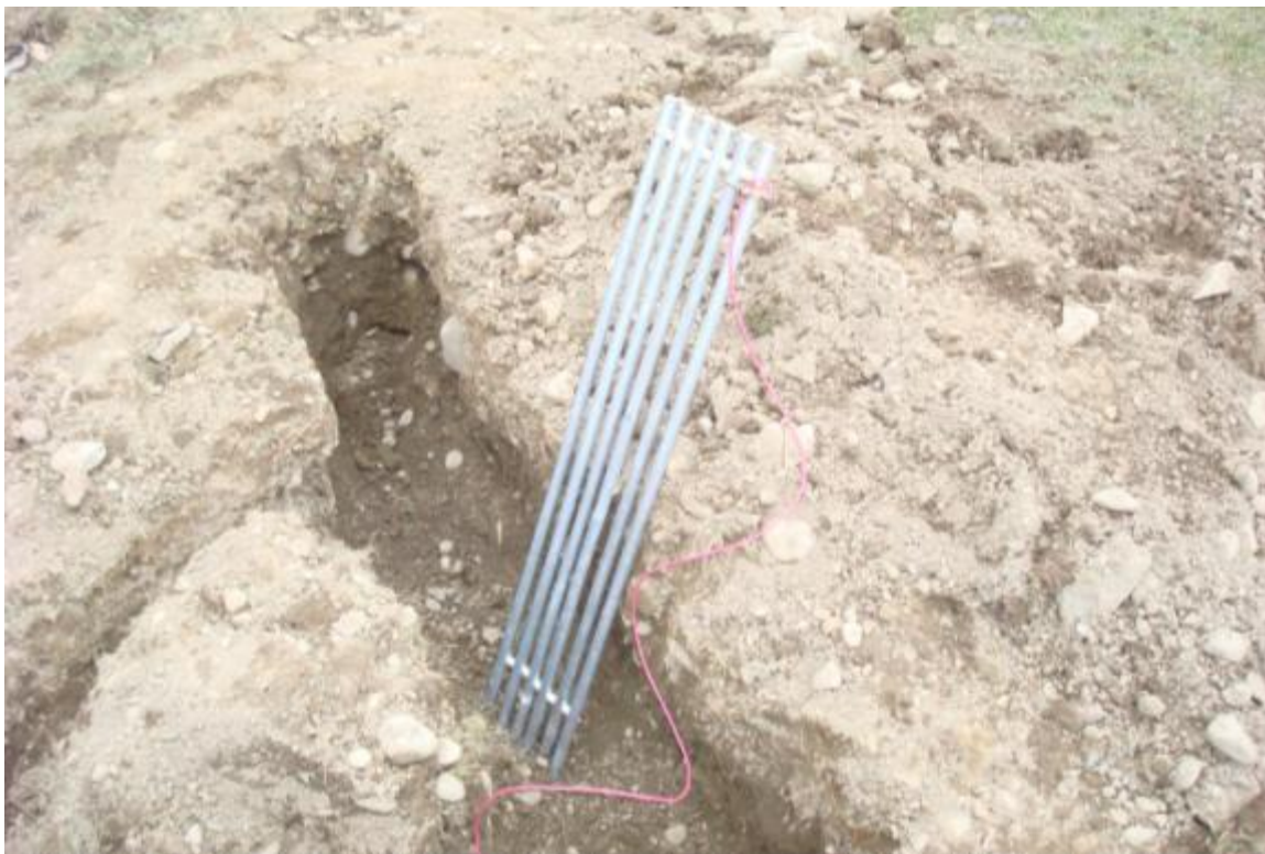
Photo 14: Caged-anode assembly
