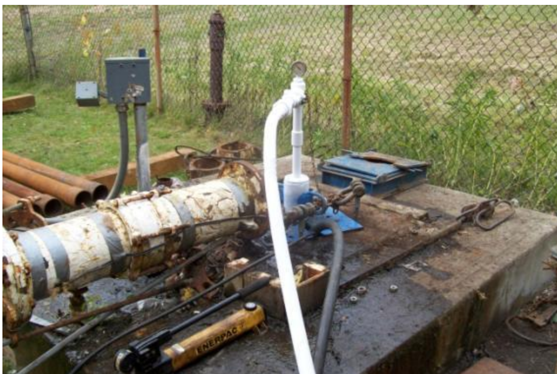
Photo 8: Aqua Freed® carbon dioxide injection
