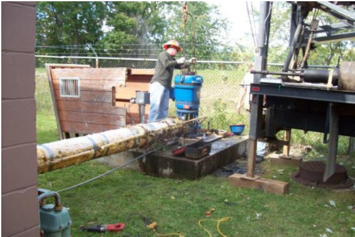
Photo 1: Removal of vertical line-shaft pump
