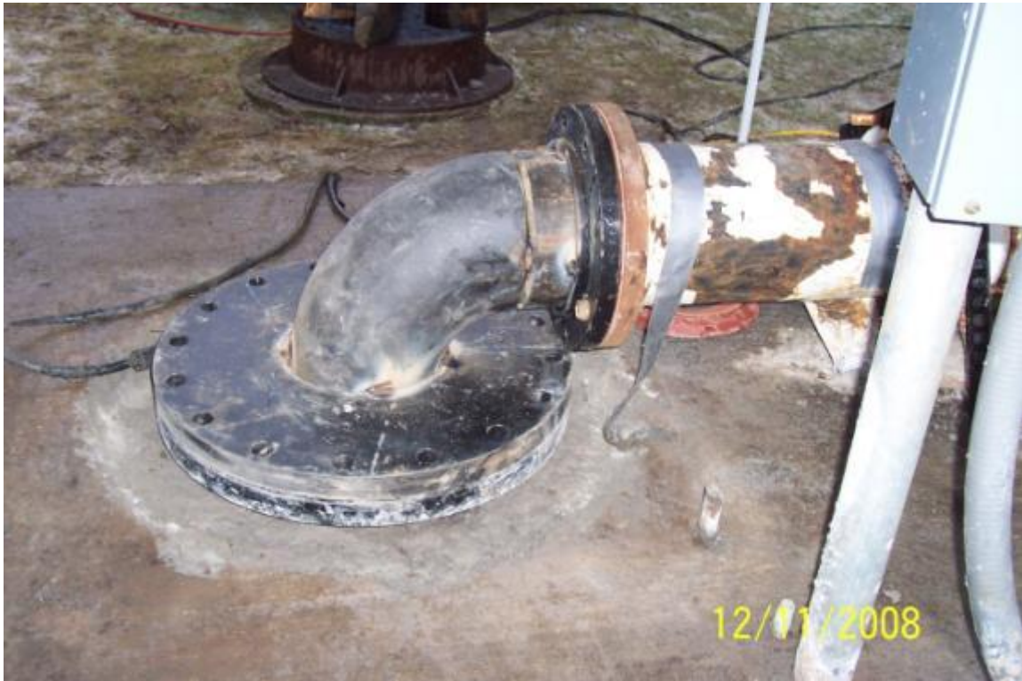
Photo 15: Fabrication of submersible pump discharge pipe
