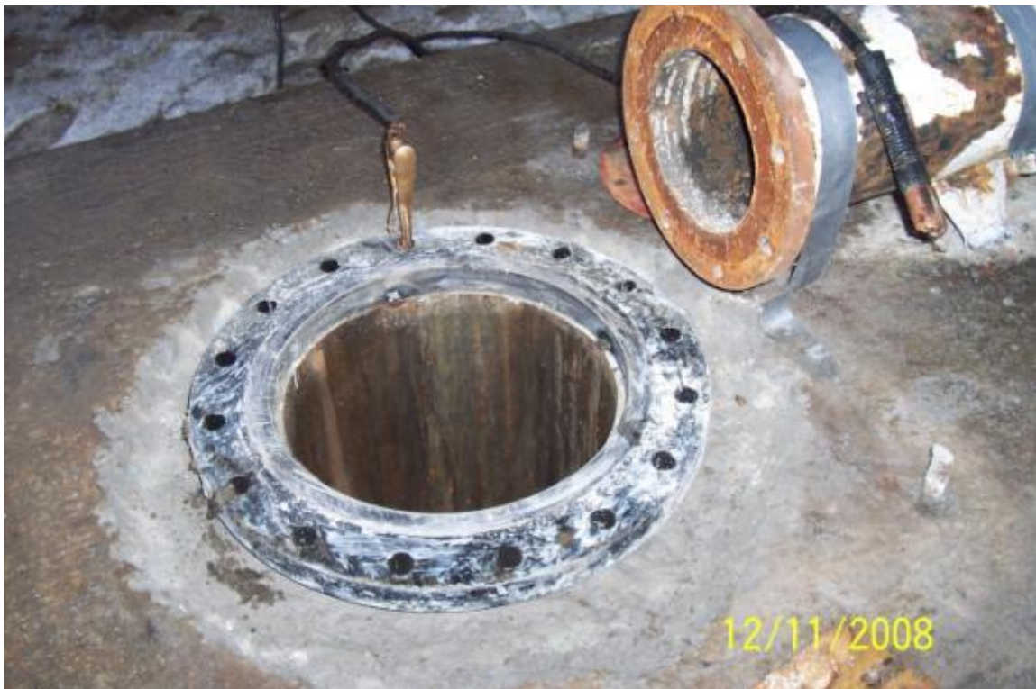
Photo 14: Companion flange being welded to well casing
