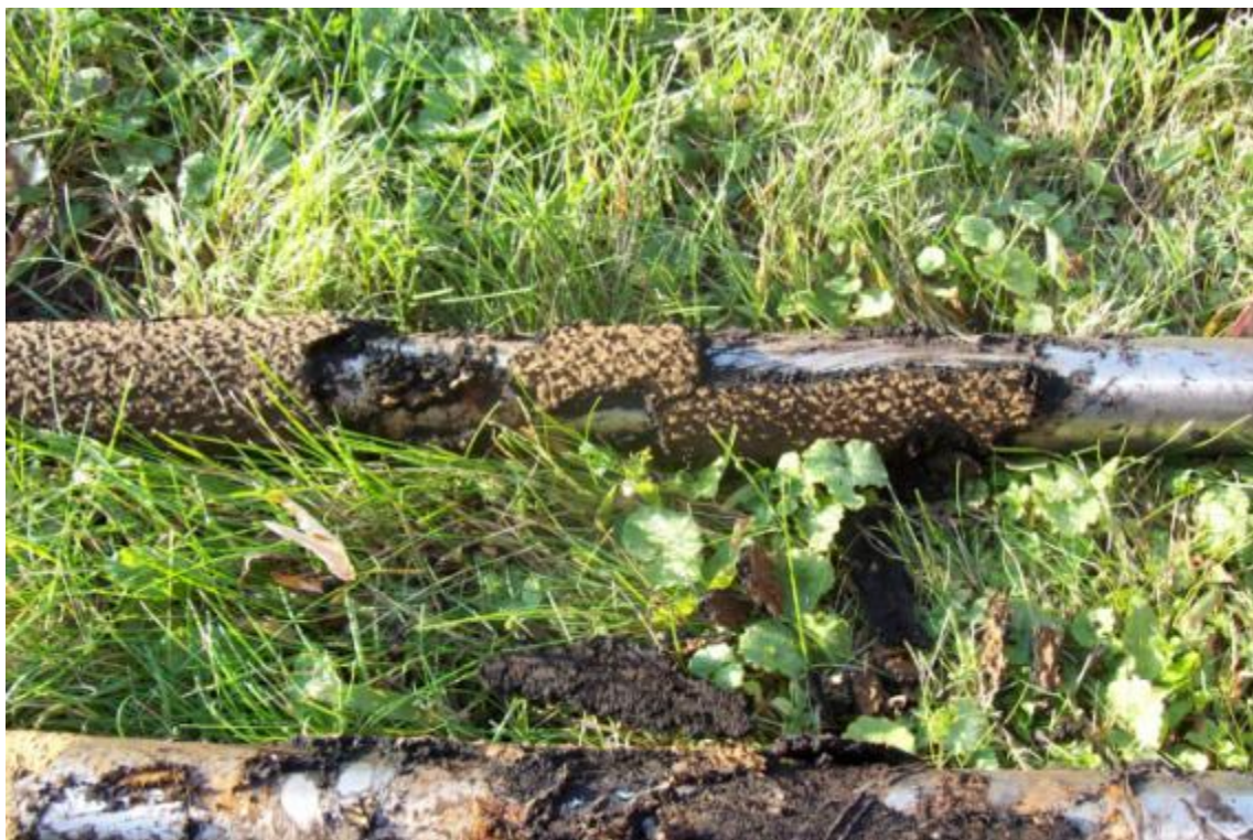
Photo 3: Deposits on line-shaft
