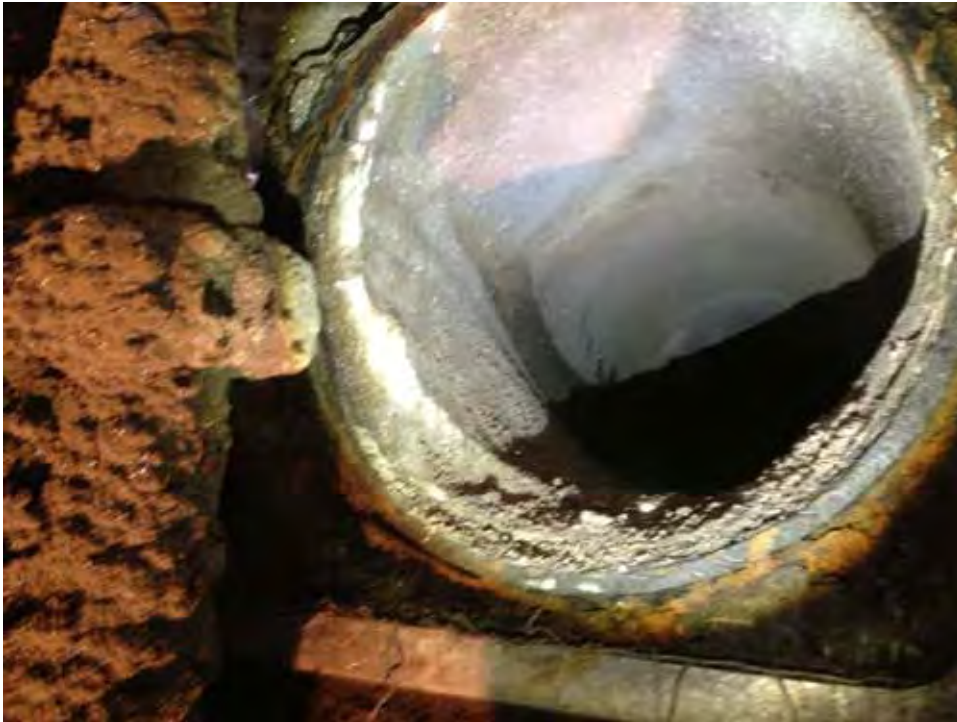
12" clear well outlet pipe following removal of obstruction..
