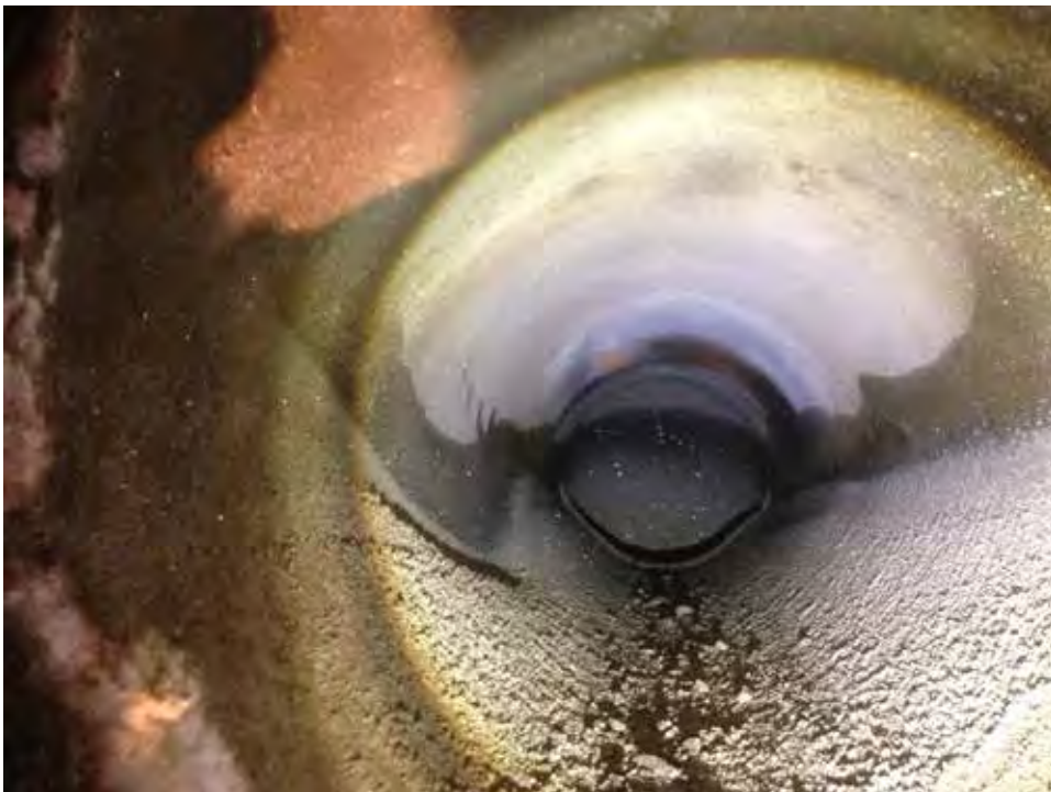
View of inside of 12" clear well outlet pipe.
