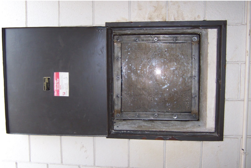
Air stripper tower access door with retaining screen and glass (photograph from 10/16/2006)
