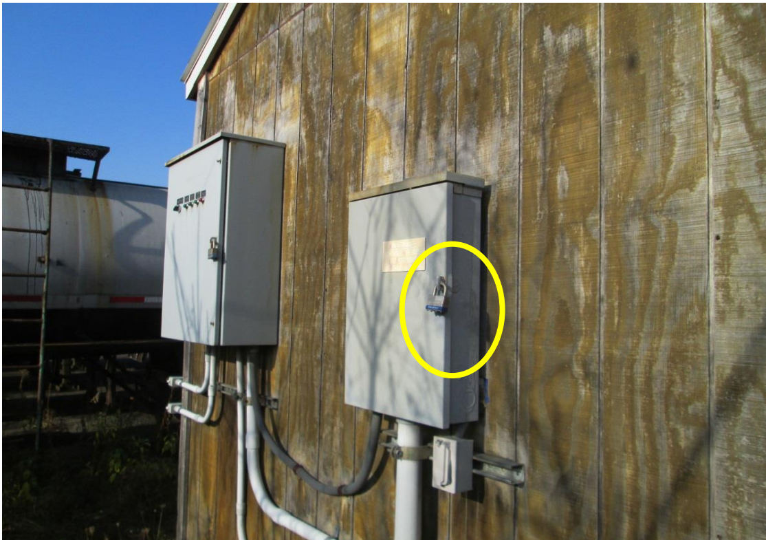
- Lock replaced on control panel
