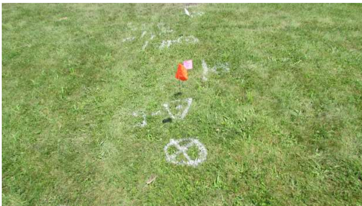
Additional field mark-outs verifying location, depth and angle of drill head
