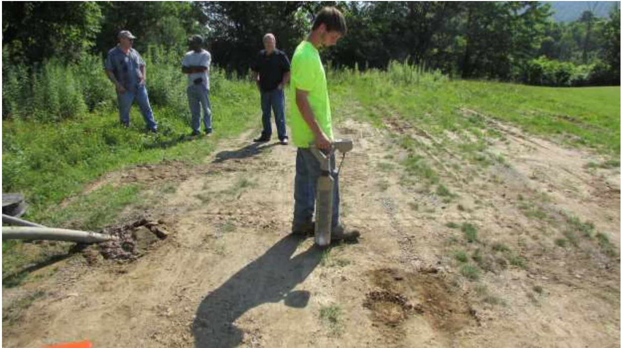
Using instrument to verify location and depth of drill head
