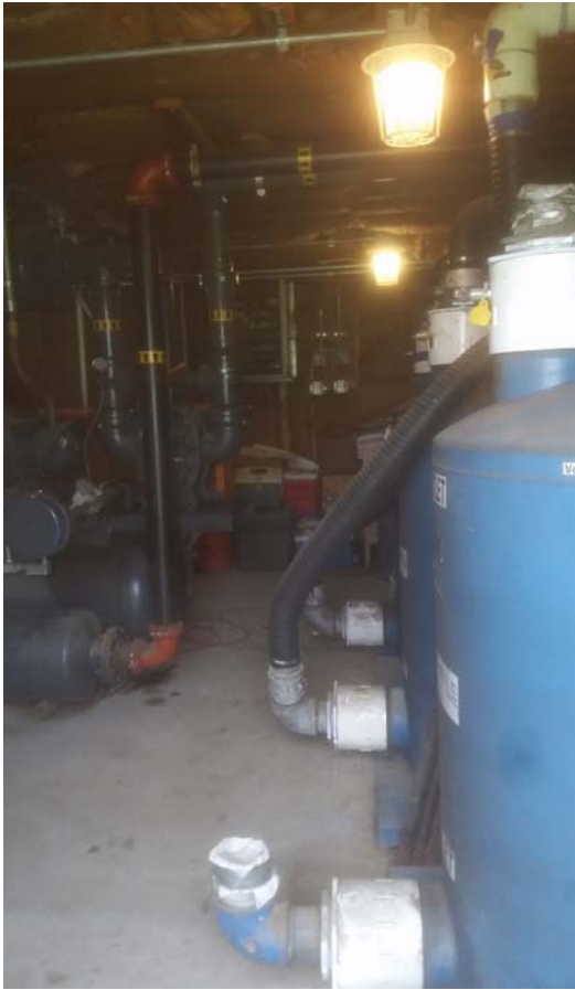
Picture 2 - Main Treatment Building Interior
