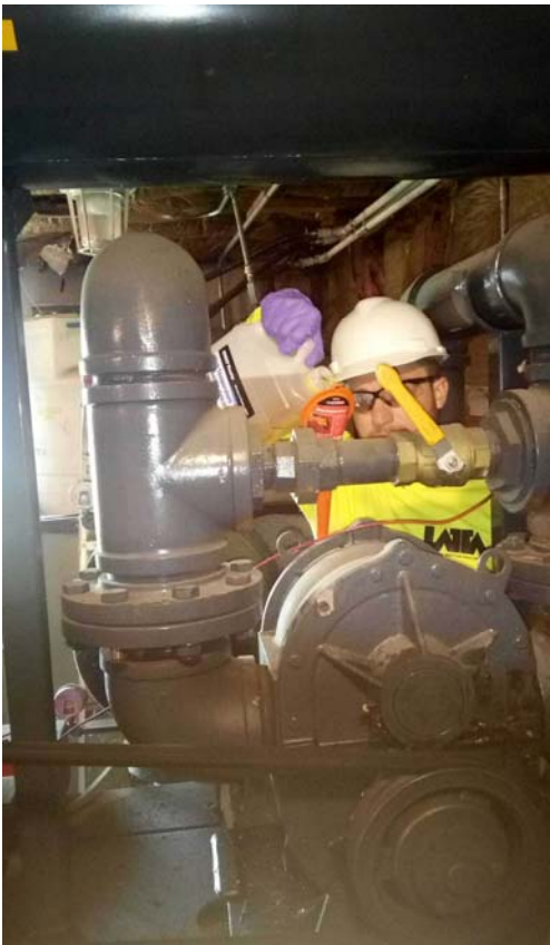
Picture 4 - Refilling the Injection and Vacuum Blowers With Oil
