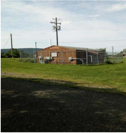
Picture 1 - Main Treatment Building Exterior
