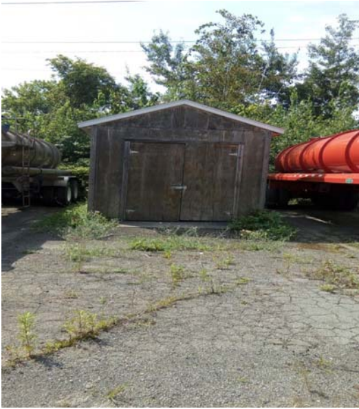
Picture 5 - Distribution Cell 1 Exterior
