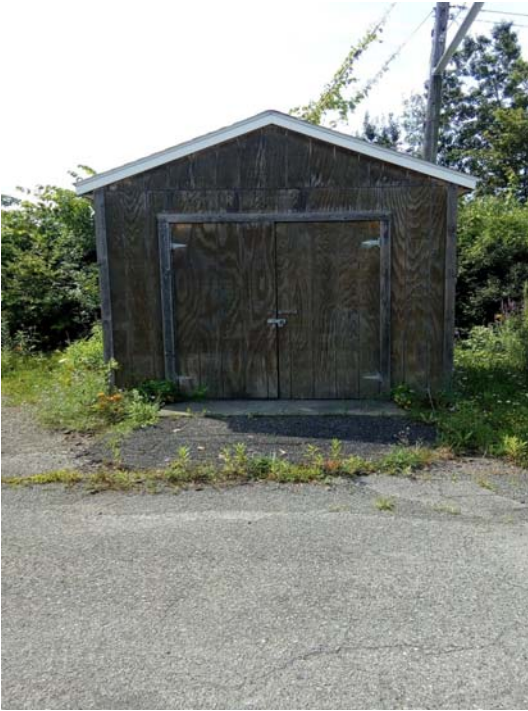
Picture 7 - Distribution Cell 2 Exterior
