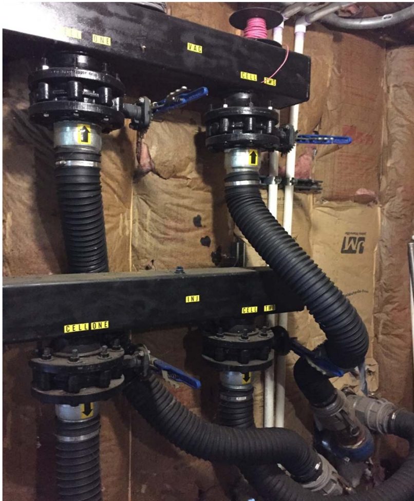
Picture 4 - All Valves on Influent and Effluent Manifolds Closed
