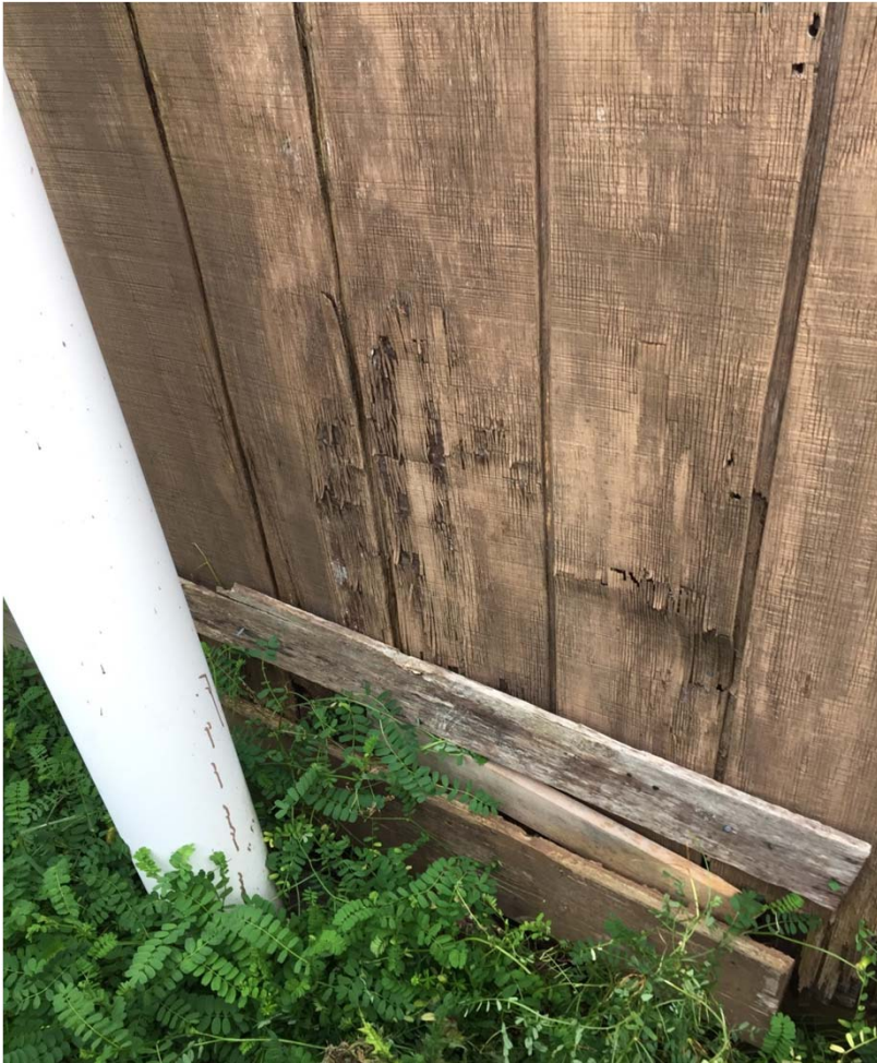
Picture 2 - Patched Hole on Main Treatment Building South Wall
