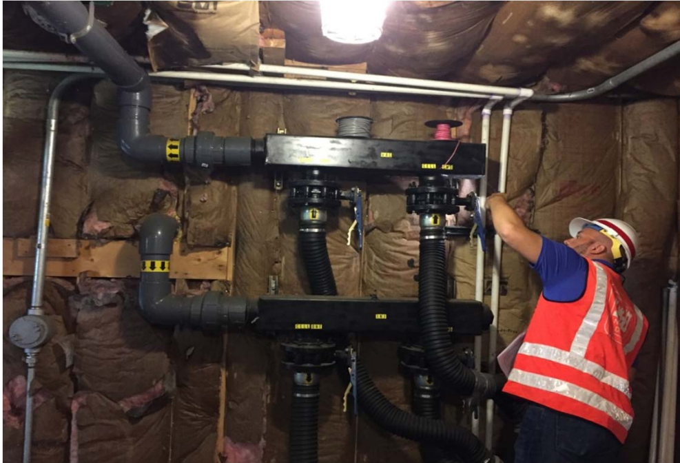
Picture 3 - Closing Valves on Vacuum Influent Manifold
