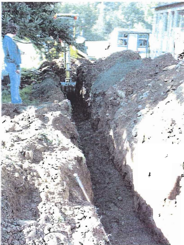
Excavation for water line and existing well abandonment at 1495 East Windsor Road
