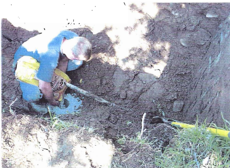
Well Abandonment at 1495 East Windsor Road using bentonite clay (Holeplug) Note distance from house
