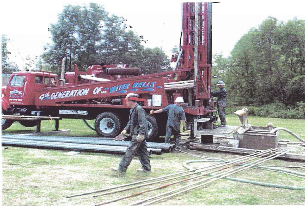
Setting 6-inch steel casing, note 1-inch tremie line in foreground
