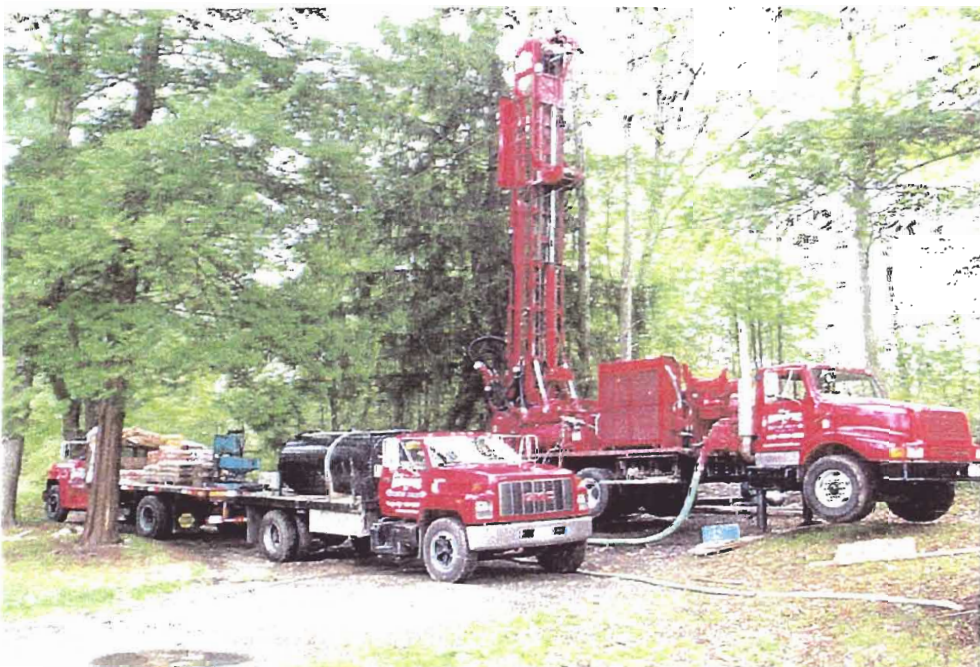
Setting 6-inch steel casing, note 1-inch tremie line in foreground
