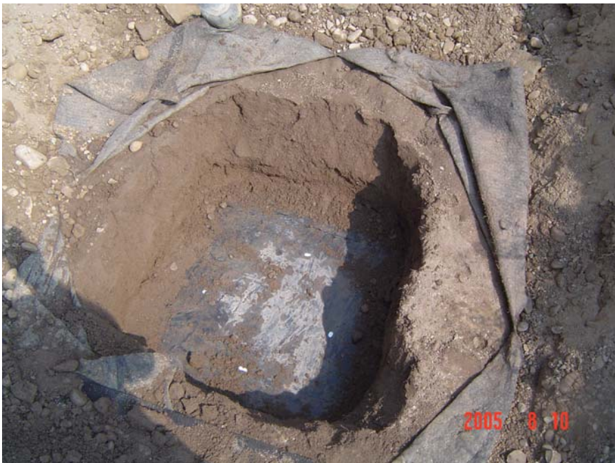
COLE-4 Investigation Location Liner Exposed
