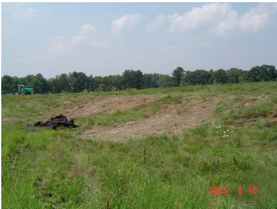
Backfilled Test Pits
