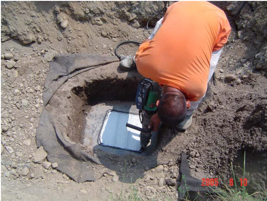
COLE-4 Investigation Location Liner Repair Welding
