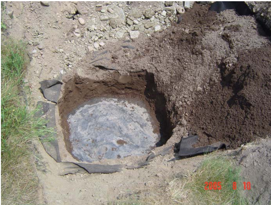
COLE-1 Investigation Location Sample Preparation
