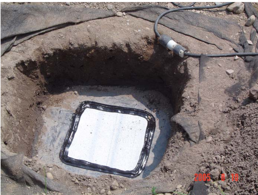
COLE-4 Investigation Location Liner Repair
