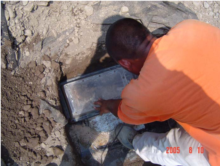
COLE-4 Investigation Location Liner Repair Vacuum Box QA Test
