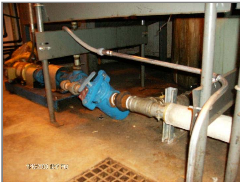
Filter in-line beneath the molassas tanks which is visible in the image describing feed-grade and food-grade.
