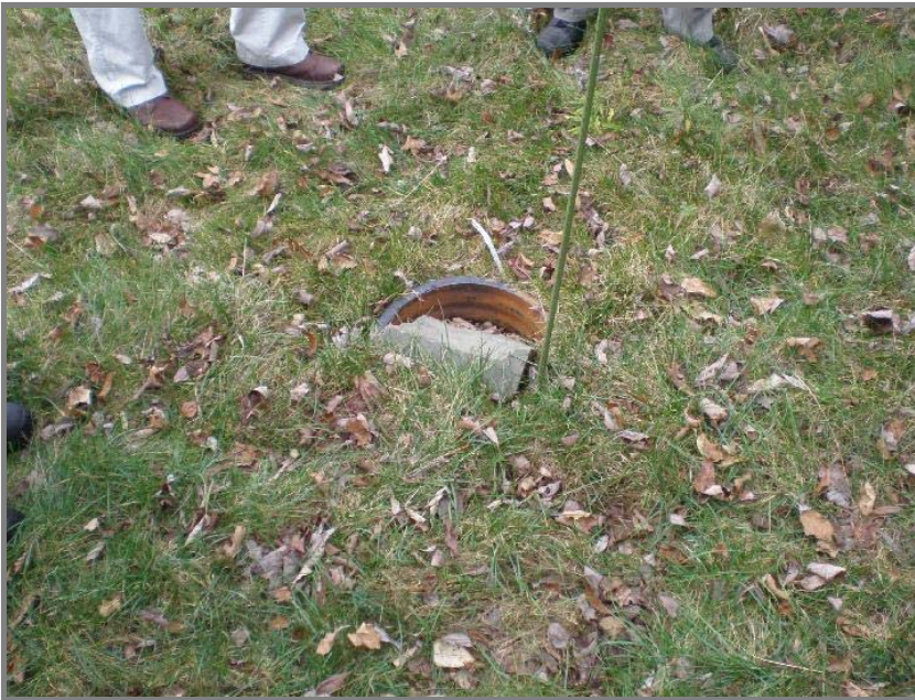
Cleanout to access the outfall
