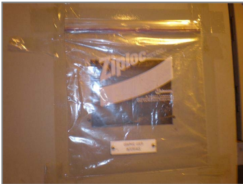
Missing panel cover. A blank needs to be installed.
