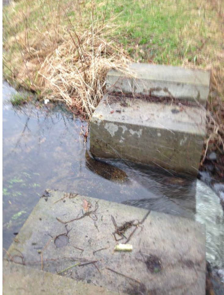
ABP Discharge Structure (cleaned) 4/23/15
