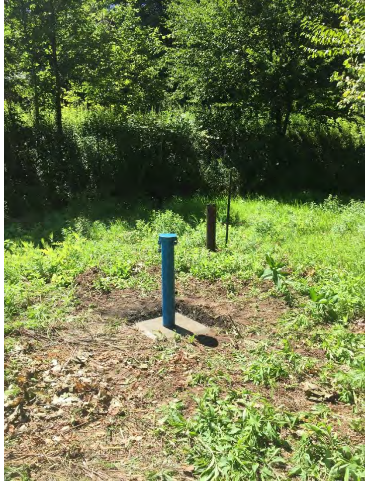
Repaired Well (MW-1D) 8/13/15
