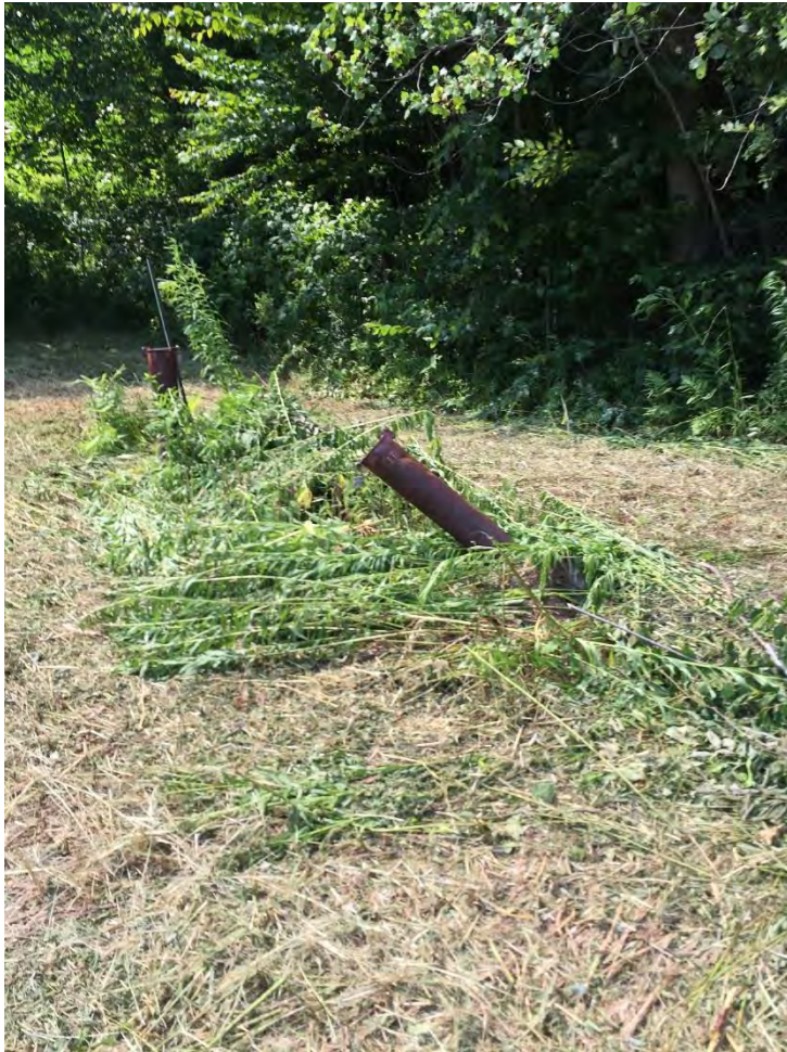
Damaged Riser (MW-1D) 7/13/15
