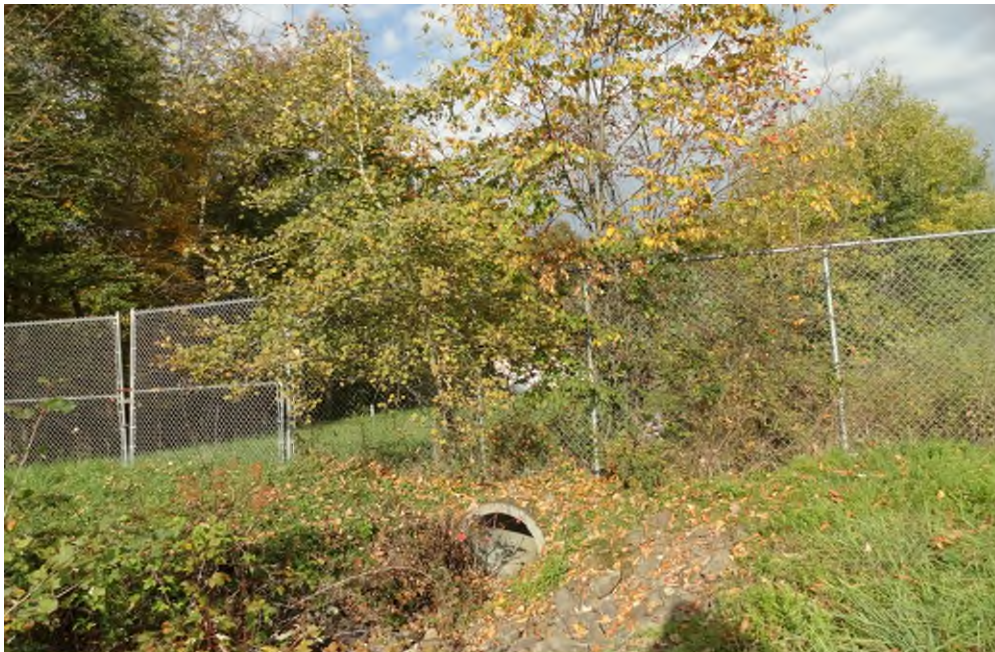
West end drainage outlet
