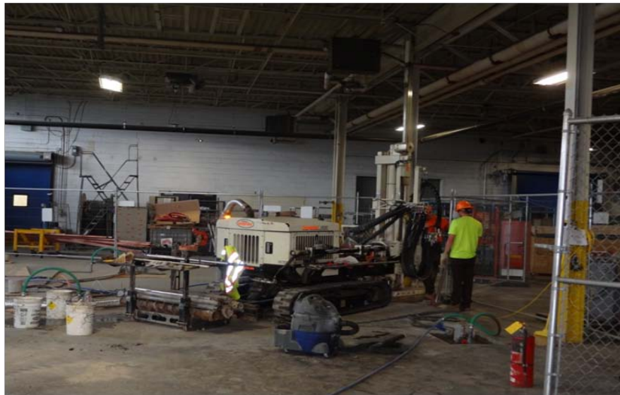
Direct Push Drilling in the Interior CFC Area
