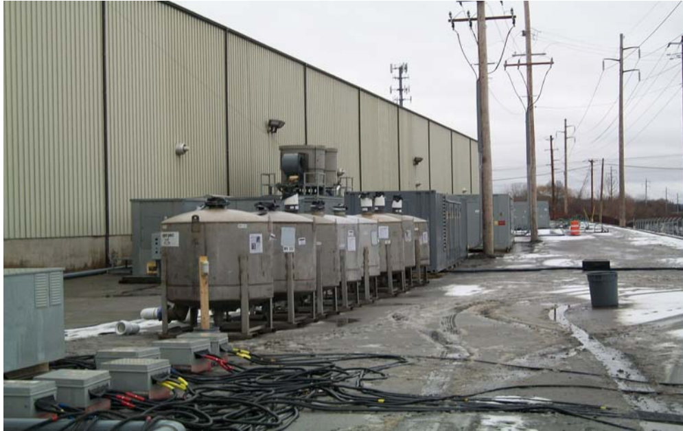
3. Equipment Compound with Vapor Treatment Vessels
