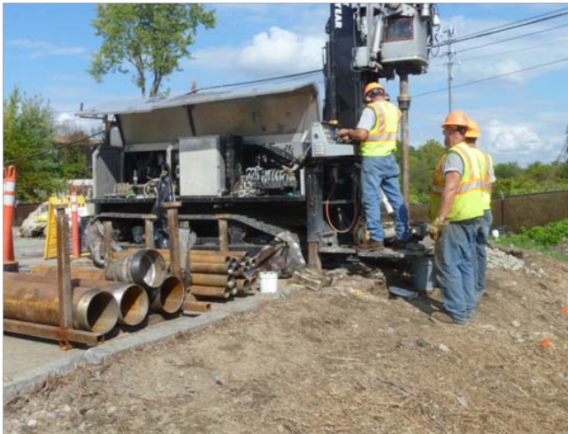
Installation of Bored Electrode by Boart Longyear in Waste Solvent Area
