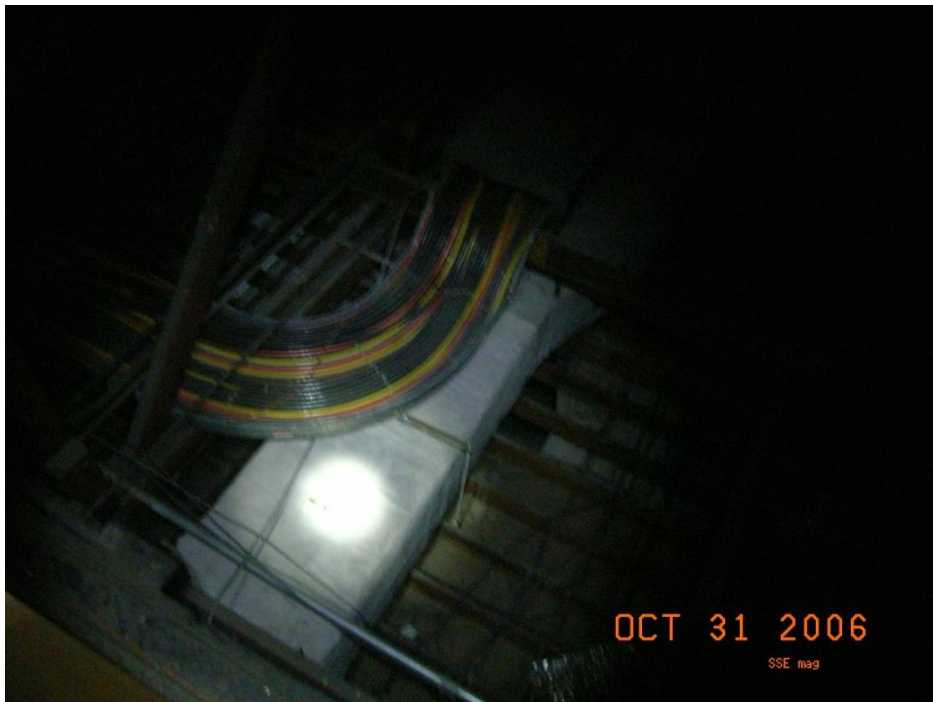
Transite Duct above Catwalk
