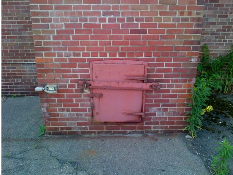
Access Door to Incinerator Stack (East Side of Building)
