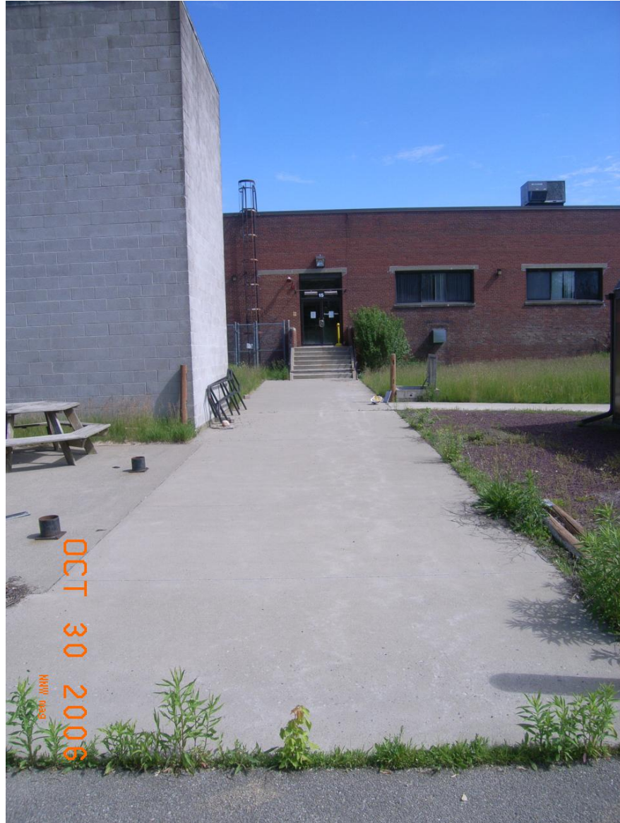
Heated Sidewalk outside exit 15 & JP-4 Building (left)
