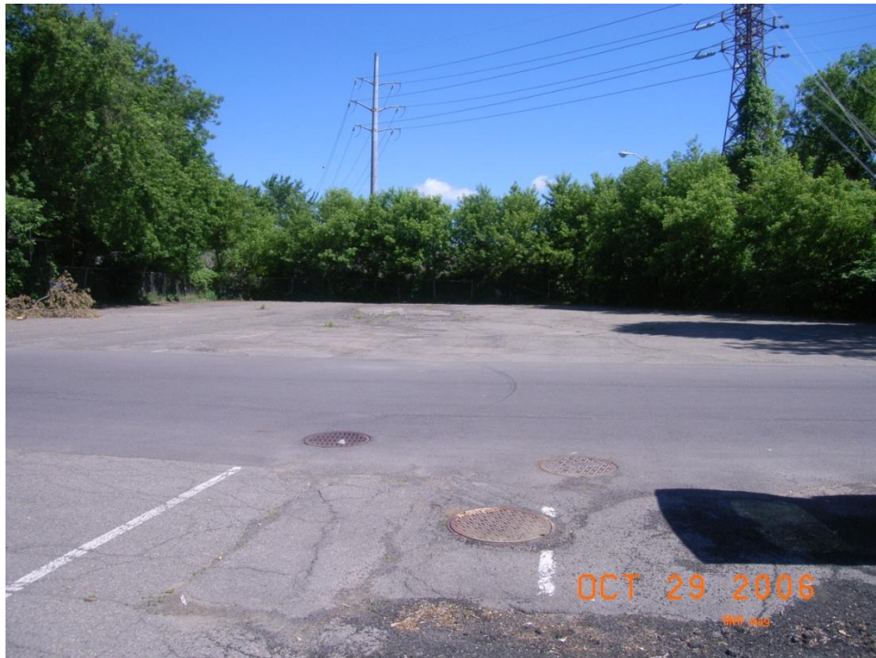
Oil Water Separator North Parking Lot
