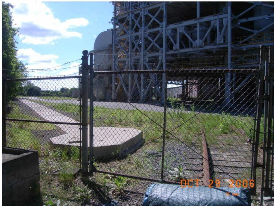
Fence to Power Plant
