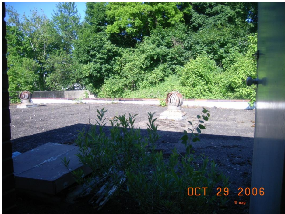
Roof of Reservoir
