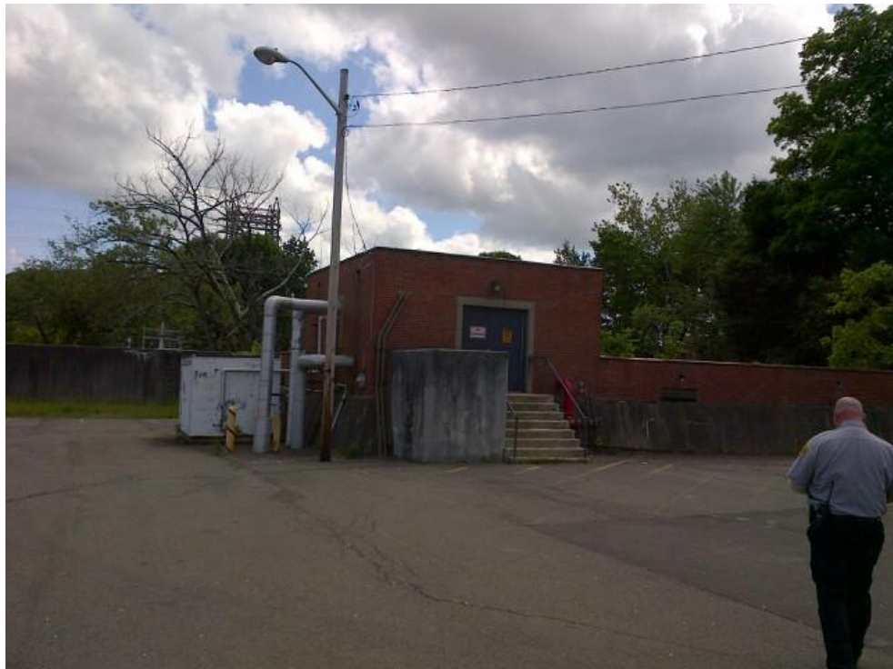
Pump House and Reservoir Building, SW Corner of Property
