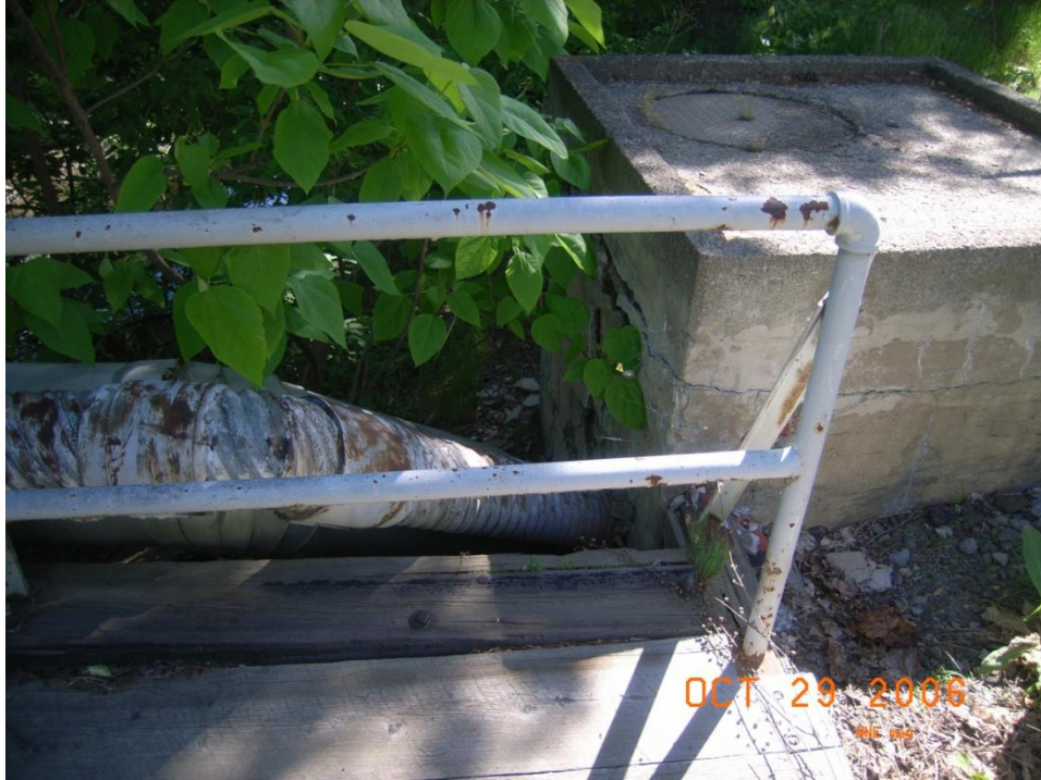
Steam Pipes go underground at the south end of the bridge
