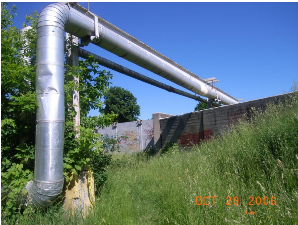
Steam Pipe over the Concrete Wall and Berm
