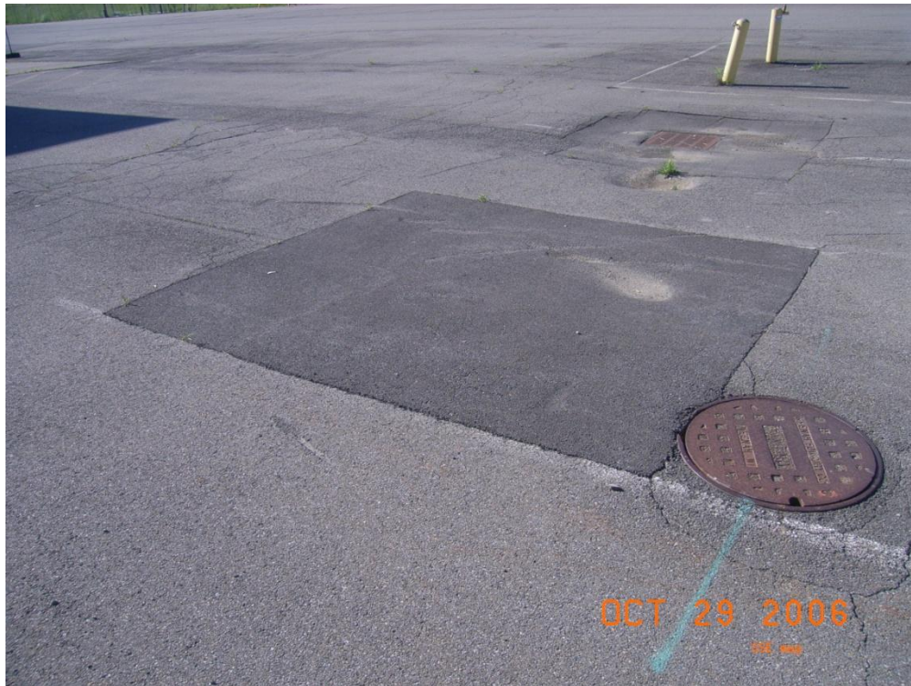
Oil Water Separator near Exit 16
