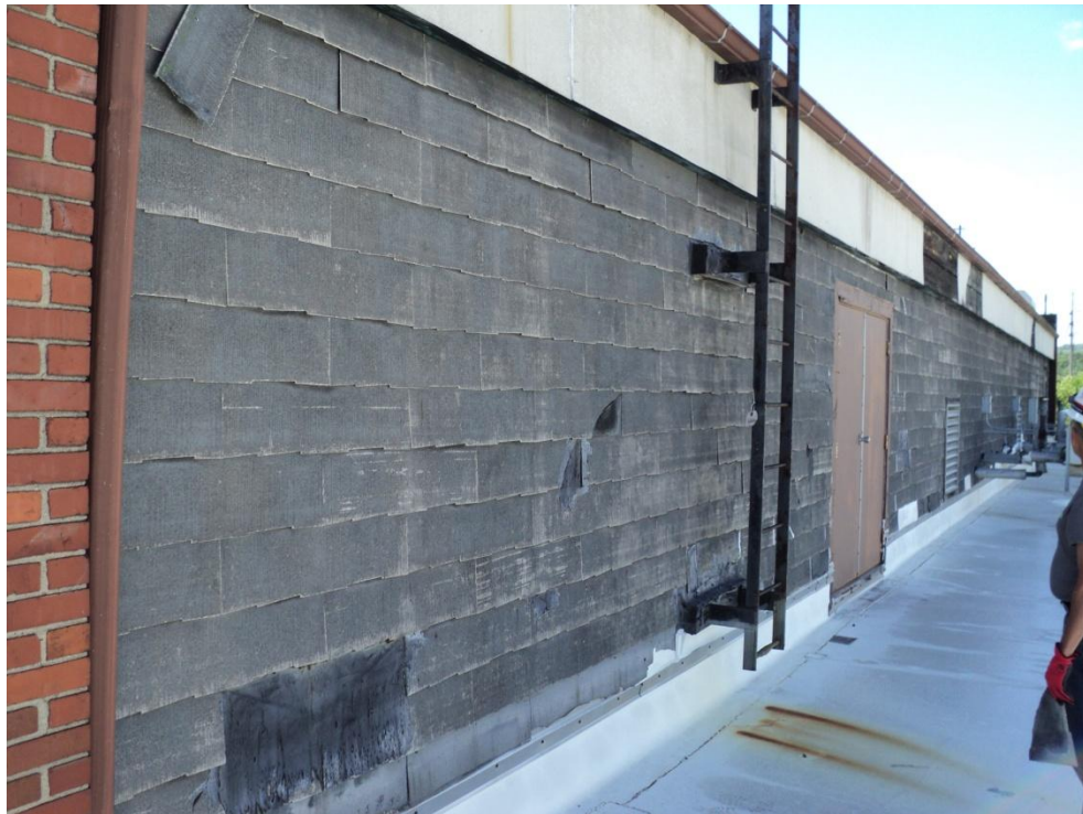
Transite Shingles on Roof
