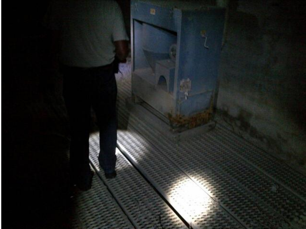
Pit Covered with Grate in Basement (SW) Area
