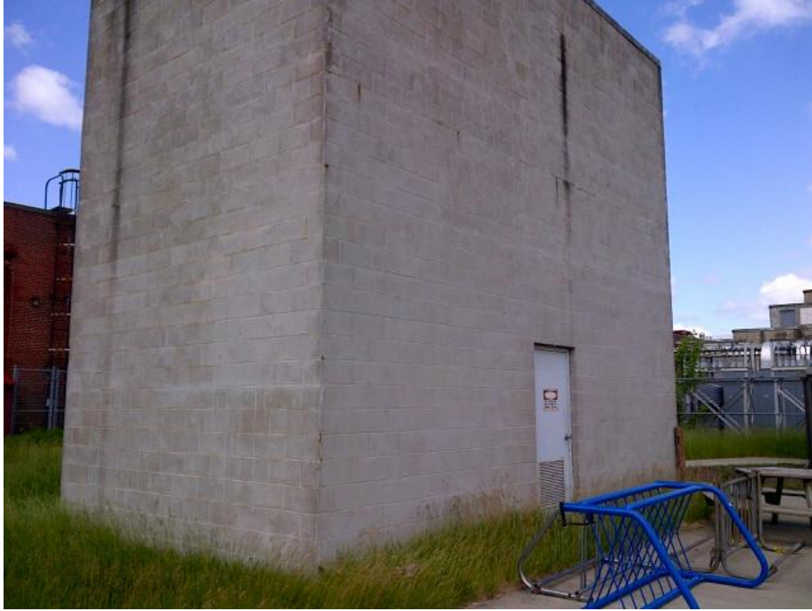
JP-4 Storage Building
