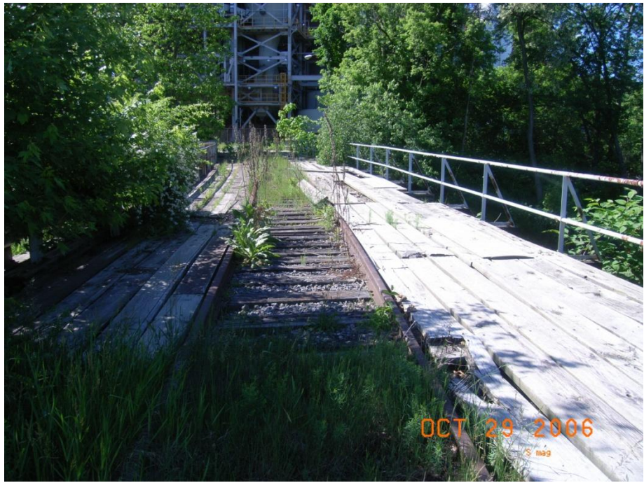
Train Trestle (Looking toward the Power Plant)
