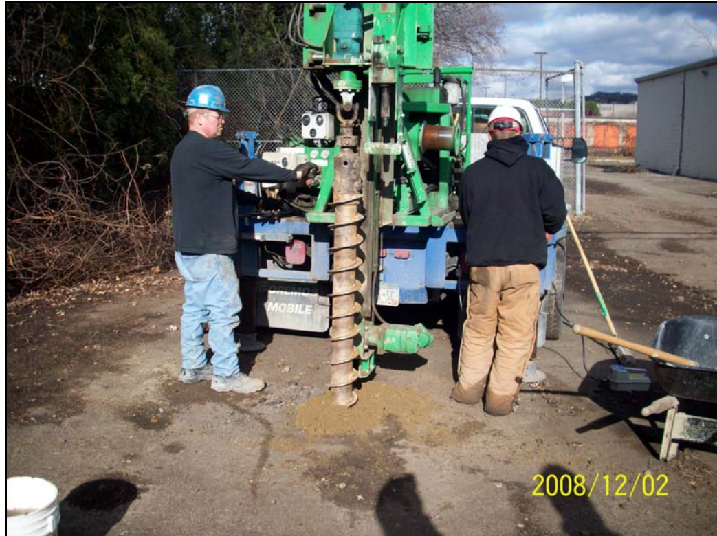
Photo 1 Drilling monitoring well MW-08, Former Bright Outdoors Site
