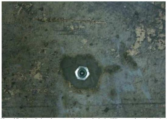
Figure 6: View of final installation of vapor monitoring point in the NW corner of warehouse (typical) (PM)
