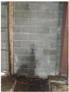
Figure 3: View of first attempt at core drilling through the wall (Looking West PM)
