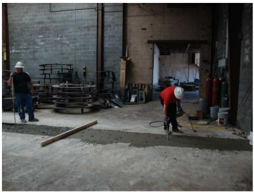
Figure 5: View of vibrated concrete (Looking South AM)
