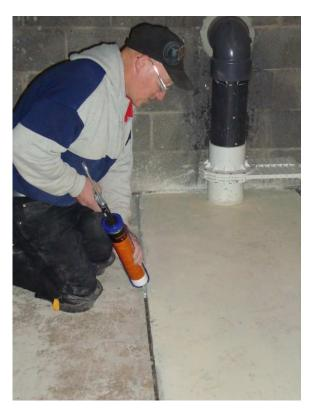
Figure 5: View of joint being sealed (Looking West PM)
