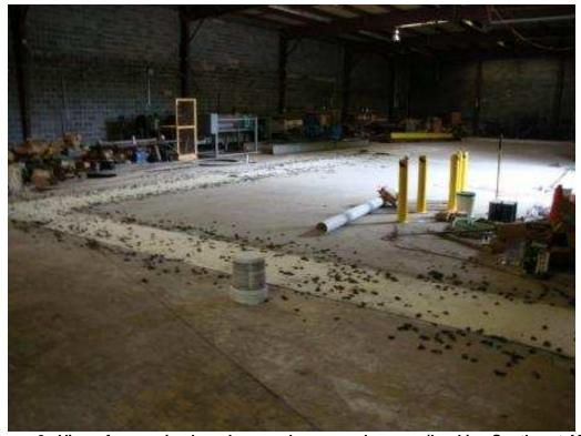
Figure 2: View of expansion board removal progress by noon (Looking Southeast AM)
