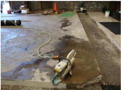
Figure 1: View of contractor's attempt to make a clean cut at broken corner (Looking West AM)
