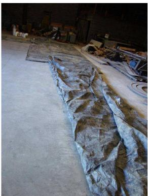
Figure 1: View of concrete covered with blankets (typical) (Looking North AM)
