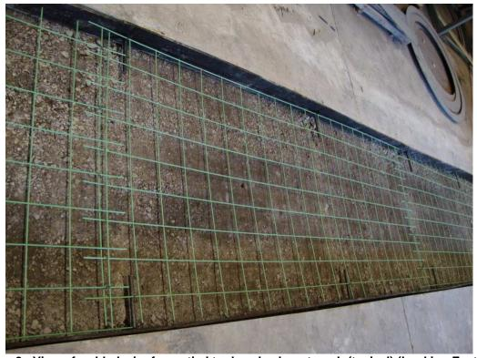
Figure 2: View of welded wire frame tied to dowels along trench (typical) (Looking East AM)
