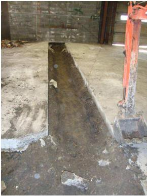
Figure 3: View of soil excavation of trench for northern fan system (Looking West PM)
