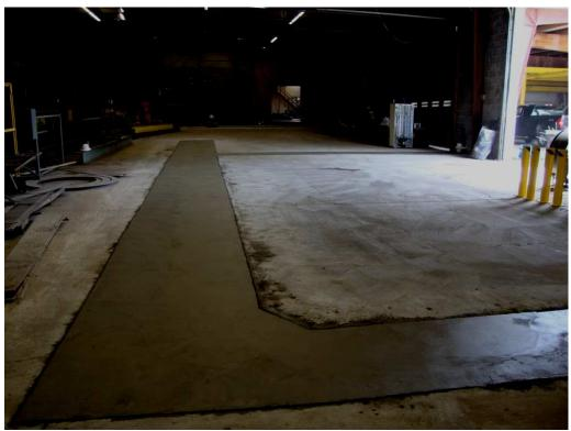
Figure 9: View of concrete after troweling (Looking South PM)
