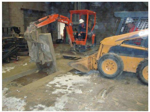
Figure 2: View of concrete removal and plastic discovered under concrete; spots caused by dust on camera lens (Looking Southwest AM)
