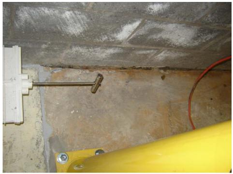
Figure 4: Second view of the open expansion joint where the floor meets the exterior wall
