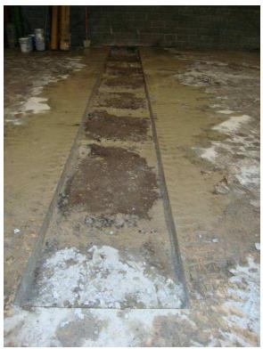
Figure 3: Concrete removed at southern-most fan system (Looking West PM)
