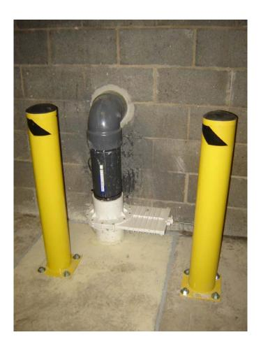
Figure 2: View of Soil Vapor Extraction unit #3 – north unit
