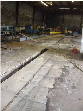
Figure 1: View of saw-cut concrete along trench (Looking East AM)
