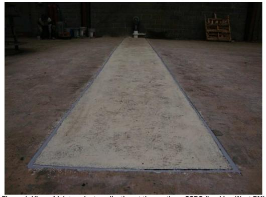
Figure 4: View of joint sealant application at the southern SSDS (Looking West PM)
