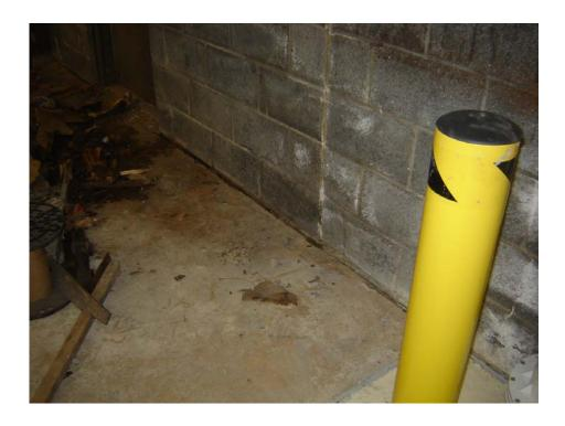
Figure 3: View of the open expansion joint where the floor meets the exterior wall
