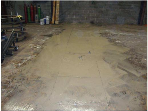
Figure 3: View of relief cuts in concrete (typical) for southern fan system (Looking West PM)
