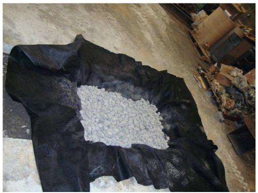
Figure 4: View of 2" stone placed over well screens (typical) (Looking Northeast PM)
