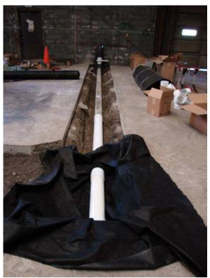
Figure 2: View of final assembled drainage pipe and well screen (typical) (Looking West AM)
