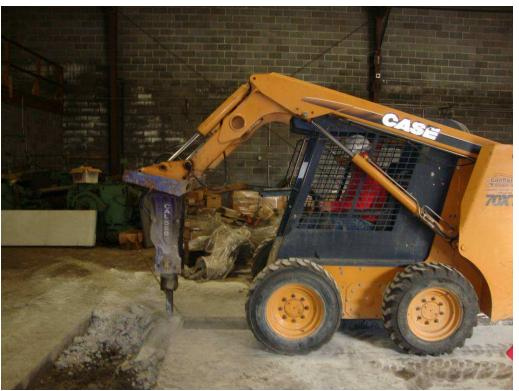
Figure 5: Jack hammering at north end of trench (Looking East PM)
