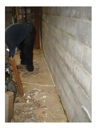
Figure 8: View of OP-TECH personnel filling the floor /wall expansion joint with caulk
