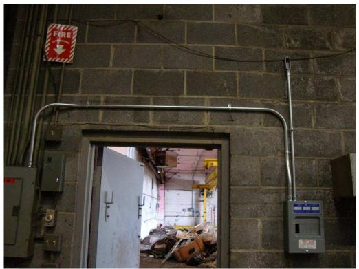
Figure 3: View of installed circuit box and conduit in the southwest corner of the warehouse (Looking East PM)
