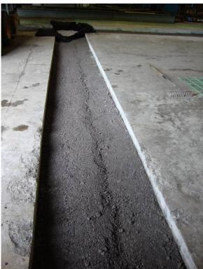
Figure 1: View of compaction along center drainage piping (typical) (Looking East AM)
