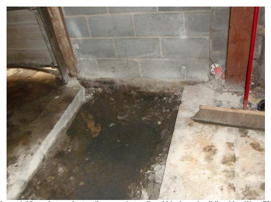
Figure 4: View of stone footer discovered at wall and blackened soil (Looking West PM)
