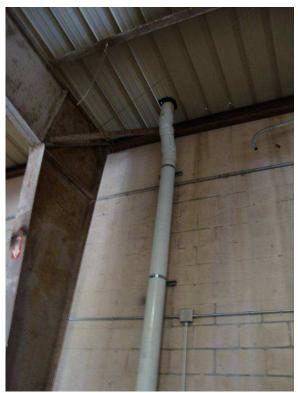
Figure 4: View of vertical piping installation through roof at southern SSDS (Looking East AM)
