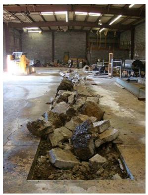
Figure 3: View of broken up concrete/trench drain at end of day (Looking North PM)
