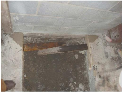
Figure 3: View of concrete patches by wall of center fan system trench (Looking West AM)
