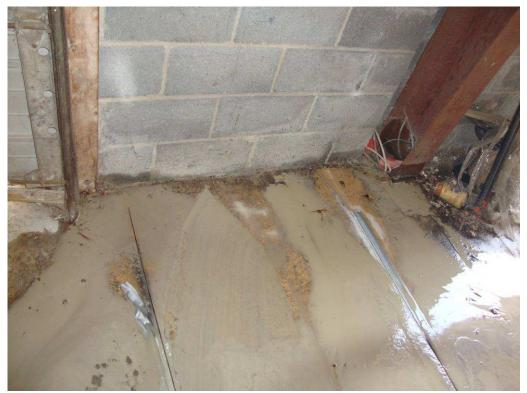
Figure 2: View of saw-cut concrete near wall for middle fan system (Looking West PM)
