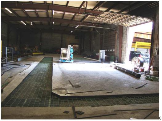
Figure 4: View of site preparation for pouring concrete (Looking South PM)
