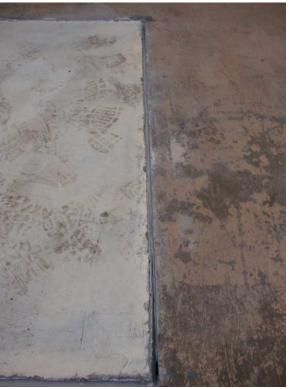
Figure 3: Close-up view of joint sealant application (typical) note that most joints required multiple layers of the caulk/sealant (Looking East AM)
