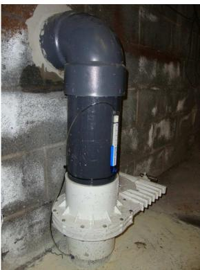
Figure 1: View of installed manometer at the northern SSDS (typical) (Looking Northwest AM)
