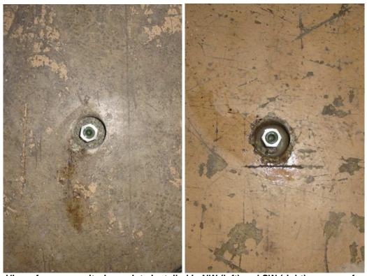
Figure 2: View of vapor monitoring points installed in NW (left) and SW (right) corners of warehouse before addition of concrete (AM)
