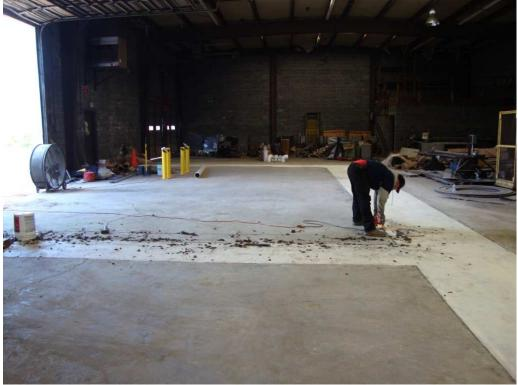
Figure 2: View of expansion board removal for joint sealant (Looking North AM)
