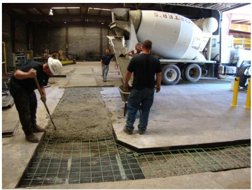
Figure 7: View of concrete placement operations (Looking South AM)
