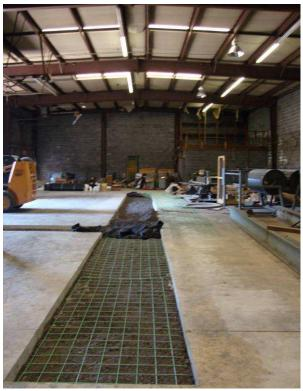
Figure 5: View of wire frame cut to size (Looking North PM)
