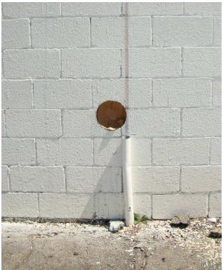
Figure 1: View of temporary hole cover (typical) and cut-off pipe (Looking East AM)
