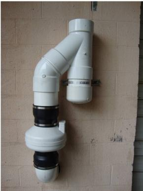
Figure 3: View of fan installation at center fan system with temporary support strap (Looking East AM)
