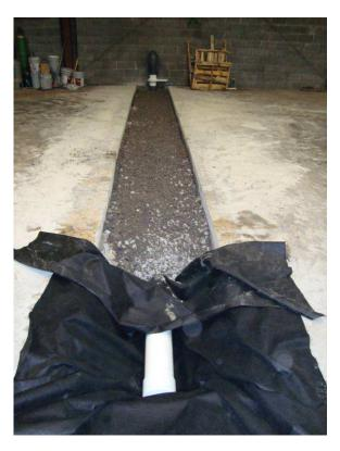
Figure 3: View of stone-filled trench (typical) (Looking West PM)
