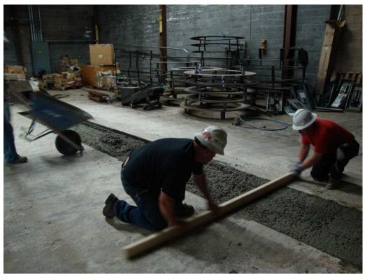
Figure 4: View of concrete leveled with 2"x4" (Looking Southeast AM)
