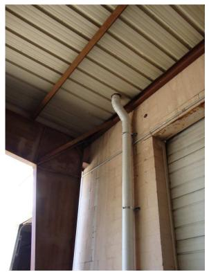
Figure 4: View of installed piping through roof for center SSDS system (Looking East PM)
