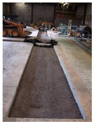
Figure 2: View of compaction in trench drain area (Looking North AM)
