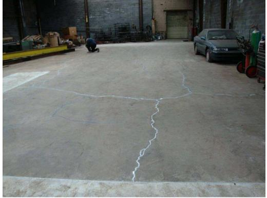
Figure 2: View of cracks being sealed (Looking South AM)
