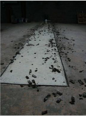
Figure 3: View of expansion joint removed (Looking West PM)
