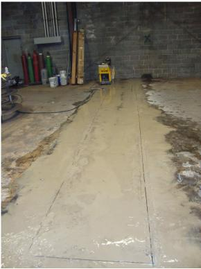
Figure 1: Cut concrete for southern most fan system (Looking west AM)
