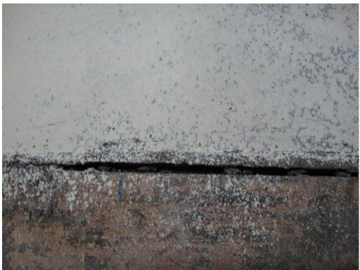
Figure 3: Close up view of expansion board where separated from existing concrete (Southern SSDS, southeast corner of new concrete, Looking North AM)
