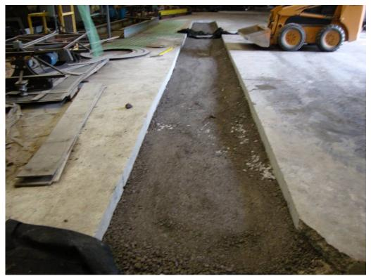
Figure 4: View of compacted fill mix of 2" and 1 1/2" with fines at northern end (Looking South PM)
