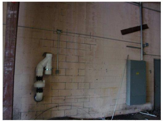
Figure 4: View of installed conduit by southern fan system (Looking Southeast PM)
