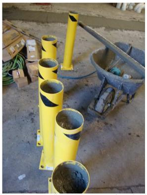
Figure 8: View of bollards filled with concrete (Looking North AM)
