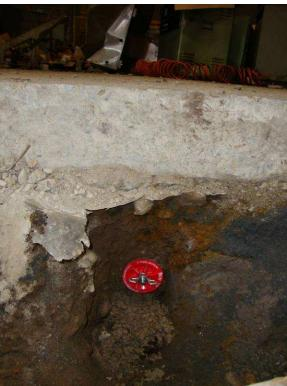
Figure 1: View of drainage pipe plugged with concrete and capped (Looking North AM)
