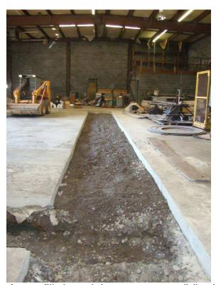
Figure 6: View of stone filled trench (not yet compacted) (Looking North PM)
