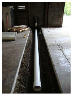
Figure 6: View of plumbing for center fan system (typical) (Looking West AM)
