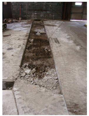
Figure 4: Concrete removed at northern-most fan system (Looking West PM)
