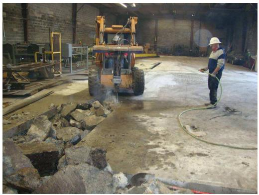
Figure 1: View of concrete removal with dust suppression. (Looking South AM)
