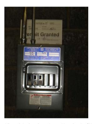
Figure 7: View of the interior subpanel box for the SVE units
