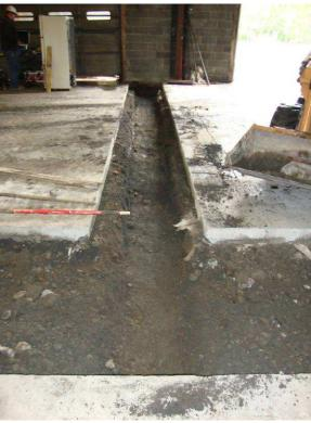
Figure 3: View of soil excavation for center fan system (Looking West PM)
