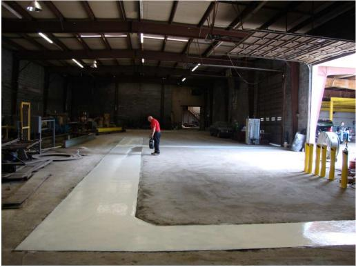
Figure 10: View of sealant being sprayed on (Looking South PM)
