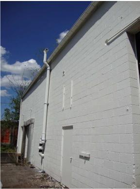
Figure 3: View of installed piping for northern SSDS system (Looking Northeast AM)
