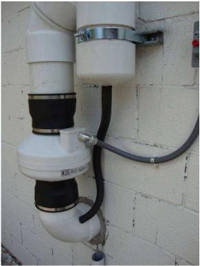
Figure 5: View of condensate bypass for northern SSDS (typical) (Looking North PM)
