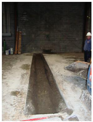
Figure 2: View of soil removed for center fan system (Looking West PM)
