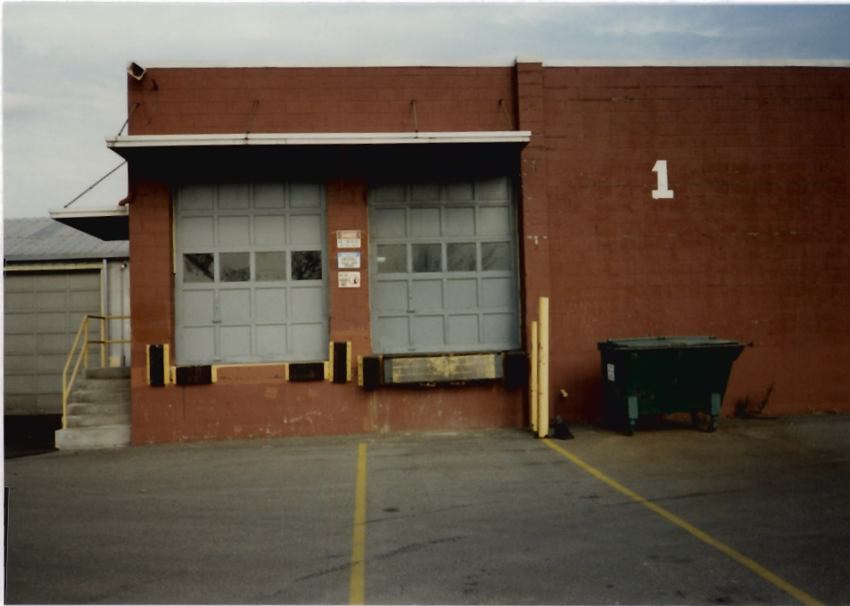
7. View of the loading docks for the Hazardous Waste Container Storage and Staging Area (SWMU 1) facing north. The general refuse Dumpster (SWMU 12) is shown on the right.
