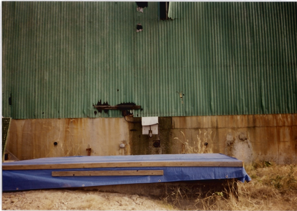
23. View of the Neutralization Pit (SWMU 2) facing east. The Fume Scrubber (SWMU 5) was located inside the wall shown in the center of the photograph.
