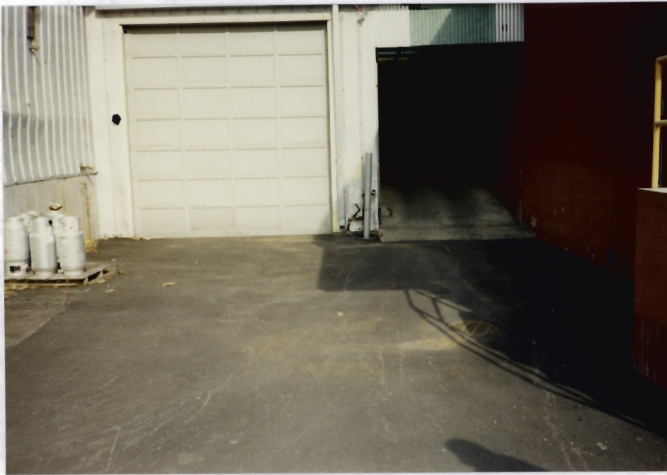
5. View of the ramp between Warehouse No. 1 and 2 showing the catch basin connected to the storm sewer. The red building on the right is Warehouse No. 1.
