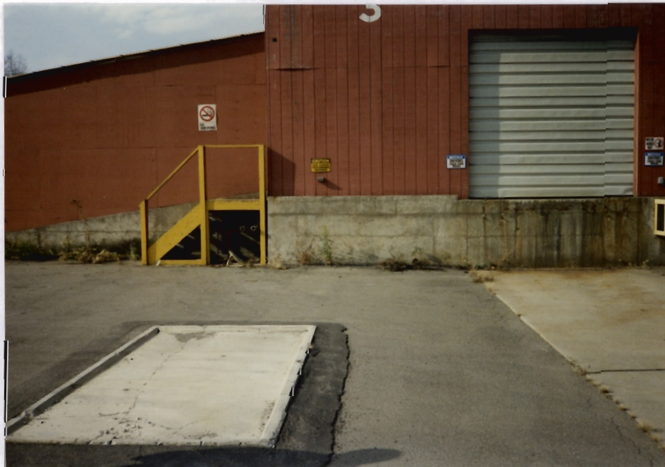
18. View of Warehouse No. 3. showing Solvent Tank Truck Loading/Unloading Area (SWMU 9) identified by the small concrete pad shown in the foreground. The view is facing west.
