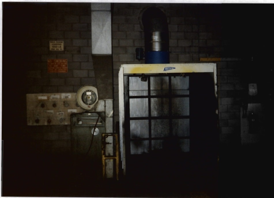
25. View inside Warehouse No. 4 showing an inactive paint booth previously used to paint drums. The former location of the intake pipes that were connected to the Old Tanks (Tks 7-14) is shown to the left of the booth (identified by the white square-- see next photograph).
