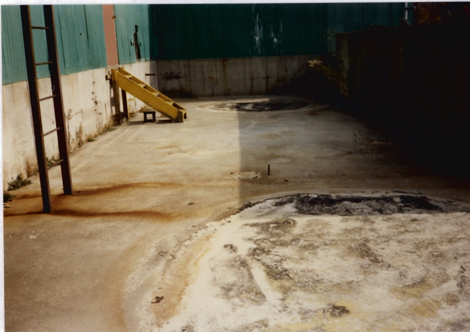
20. View outside Warehouse No. 3 showing the location of the former Solvent Tanks (Tks 1-3) facing east. These tanks were identified as SWMUs in the PR.
