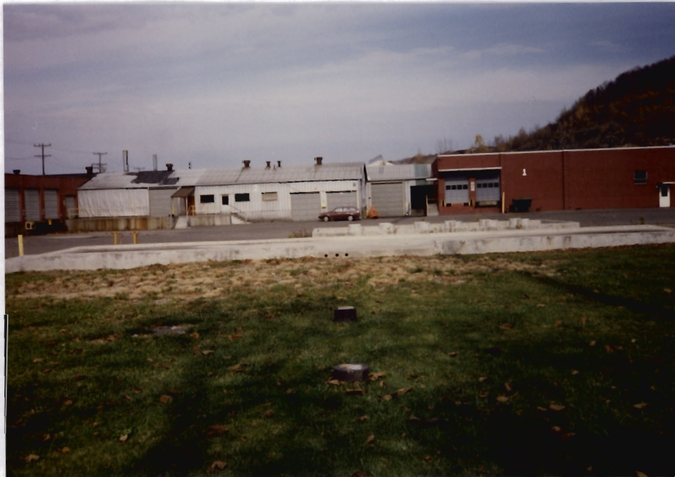
32. Overview of the facility facing north. The unused Solvent Tank Truck Loading/Unloading Area (for Tks 101-103) is shown in the center of the photograph. Warehouse No. 1 and Warehouse No. 2 are shown in the background. The black objects in the foreground are part of the pipe stand that was part of the Solvent Blend Tanks (Tks 101-103).
