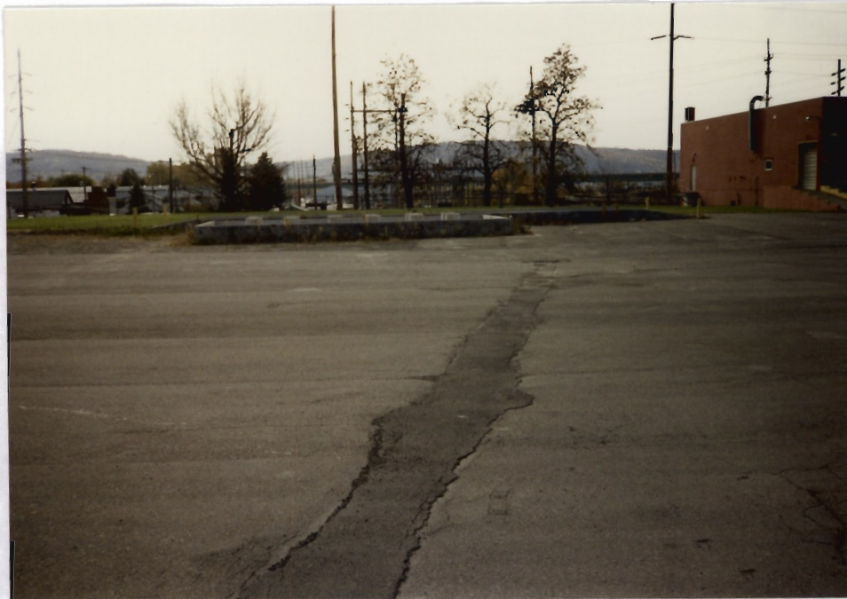
6. Overview of the south section of the facility facing south. The view shows Warehouse No. 4 on the right and the former location of the Solvent Blending Tanks 101, 102, and 103 in the center of the photograph. Another catch basin connected to the storm sewer is located at the end of the newer asphalt shown in the foreground.
