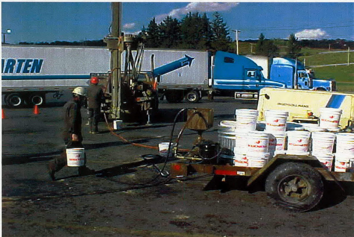
Pilot Truck Stop – HRC injection (Drill rig and trailer with pump, water bath and HRC)
