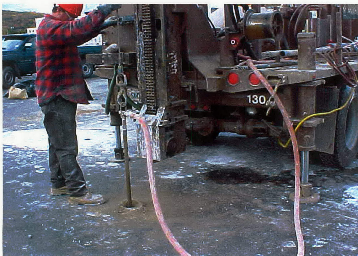
Pilot Truck Stop – ORC injection in progress through direct push rods
