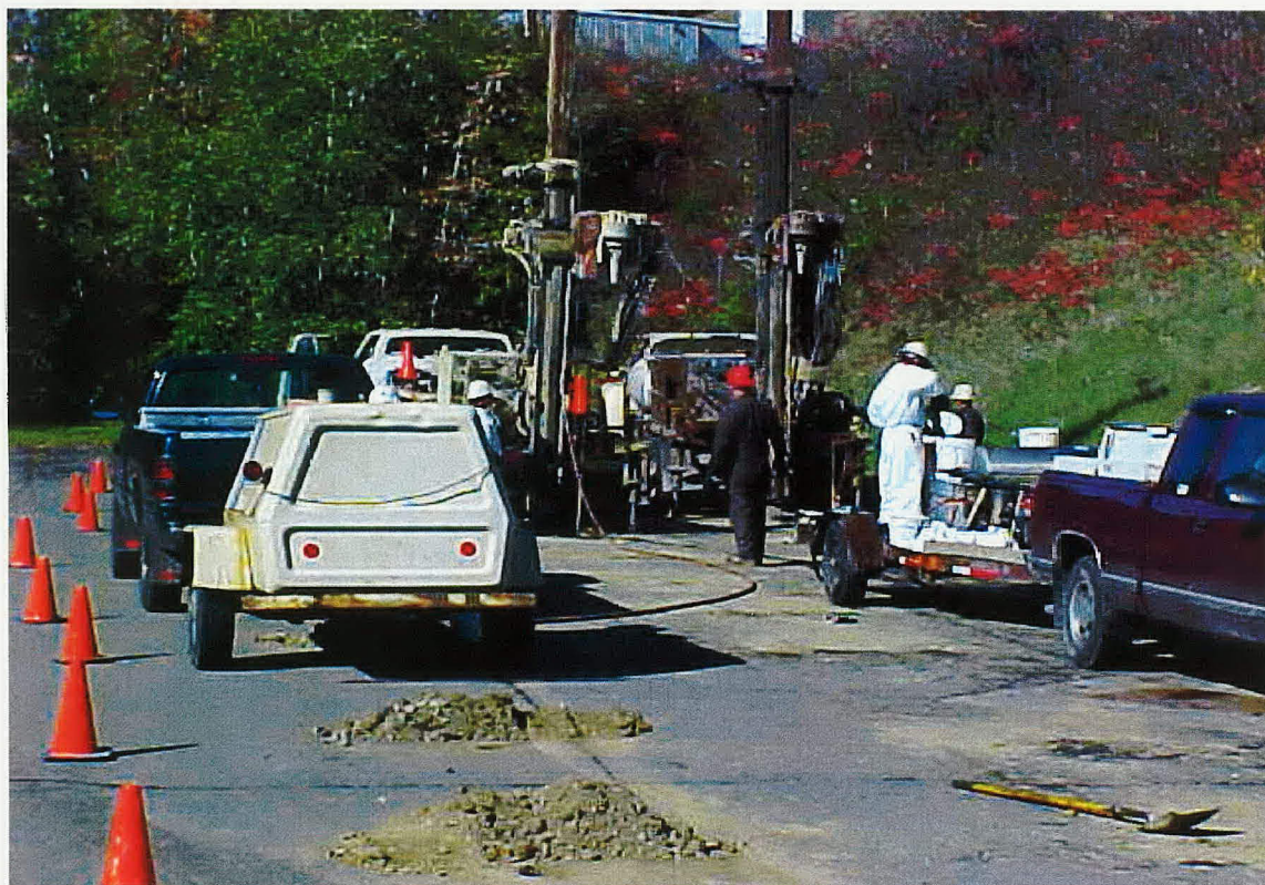
MW-7A Area – HRC injection in progress
