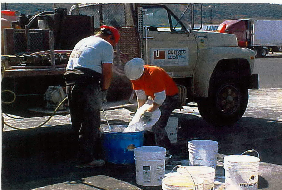
Pilot Truck Stop – ORC injection (Drill rig with pump and ORC bucket [blue])
