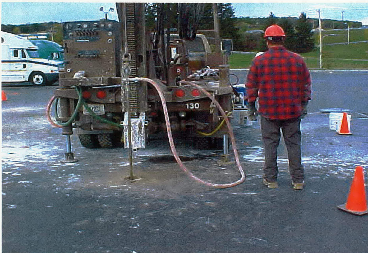
Pilot Truck Stop – ORC injection (Drill rig with pump and ORC bucket [blue])
