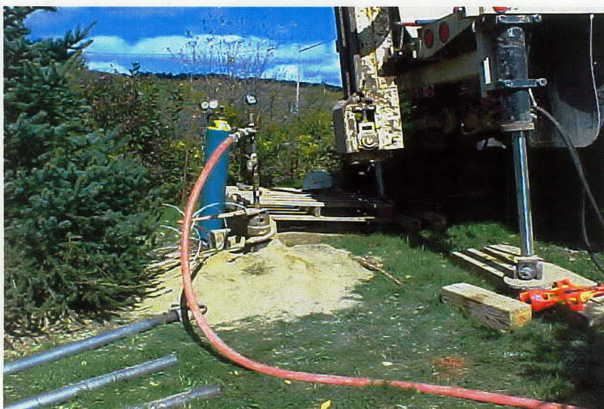
MW-24 Area – HRC injection at first point (Cylinder for packer inflation w/ inert gas)
