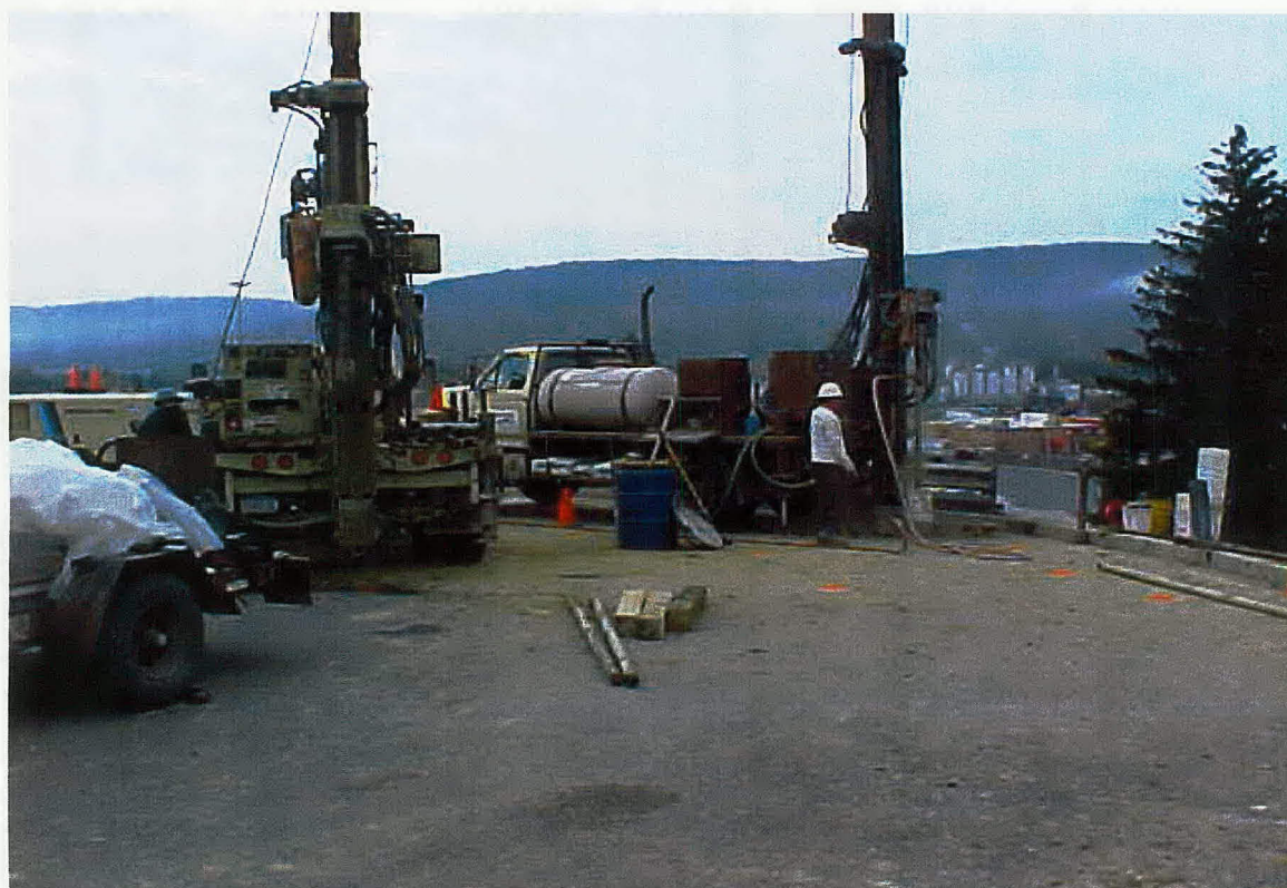
MW-24 Area – HRC injection point installation
