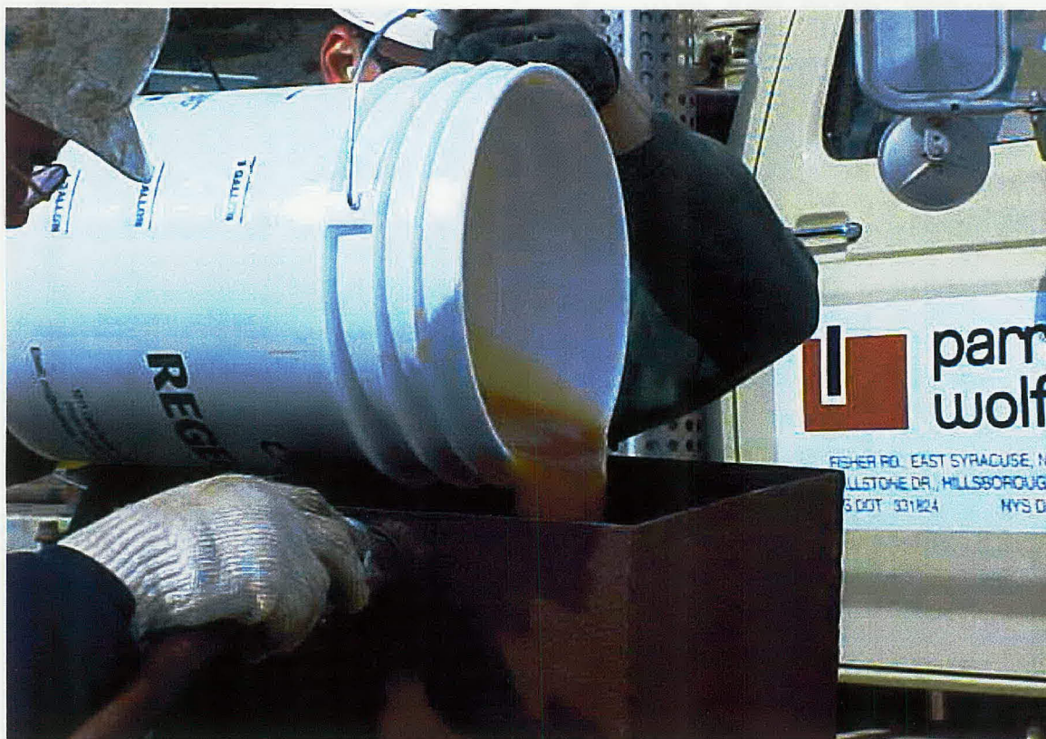
MW-24 Area – Heated HRC being poured in pump hopper
