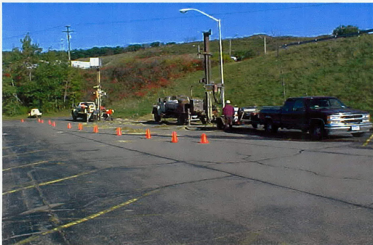
MW-7A Area – Installation of injection points
