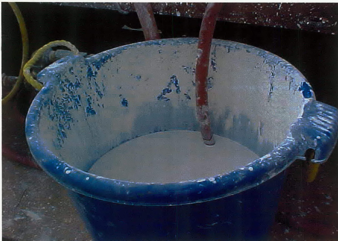
Pilot Truck Stop – ORC injection (50% solids mix) in progress
