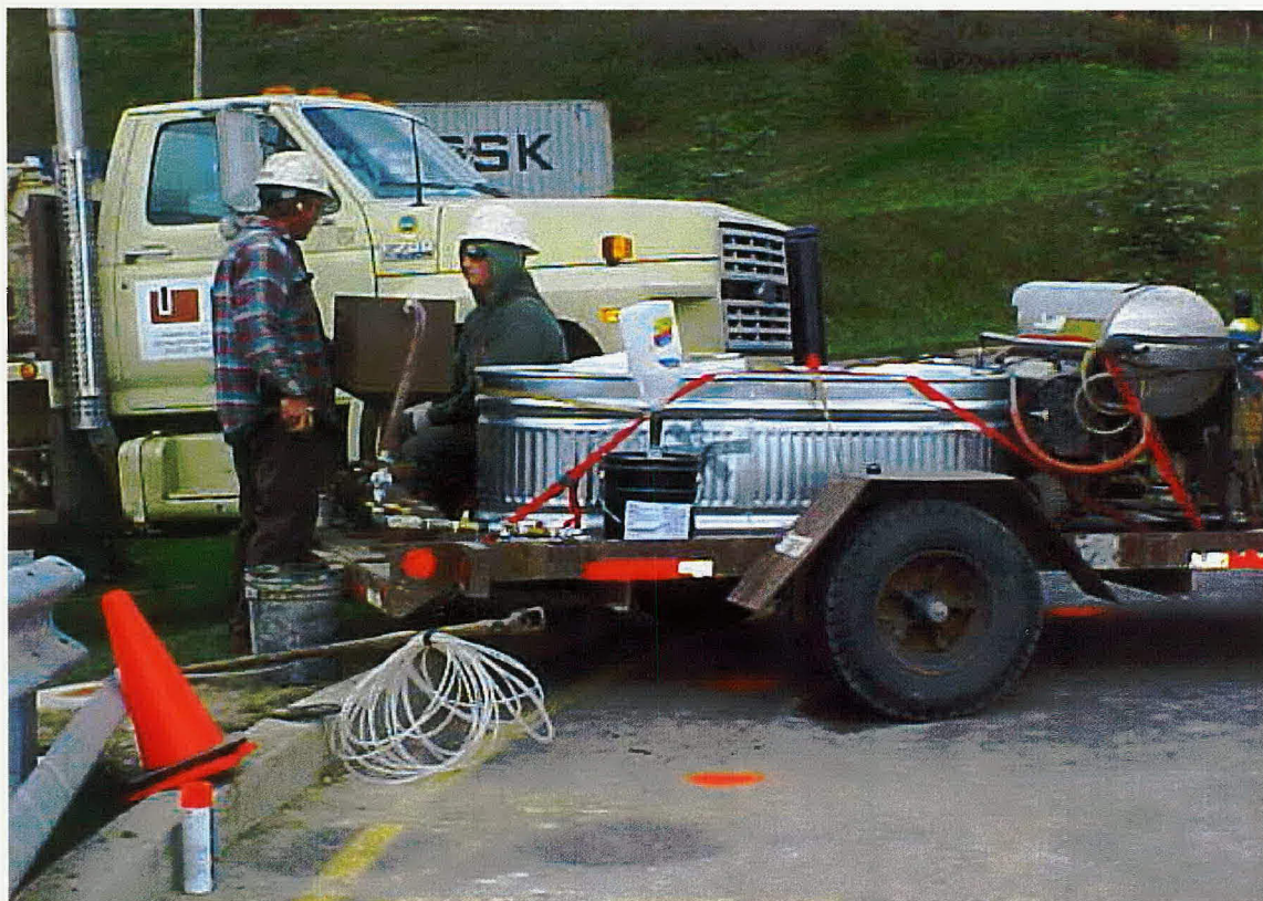
MW-24 Area – HRC injection trailer (pump and hopper, glycerin rinse, and water bath
