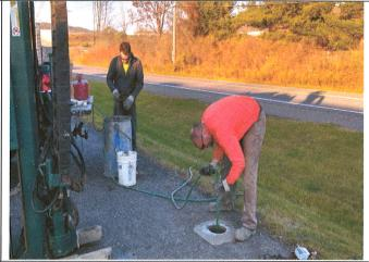
Monitoring Well MW-1 grouting.
