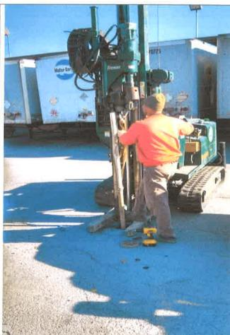
Monitoring Well GP-2 being removed.
