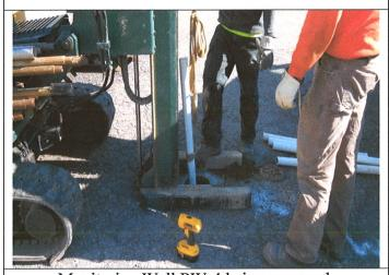
Monitoring Well PW-4 being removed.
