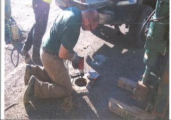
Preparing Monitoring Well MW-3 for removal.
