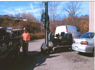
Monitoring Well PW-4 being removed.
