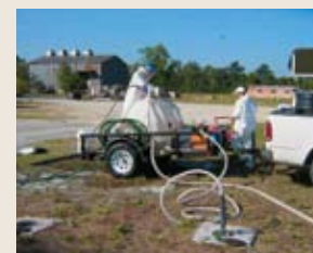
The HRC Advanced microemulsion is then injected in high-volumes into the treatment area
