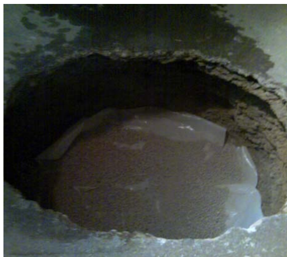
Dry Well Excavation Demarcation Layer
