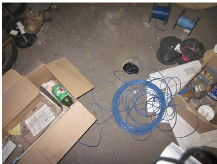
Dry Well – Pre Excavation
