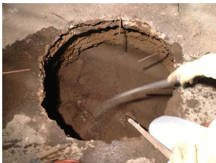
Dry Well Excavation during backfill activities
