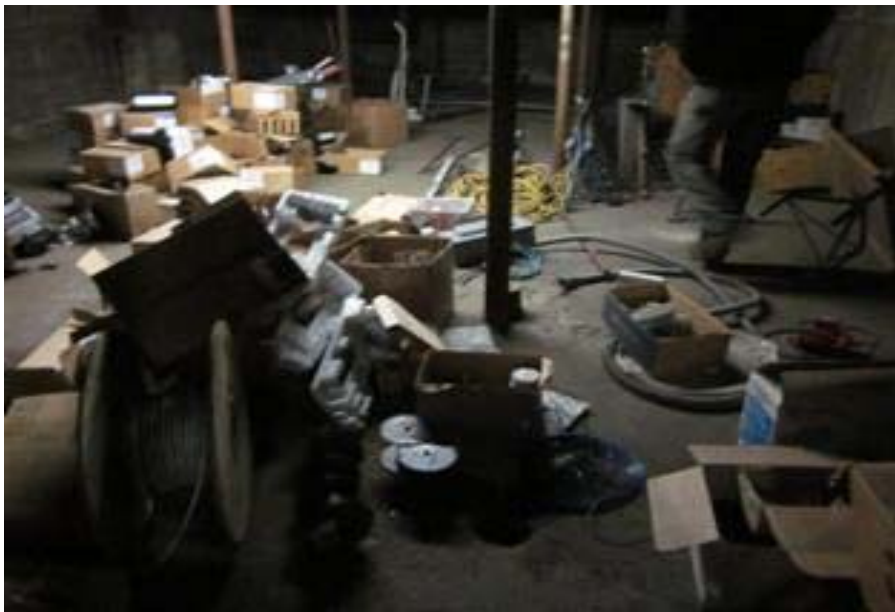
View of east unfinished basement with dry well in foreground.
