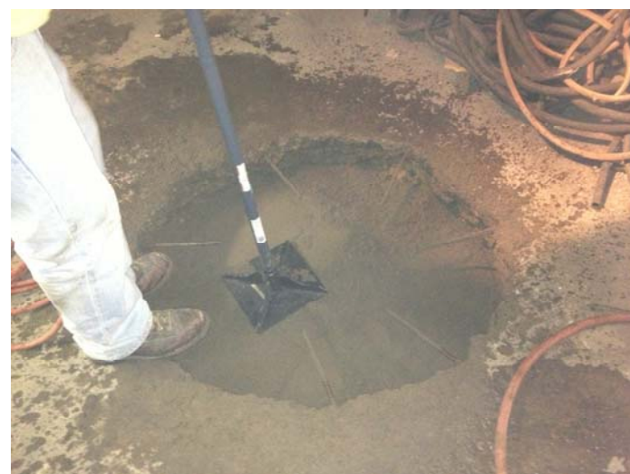
Dry Well Excavation during backfill activities
