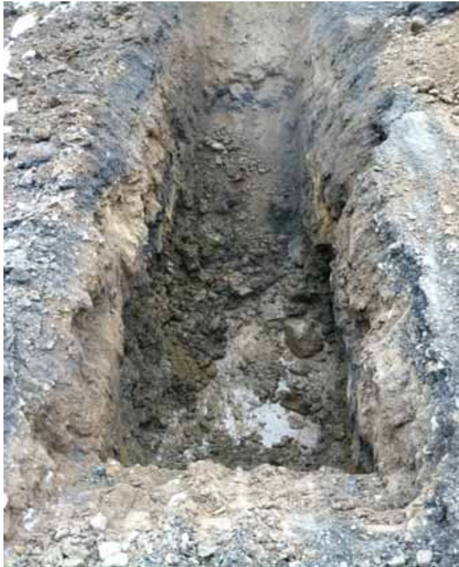
Photo #14 (2011.09.16): CTP-9. Looking south to north of test pit, no visual impacts.
