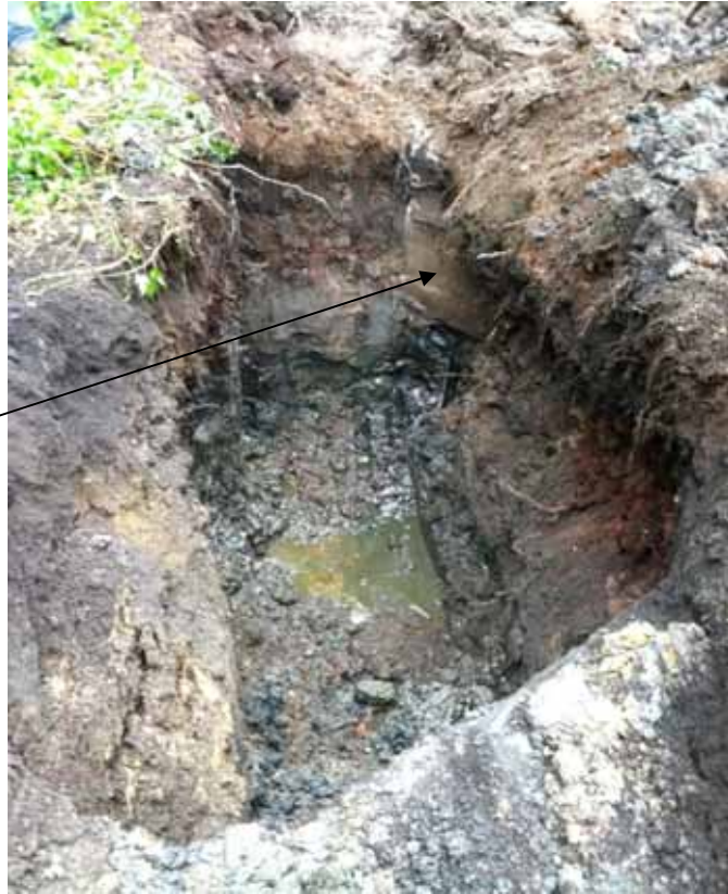
Photo #3 (2011.09.15): CTP-3. Dark stained soil looking east from top of gas holder #1.
