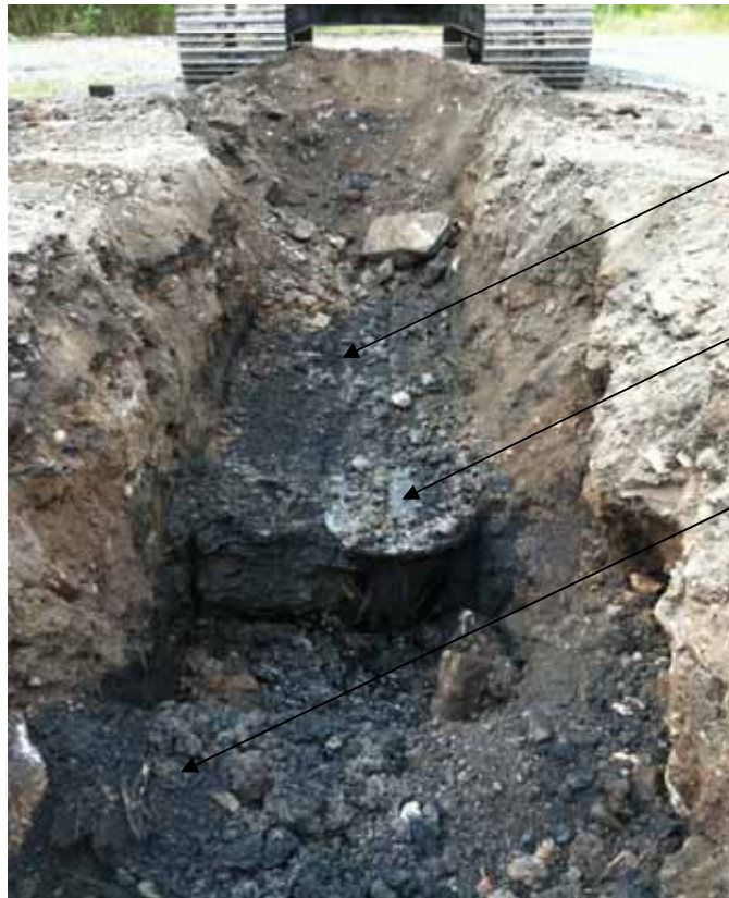
Photo #8 (2011.09.14): CTP-6. Looking east to west from top of gas holder #2. 8" vertical pipe observed 3' below groundwater surface.
