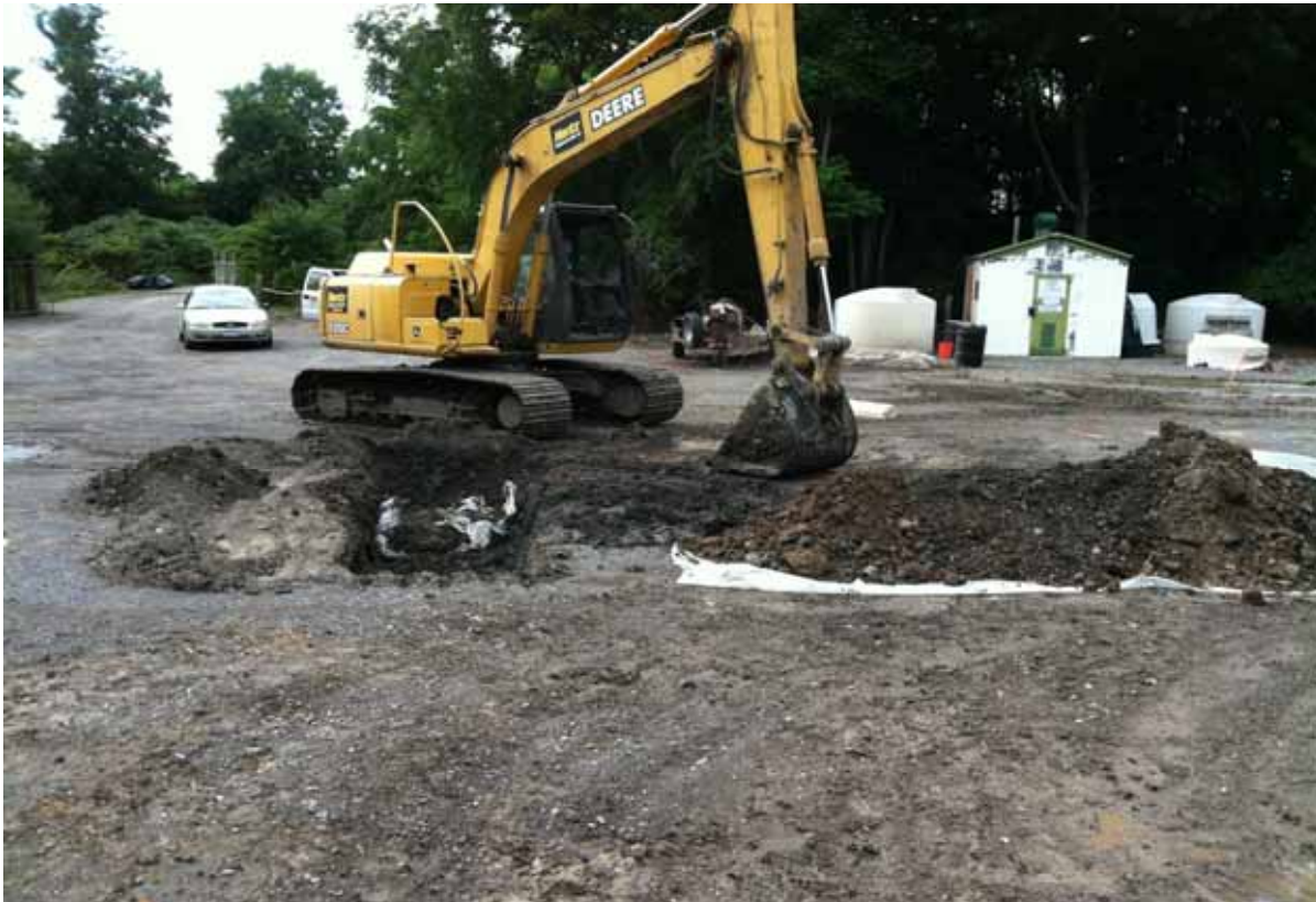
Photo #12 (2011.09.16): CTP-9. Looking south. Excavator completing test pit.
