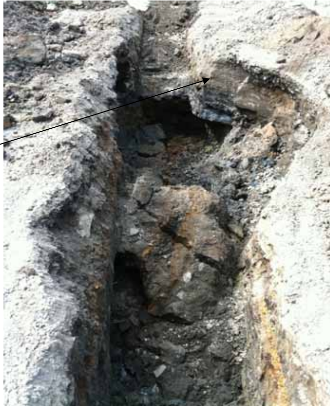
Photo #11 (2011.09.14): CTP-7. Looking east to west at start of test pit at east side of gas holder.
