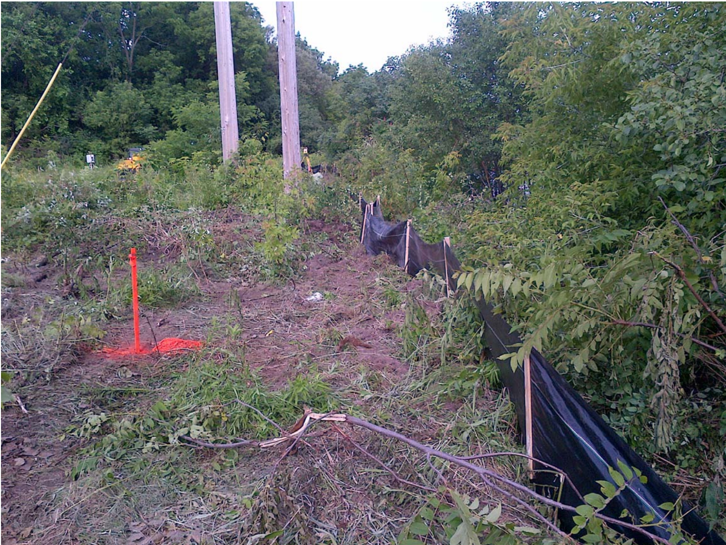
Siltation fence beginning install – northern edge of site near Owasco Outlet
