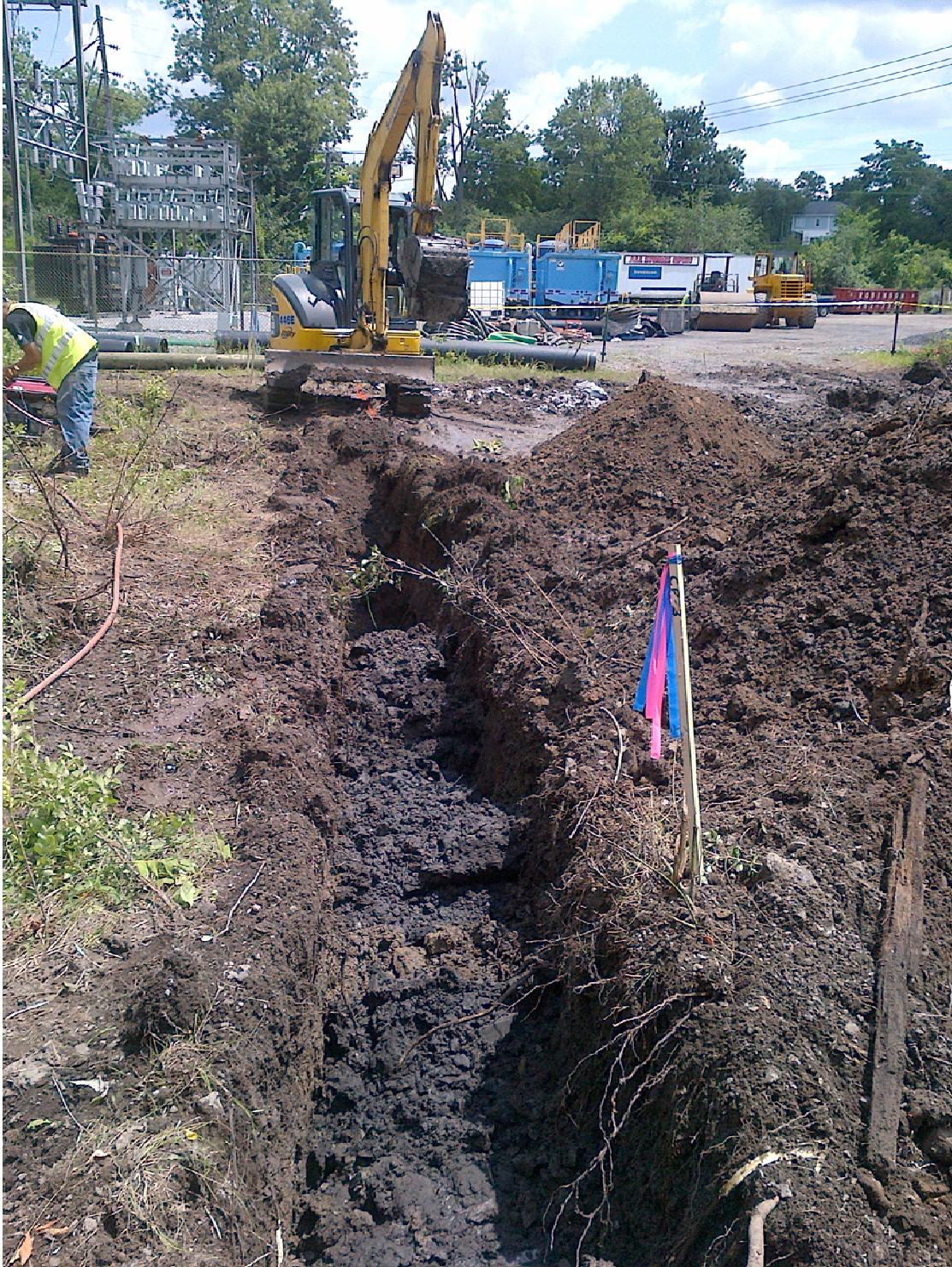
Northern leg of ISS wall facing east
