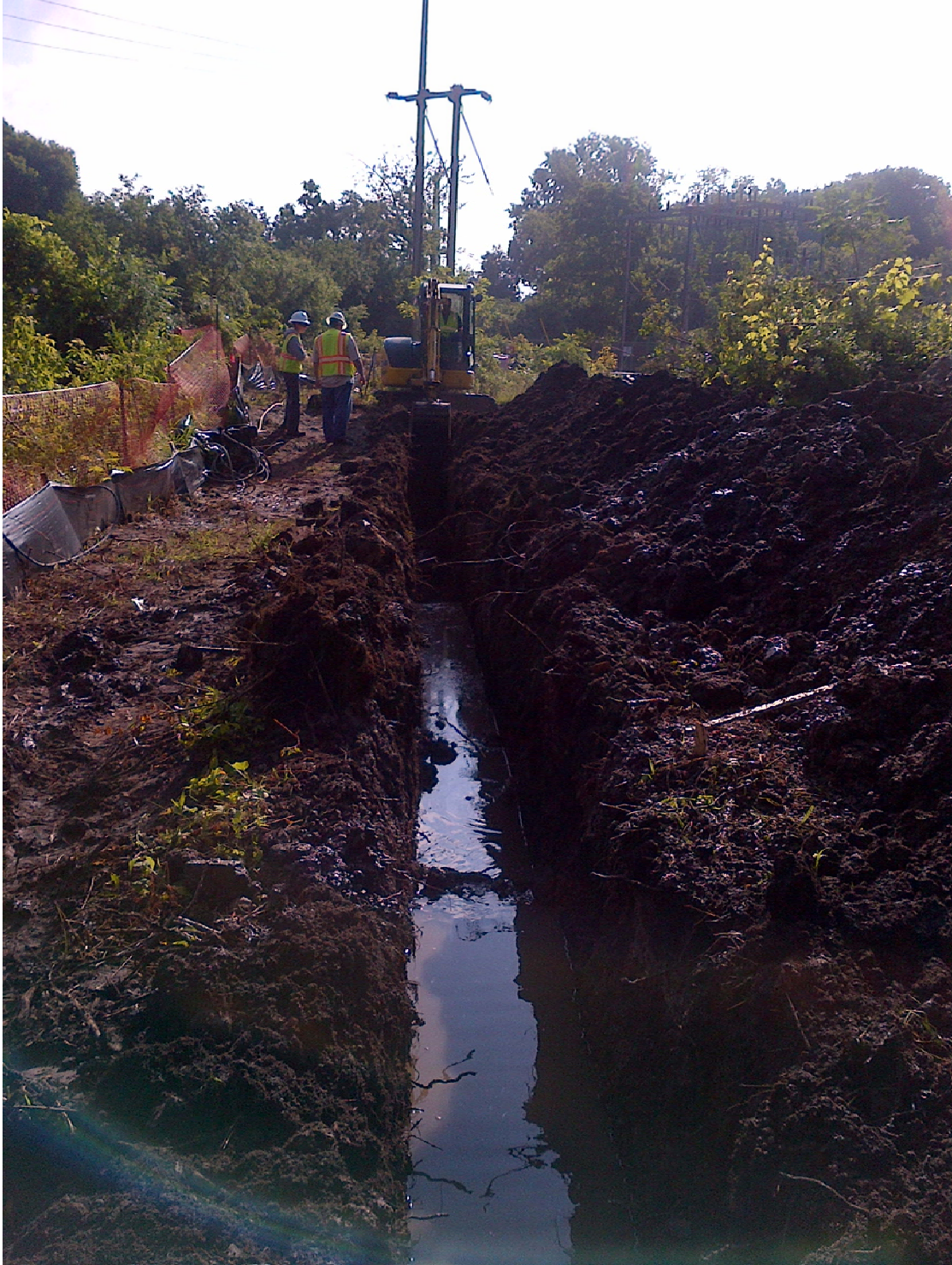
Western leg of ISS wall facing north
