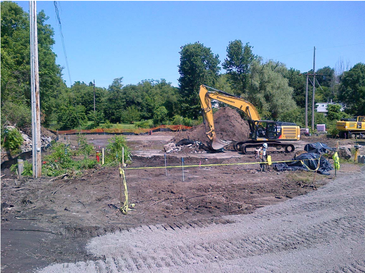
Potential reuse soil stockpiled atop concrete holder floor
