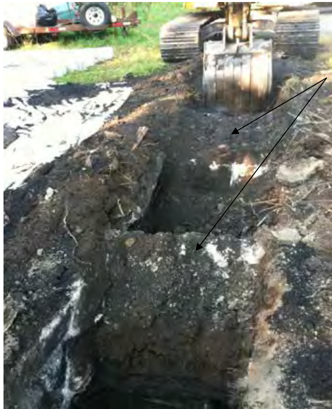
Photo #12 (2010.09.13): MTP-3A. Concrete structures found at west end of test pit (0.5' – 1' bgs).
