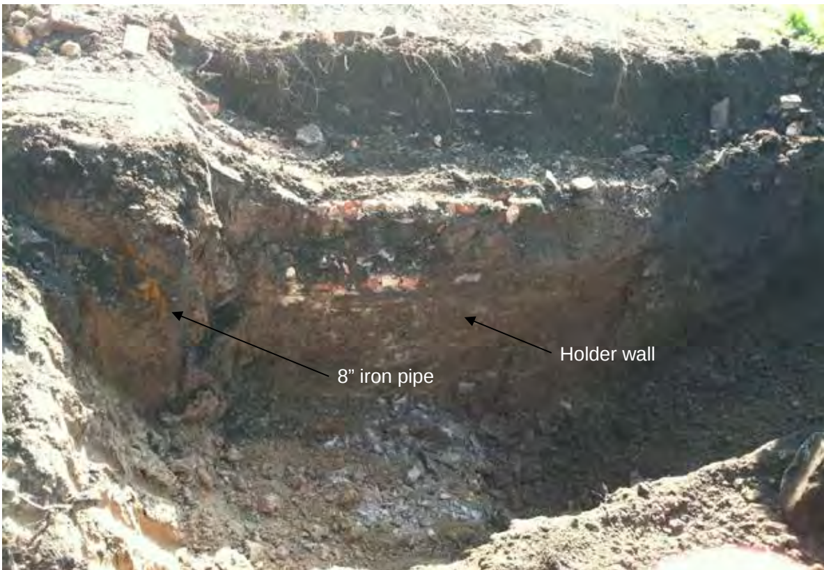
Photo #6 (2010.09.12):MTP-1C. Vertical 8" pipe located from 1.5 to 5' bgs.
