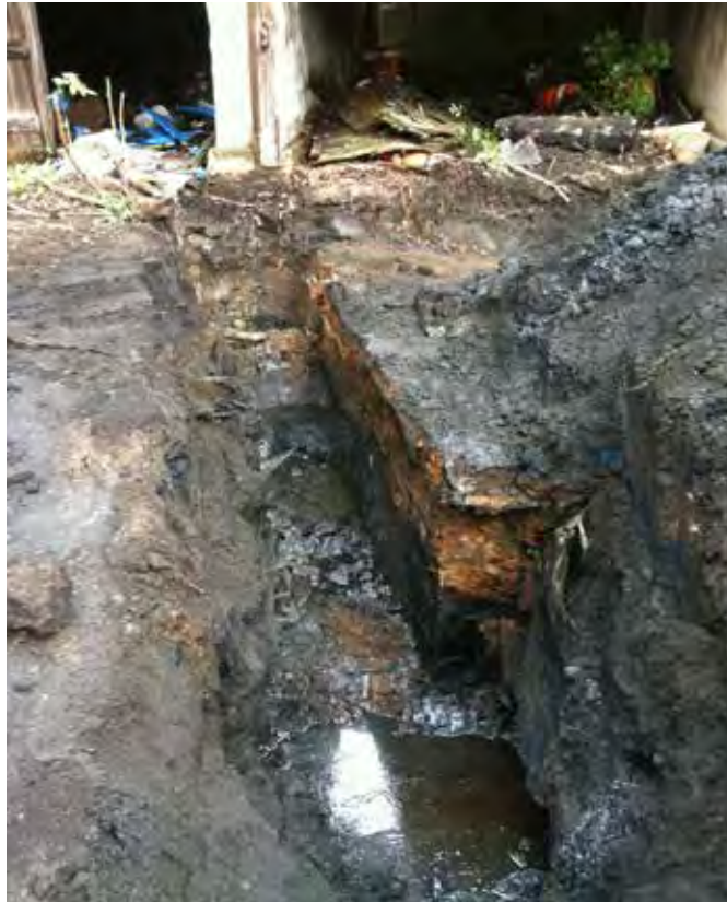
Photo #13 (2010.09.08): MTP-3A. Basement/foundation at east end of test pit.
