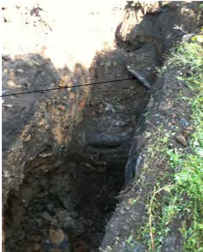
Photo #4 (2010.09.12): MTP-1B. 4" PVC pipe approximately at north end of test pit.
