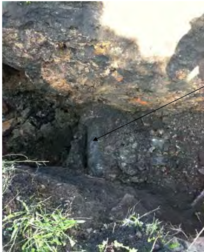
Photo #3 (2010.09.12): MTP-1B. Looking down at 8" black iron pipe.
