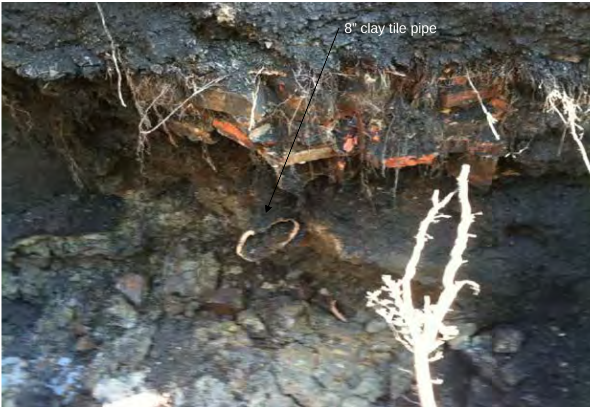
Photo #11 (2010.09.13): MTP-3A. Red brick structure atop wood structure, 8" clay tile pipe just below.
