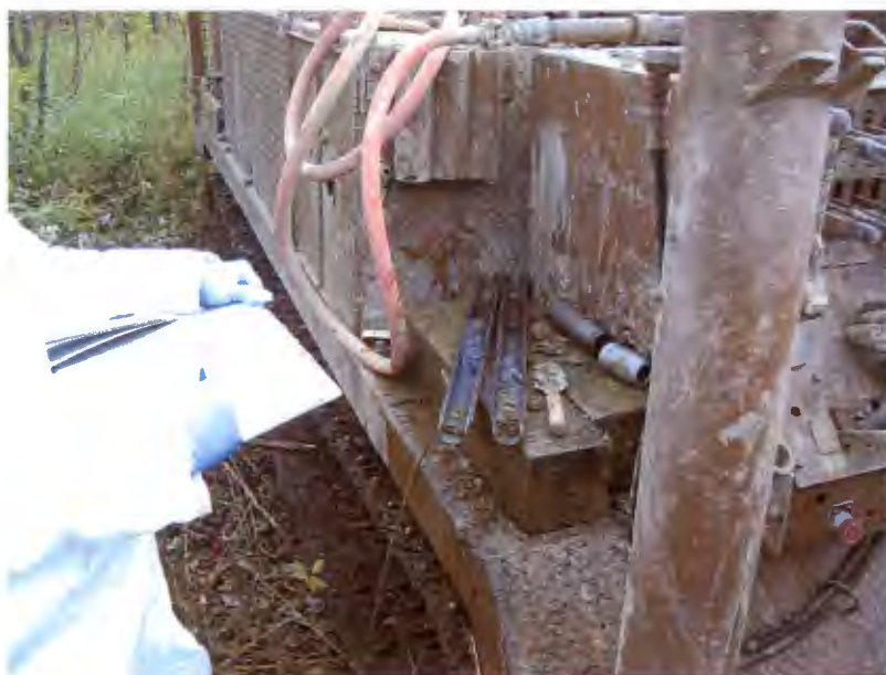
Photograph 3. Soil boring sample MDA-TB5 (4 to 6 ft) collected from sludge disposal area.
