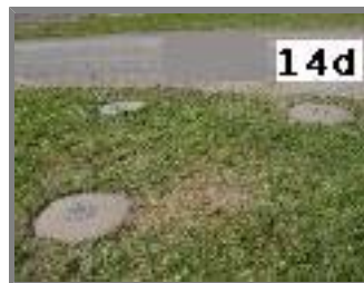
(Left) TW-14d, new roadbox and collar just emplaced on 10/4/2007. TW-14d is the well on the right in the above photo.
