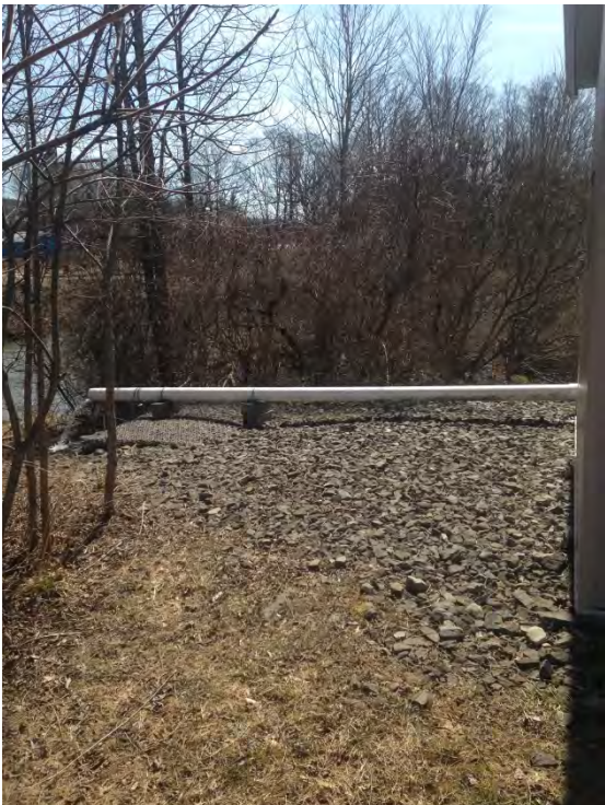
Effluent Outfall to Otselic River
