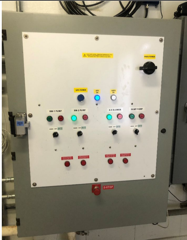
View of Treatment System HOA panel door.
