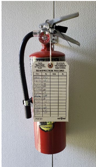
Fire Extinguisher with inspection record.
