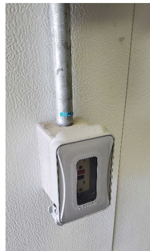
Ground-fault circuit interrupter (GFCI) outlet.
