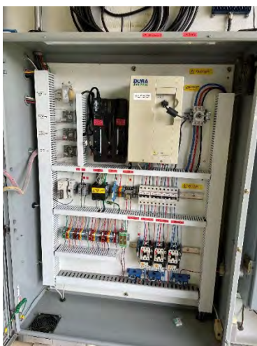
Interior view of MCP.
