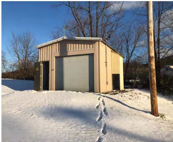
Front exterior view of treatment system building.
