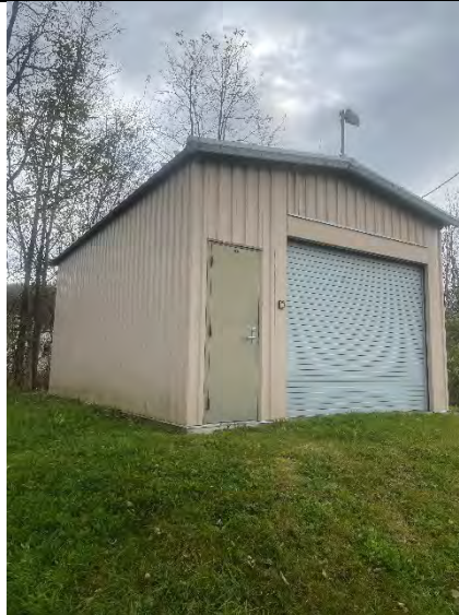
Exterior view of treatment system building.
