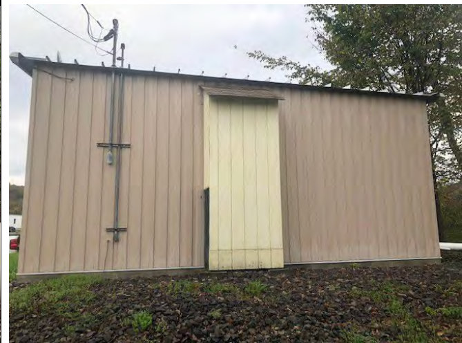
Exterior view of treatment system building.
